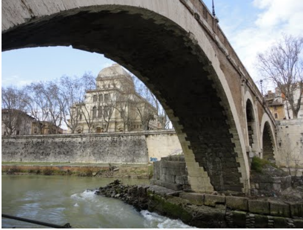
Figure 1 – Fabricio bridge, Rome - Italy
