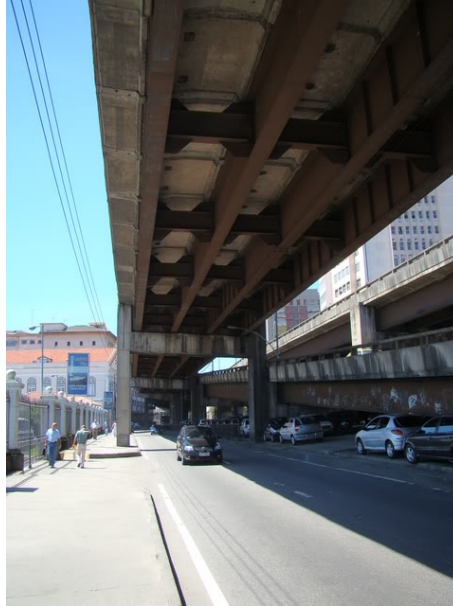
Figure 3 – Perimetral viaduct, Rio de Janeiro - Brazil
