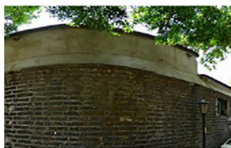
FP Error Type 1: failing to identify an unattractive wall which blocks the sight
