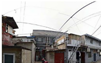
FN Error Type 1: failing to identify dilapidated buildings as a building
