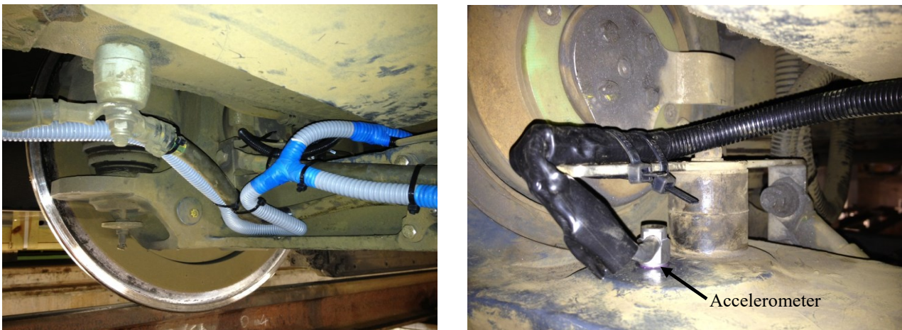
Figure 6: Accelerometer cabling (left) and location (right) on the axle bridge of the trailer bogie
