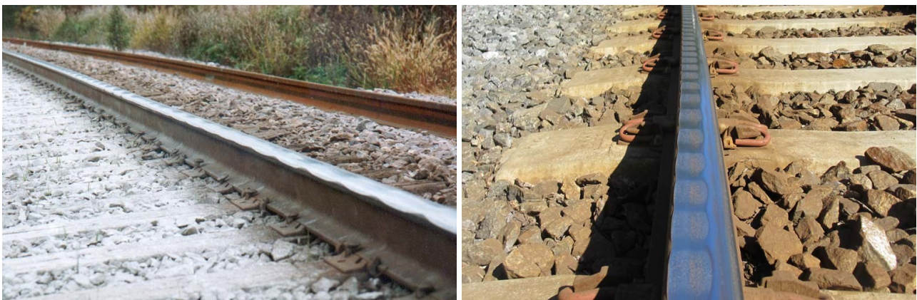
Figure 1: Examples of rail corrugation on mainline track (Images: RailMeasurement Ltd. Used with permission)
