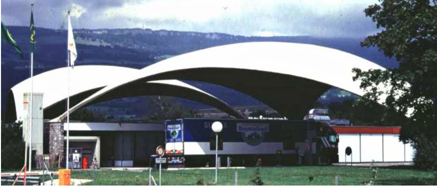
Fig. 8 The 31.6 m span shells for Deitingen Süd Petrol Station (1968) (Photo: John Chilton)
