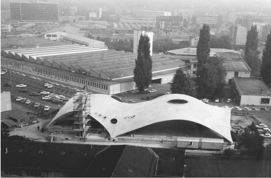
Fig. 10 Sici SA Factory shell, Geneva (© gta archives/ETH Zurich (Holding Heinz Isler), Photo: Chu-Chun Chuang)
