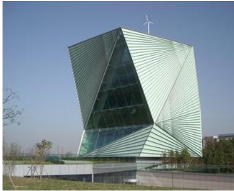
Figure 5: The CSET building
