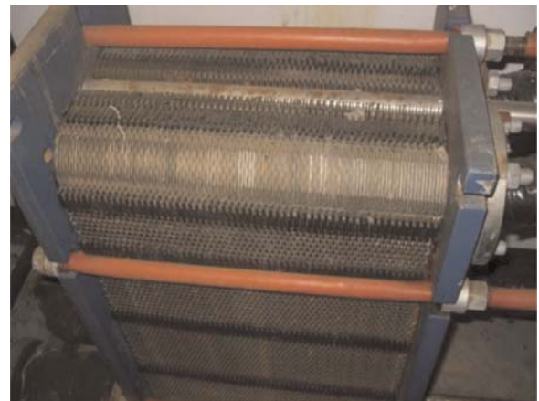
Figure 4. Flat-plate heat exchanger.
