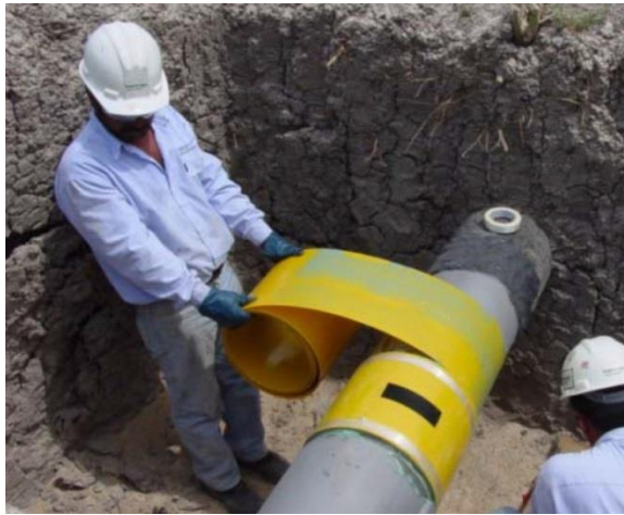
Figure 2-5, Installation of Clock Spring® on a steel pipe (Clock Spring, 2012)
