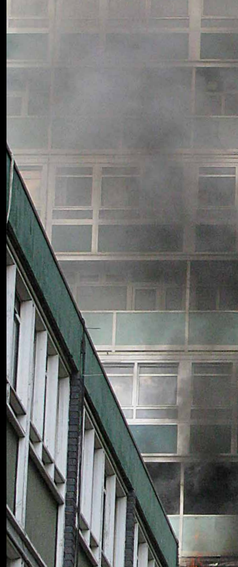
Above: The fire at Lakanal House in South London that killed six people in 2009 – recommendations from the coroner’s report were still under review by government when many more died in Grenfell Tower
