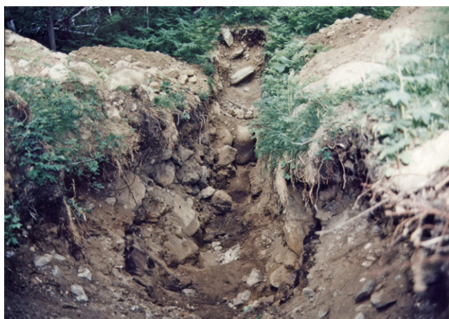
Fig. 8. Trench A-2, viewed from the side of the basin.
