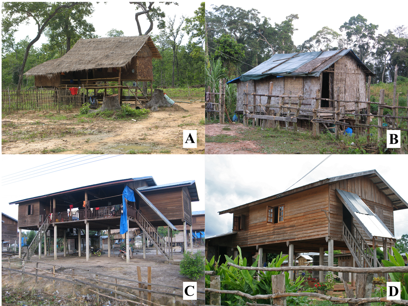
Figure 2. Typical resettlement and traditional houses in the study area. Traditional houses (A and B) are normally constructed from bamboo thatch with roofs made from thatch, wooden tiles or corrugated iron. Doors and windows are poorly fitting and there are many gaps in the walls and floors. Traditional houses are raised on stilts on average 1.27 m above the ground. Resettlement houses in contrast (C and D) are built from pre-dried hard wood with corrugated iron roofs. They generally have fewer gaps in the walls and floors than a traditional house and have well-fitting doors and windows. They are raised on stilts an average of 2.66 m above the ground. The houses shown in this figure are for illustrative purposes and may not have been sampled during the study. doi:10.1371/journal.pone.0062769.g002
