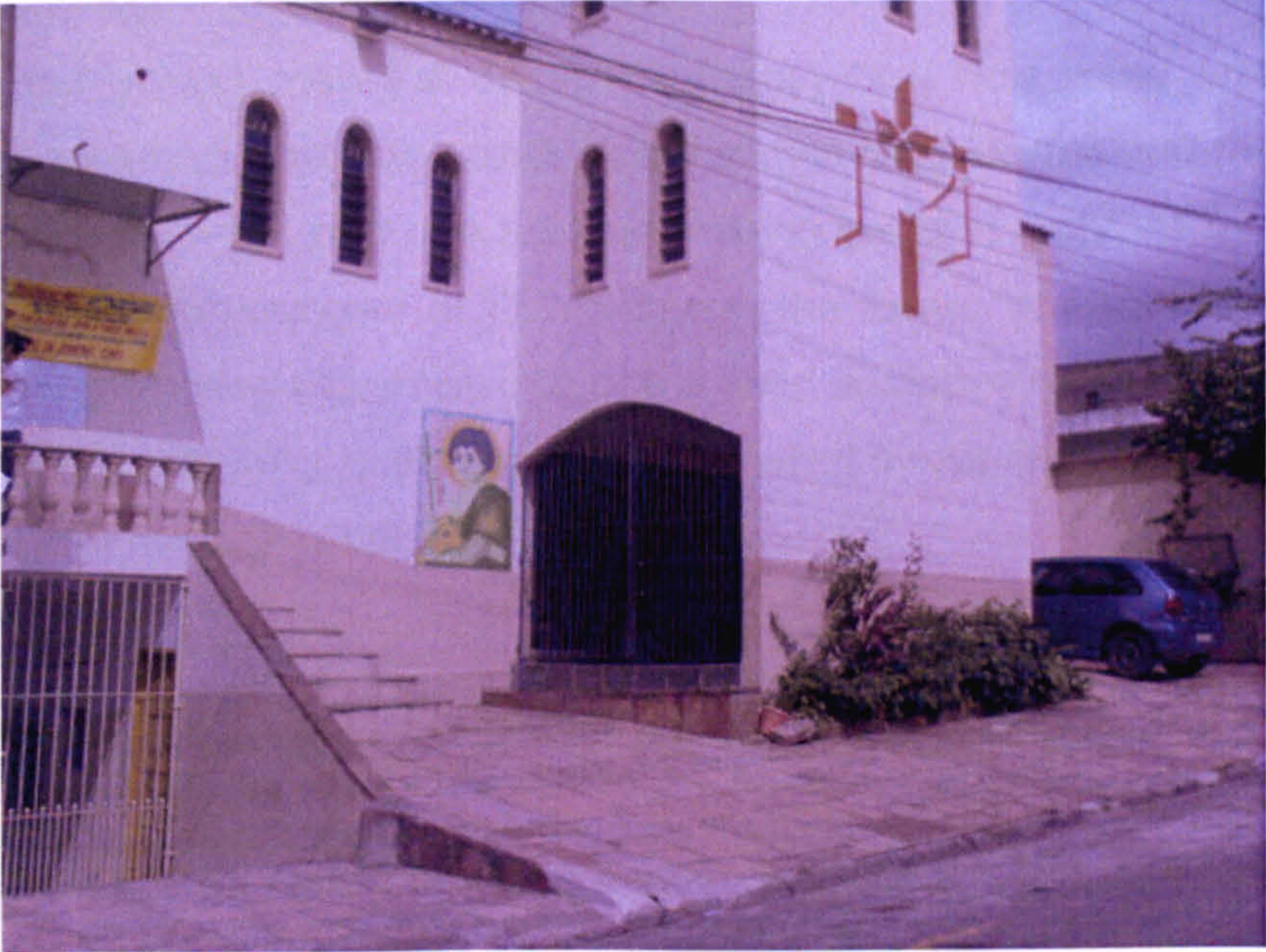
Figure 6 The RAC Building from the front
