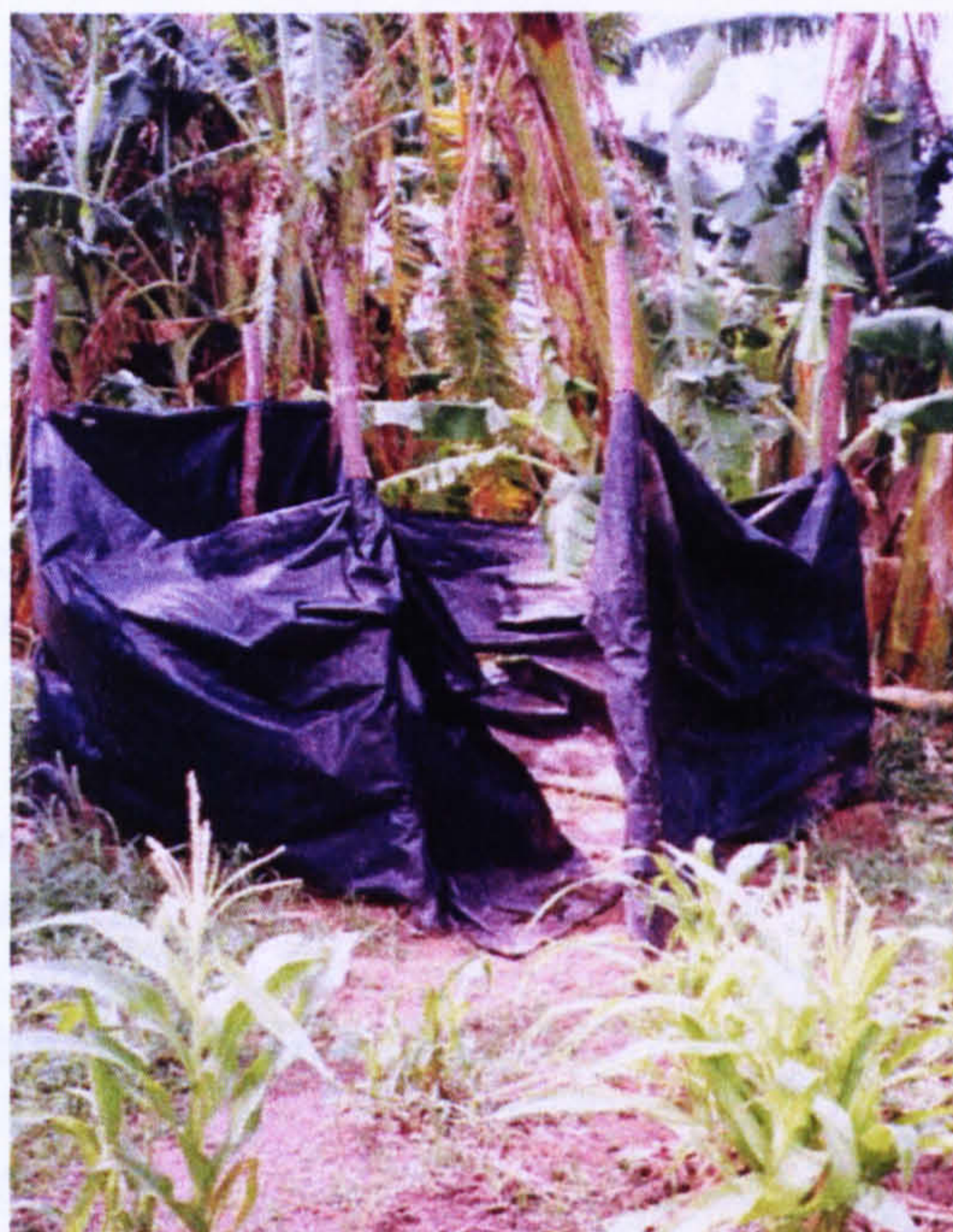
Figure 7-1: Typical latrine superstructure
