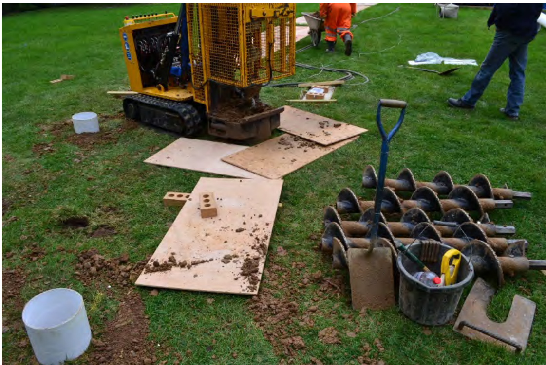
Figure 5-6: Site trial pile installation.
