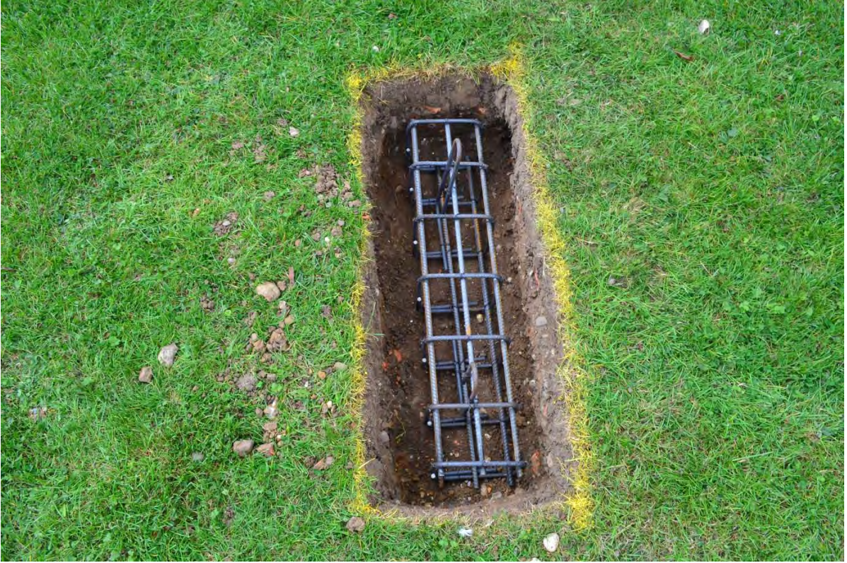
Figure G-5: Rebar cage in excavation
