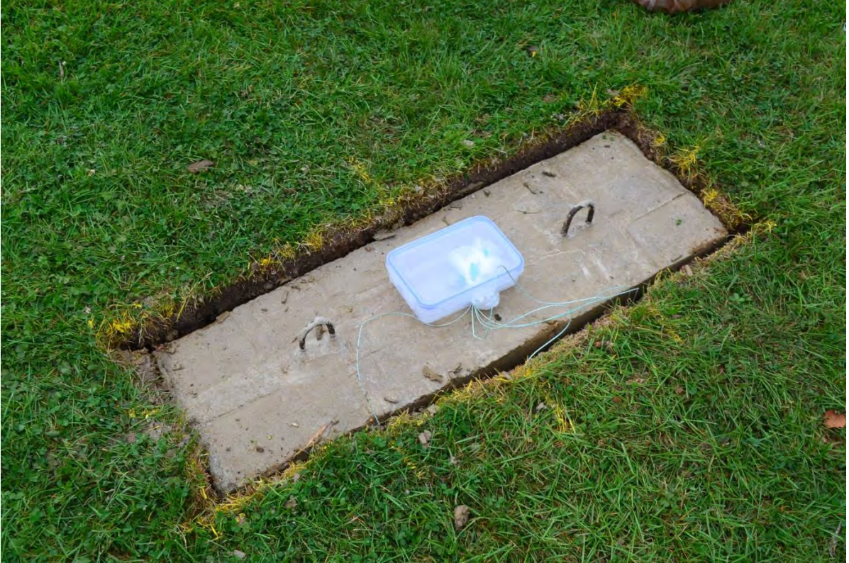
Figure G-9: Concrete footing in place
