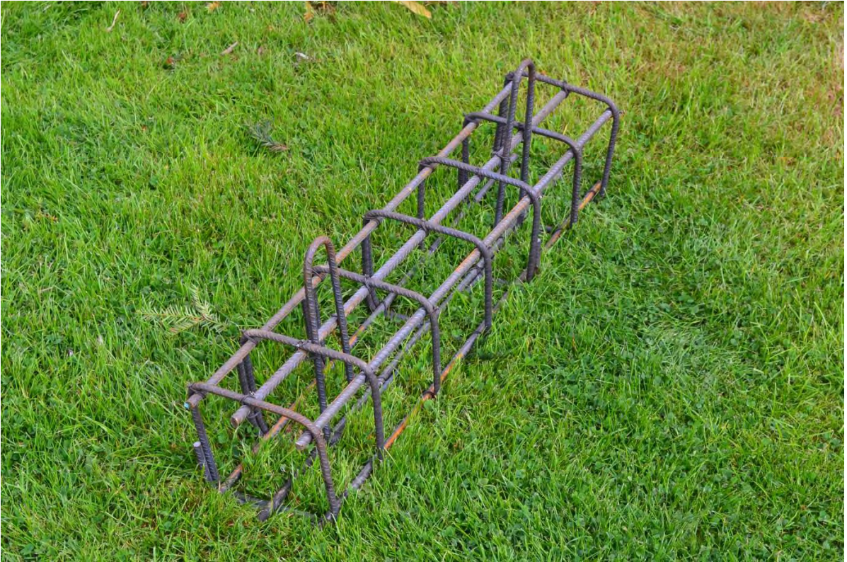
Figure G-6: Rebar cage
