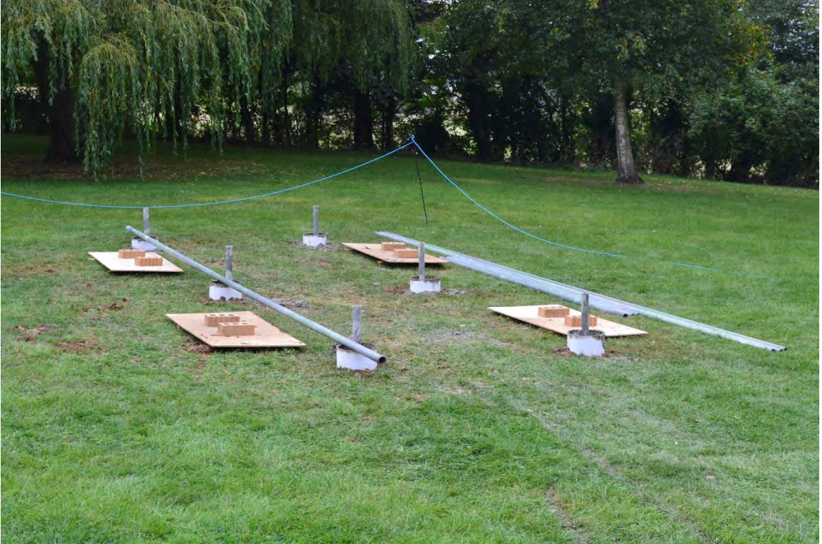
Figure G-12: Completed piles
