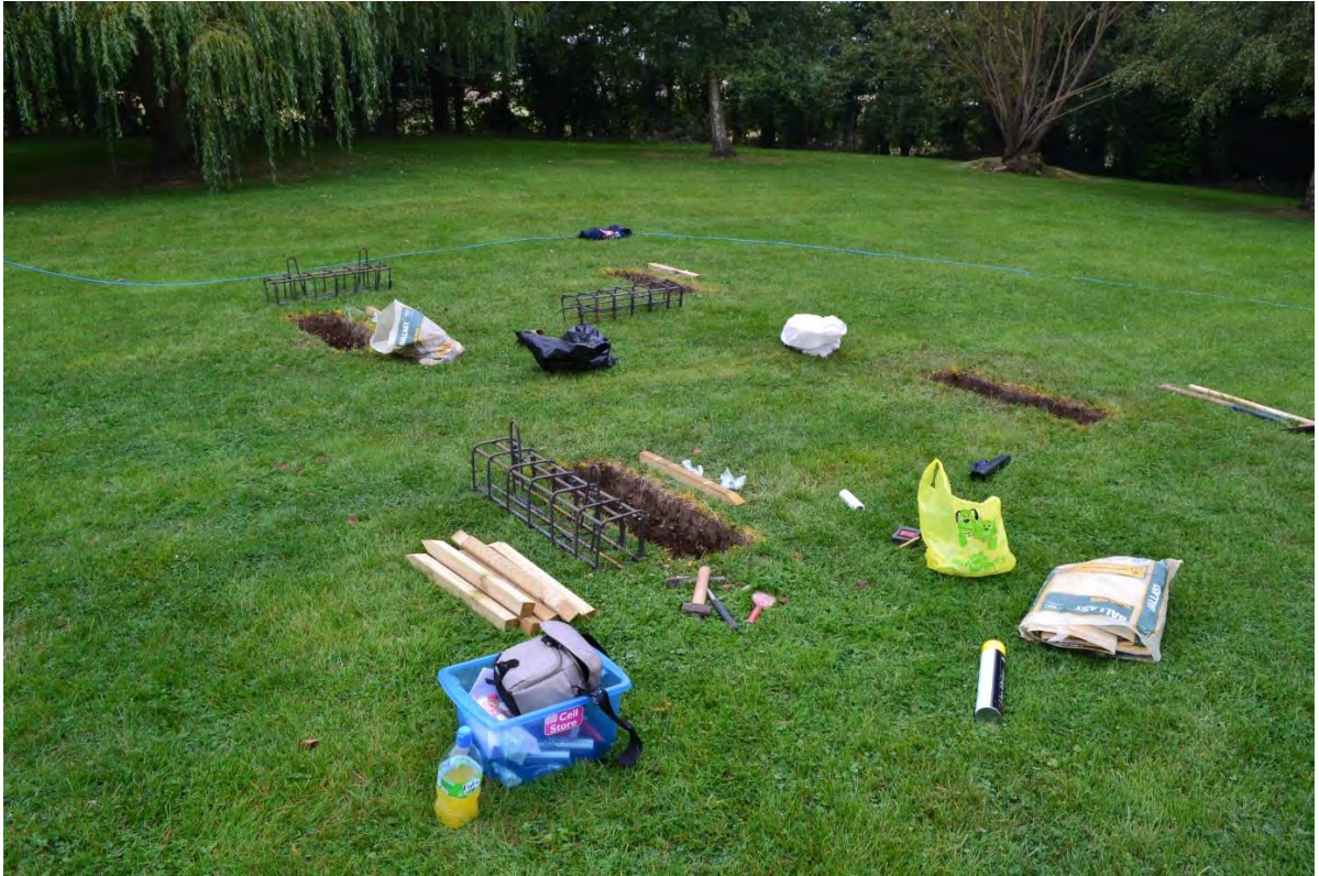
Figure G-7: Excavations and cages
