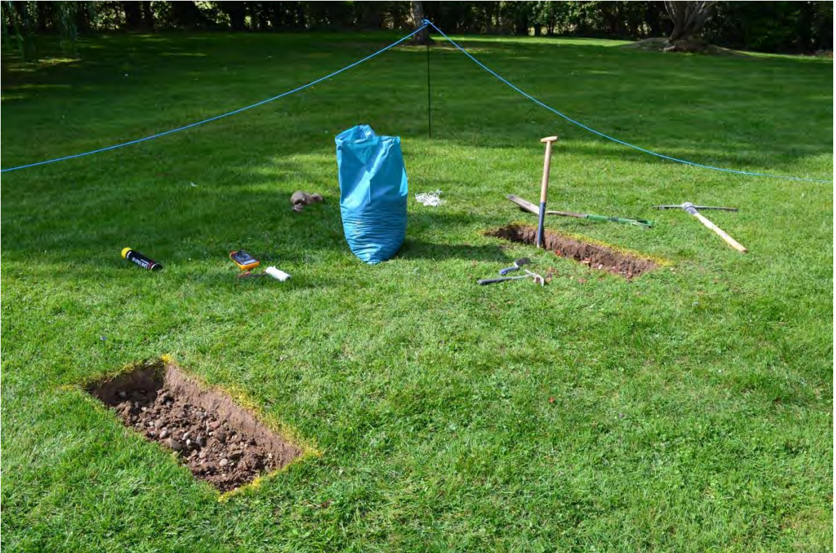
Figure G-4: Footing excavations
