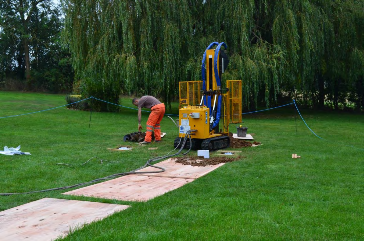
Figure G-10: Piling
