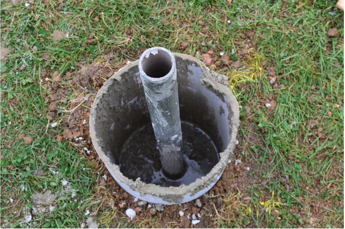
Figure G-13: Completed pile with scaffold reinforcement
