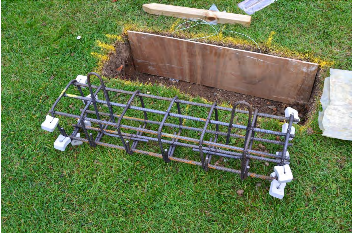
Figure G-8: Rebar cage with spacers
