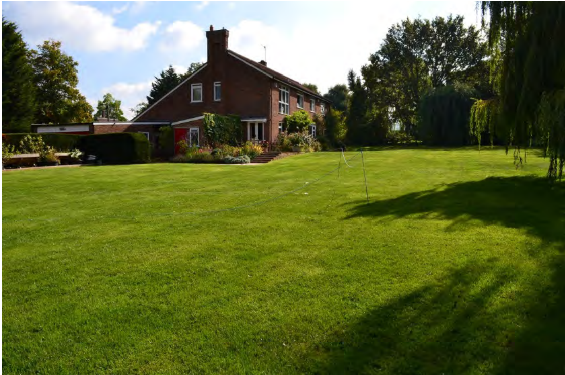
Figure 5-1: Site trial area with nearby subsidence affected house.
