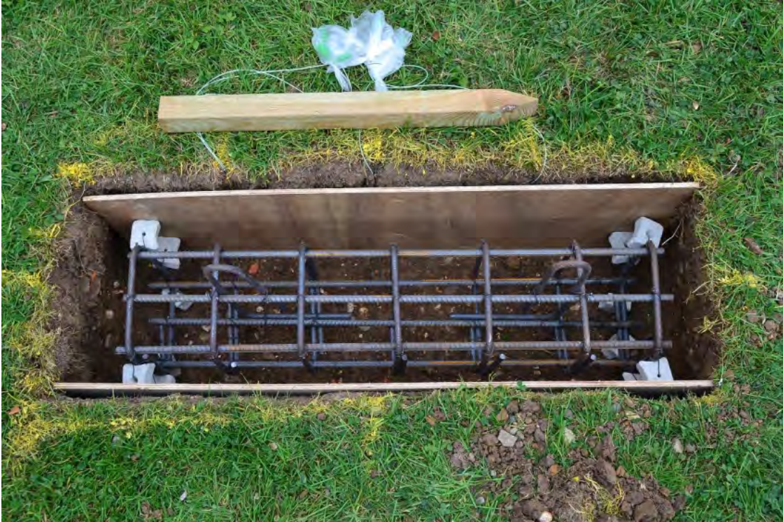
Figure 5-18: Site trial footing reinforcement and shuttering before concrete pouring.
