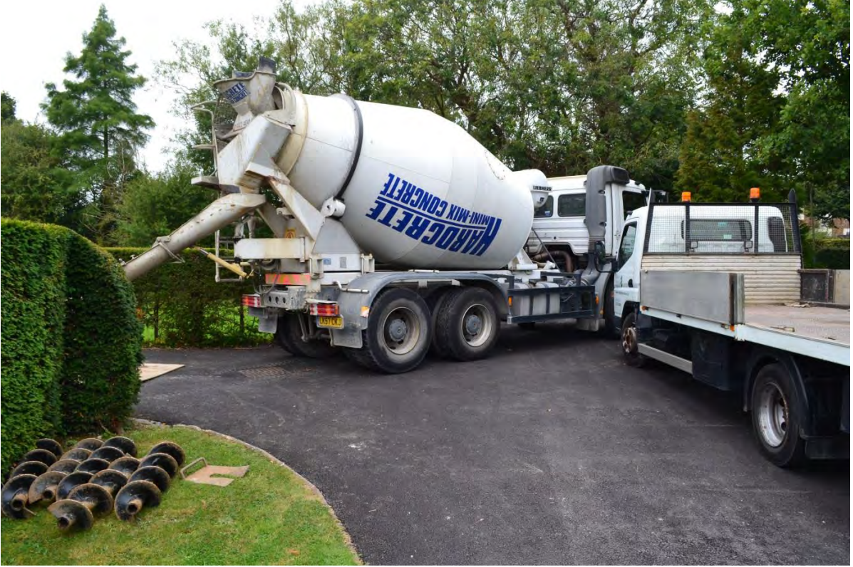
Figure G-11: Concrete wagon
