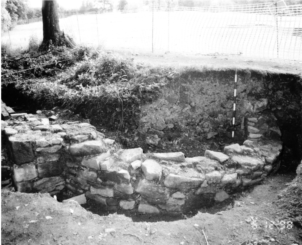
Fig. 5.1: Shenstone's use of sandstone rubble coursing observed in the curved Ruined Priory wall. 642
