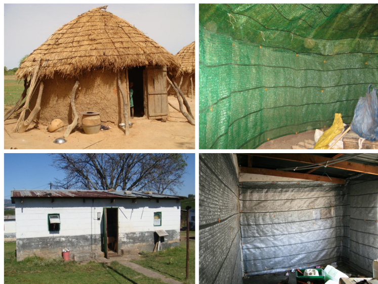
Figure 3 Durable linings (right) installed in traditional houses in rural Mali (top left) and South Africa (bottom left).
