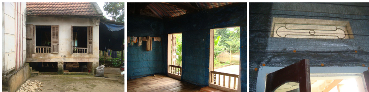
Figure 4 Durable lining installed in bedrooms (middle) or sitting rooms (right) in traditional houses in rural Vietnam (left).
