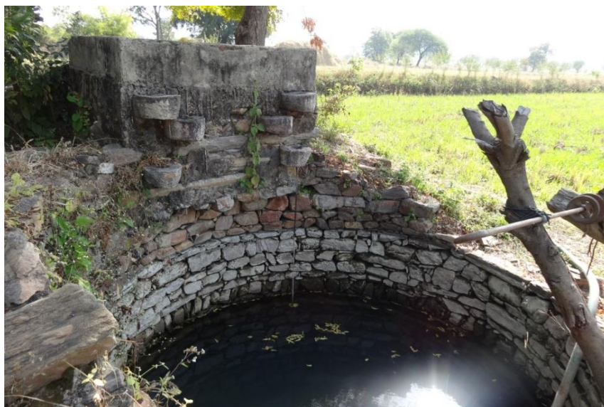
Figure 8-13. Site 162: Round brick and stone well with a parapet, located in agricultural fields.
