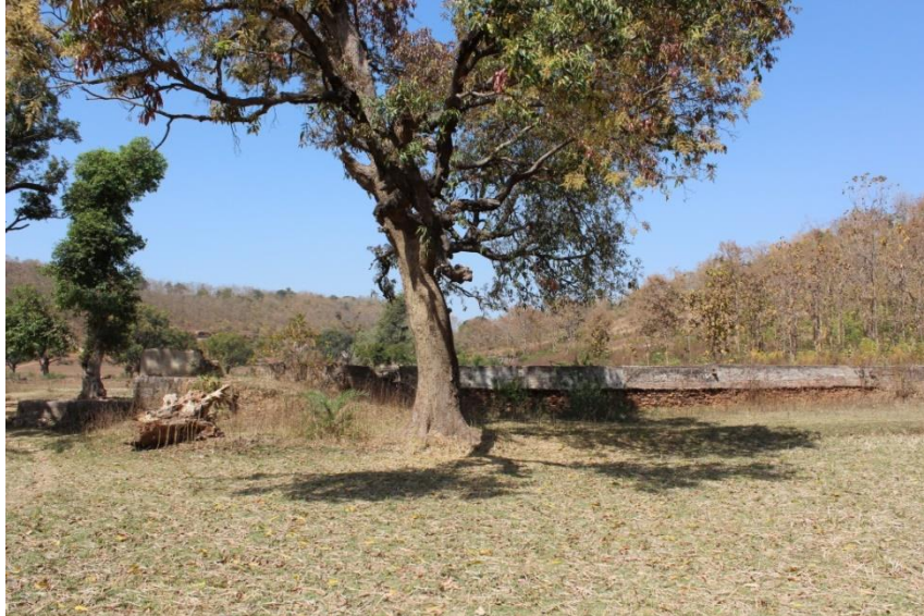
Figure 8-15. View of brick and stone bāvlī to the east of Ambālā tank. In the left hand side of the picture the long, underground arched bāvlī terminates in a round brick and stone well with a parapet.
