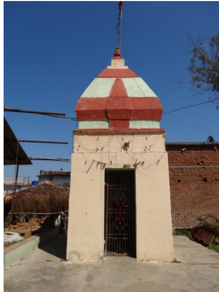
Figure 9-30. South facing Hanuman temple with modern exterior in Nagardhan (site 62).
