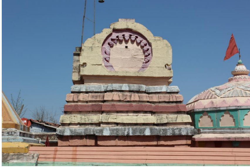
Figure 3-14. Vaulted roof of the Kālikā Devi temple in Rāmṭek town.
