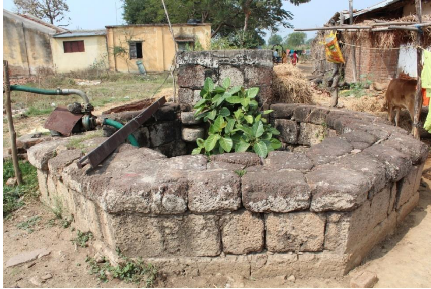
Figure 8-12. Site 307: Stone well in Bori village with octagonal casing and hooped stones on a parapet for a pulley system.
