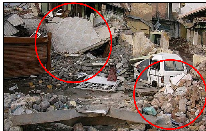
Figure 5.11 A pukka building in urban Bagh, mixed construction material (stones and bricks) is used in the same wall (picture above); destroyed pukka construction in urban Muzaffarabad, mixed construction material such as bricks and concrete blocks can be noticed in red circles (picture below). (Source: SERRA)
