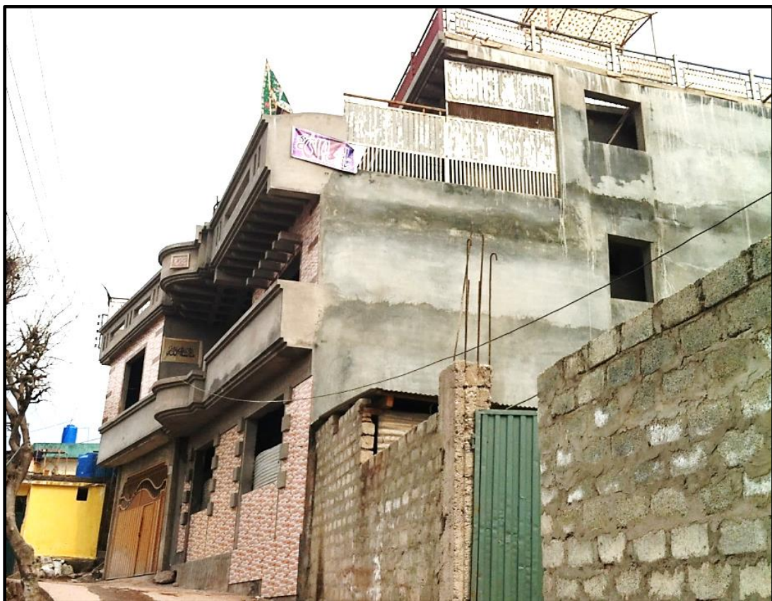
Figure 7.10 A three storey heavy pukka house in Red Zone, where only a lightweight single storey structure should have been constructed. (Source: Author (fieldwork))
