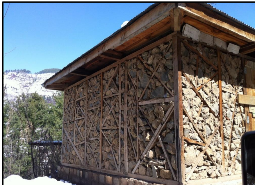
Figure 5.6 A Dhajji-dewari building in rural Muzaffarabad. (Source: Author fieldwork)
