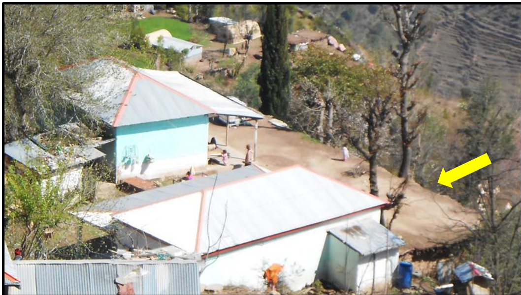
Figure 5.3 A Pukka house in rural area with a kacha cattle shed or gohaal (yellow arrow) added with the house which serves as courtyard as well; notice shear fall in front of the cattle shed. (Source: Author fieldwork)
