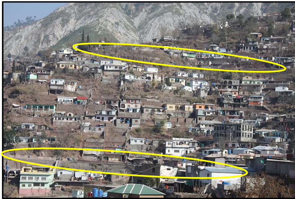
Figure 5.18 Massive building and road construction (yellow circles) on steep slopes in Muzaffarabad city. All the construction has been done after doing earth cutting.
