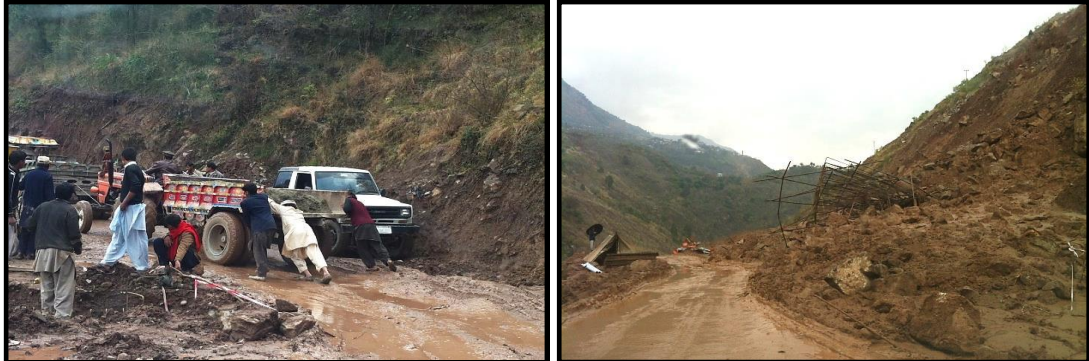
Figure 9.2 Landslide hazard on the roads.
