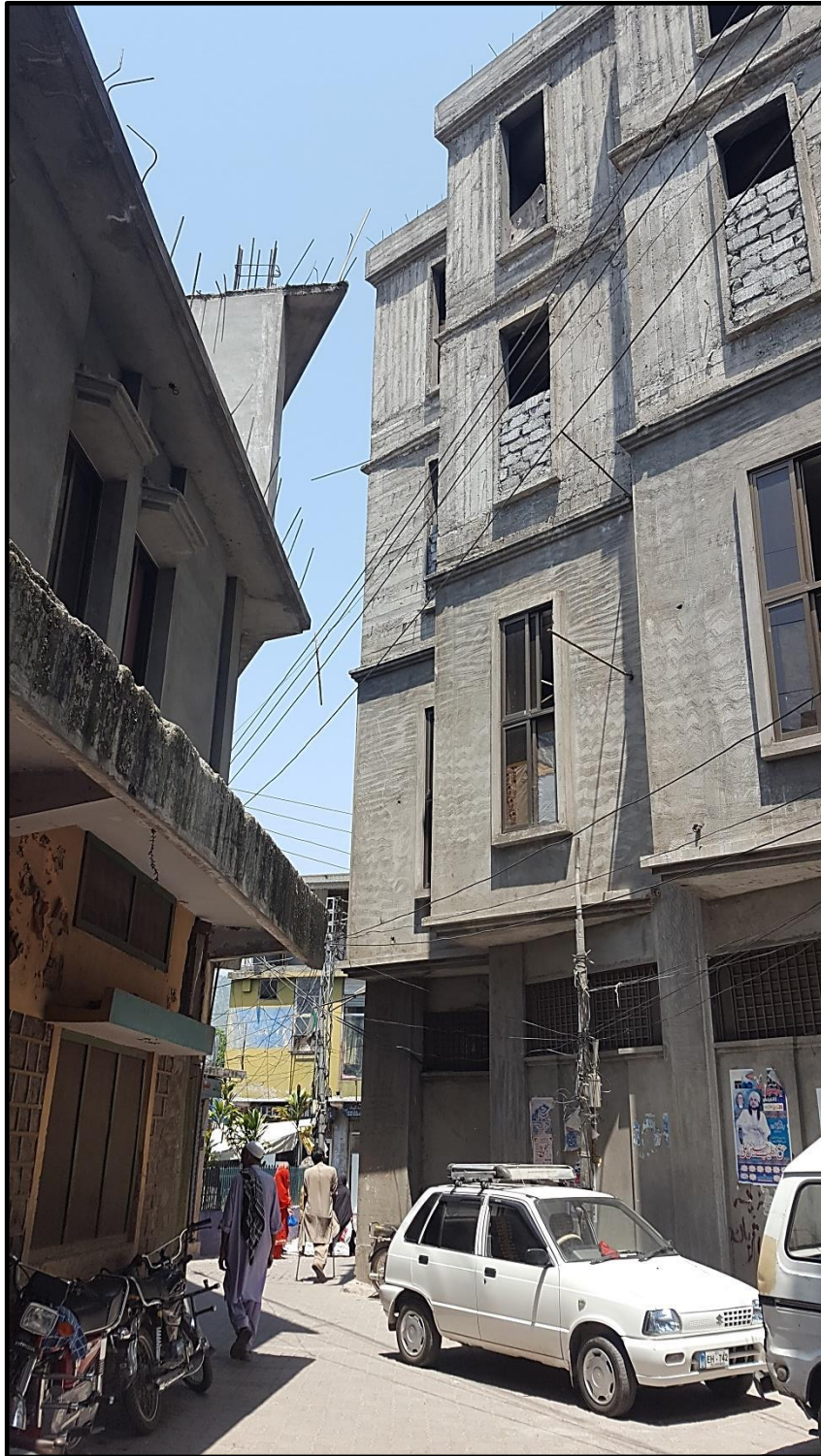
Figure 7.14: Newly constructed multi-storey buildings in the congested old city area of Muzaffarabad. Notice narrow street and addition of new storeys on an old dilapidated building on the left. (Source: Author fieldwork)
