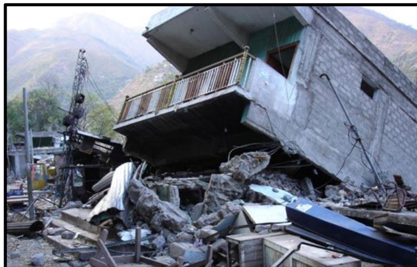
Figure 5.12 A Destroyed Pakka House
