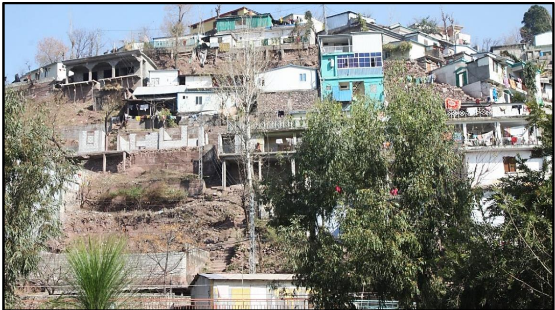
Figure 7.11 Construction on steep slopes in Muzaffarabad city; these houses have been built by cutting the hill. Almost half the house is on ground and half of stone pedestal or concrete pillars which seriously compromises the safety of the structure.
