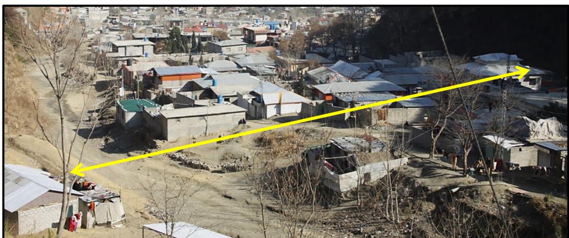
Figure 7.13 Construction in the Gojra Nullah; the yellow arrow shows the width of the nullah that has been taken over by illegal houses. (Source: Author fieldwork)
