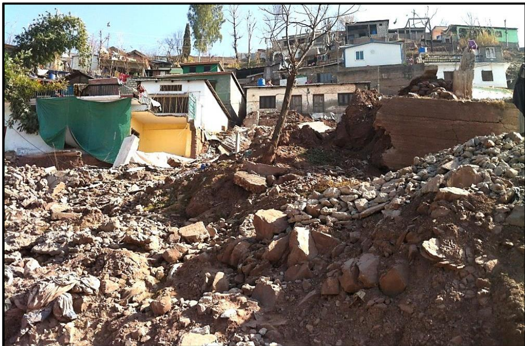
Figure 7.18 Houses facing grave danger due to landslide. People are still living in these houses. (Source: Author (fieldwork))
