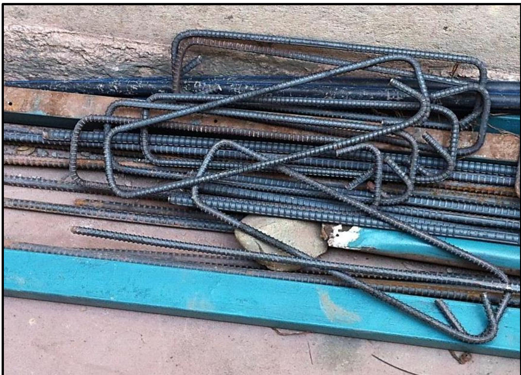
Figure 7.3 Properly formed steel rings for RCC frame structure, a rarity before the earthquake. (Source: Author fieldwork)
