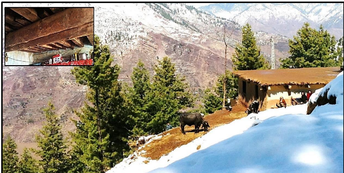
Figure 5.1 A rural kacha house in Salmia (Muzaffarabad), flat mud roof (saturated with water) and steep slope can be noticed (inset: whole tree trunks as roof beams).
