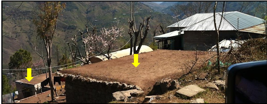
Figure 7.9 Kutcha structures (yellow arrows) added with reconstructed pukka house in rural Muzaffarabad. (Source: Author fieldwork)
