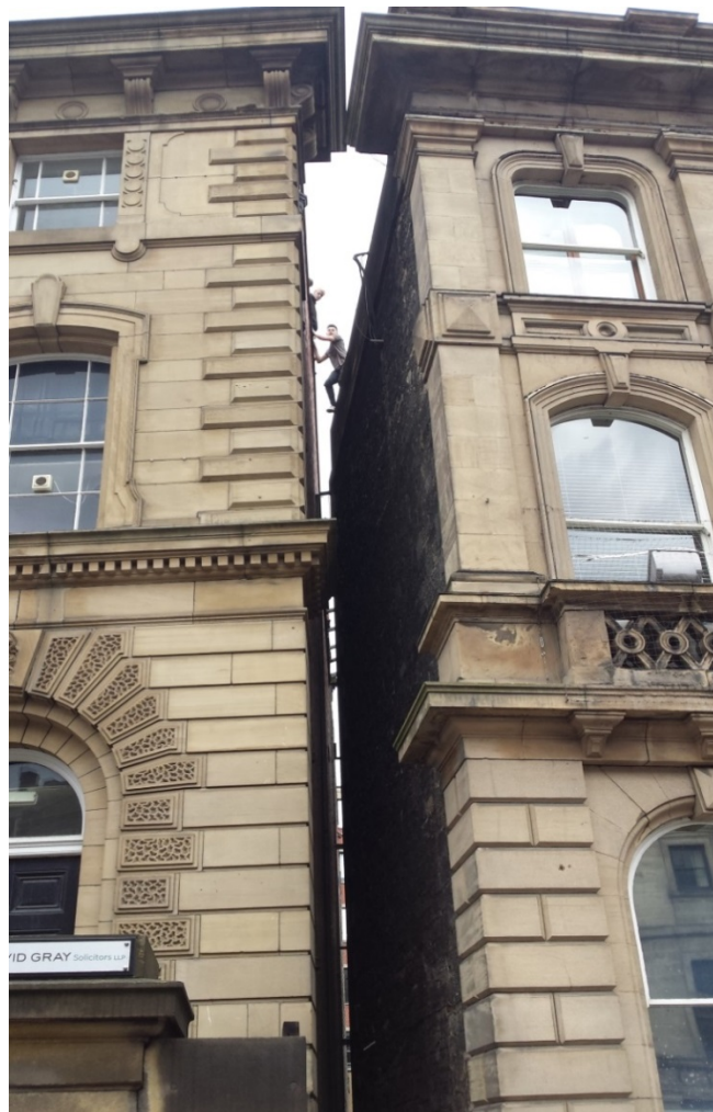
Roof mission: Out of sight on one of the busiest streets in Newcastle. March 2015
