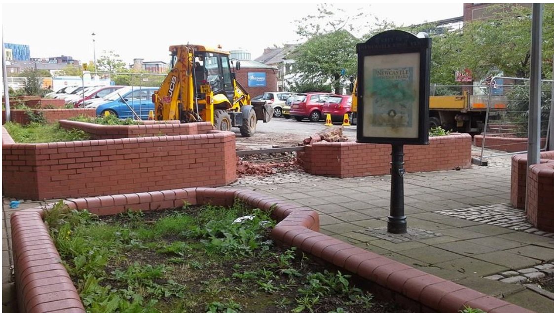
The ‘double kong’ wall is the first to go down. September, 2014
