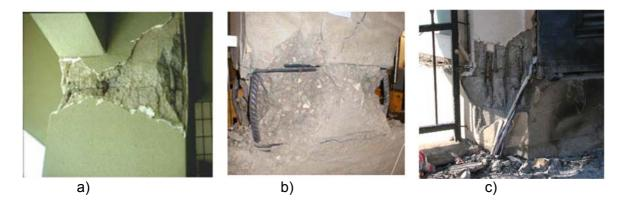
Figure 9: Examples of indicators observed during post-earthquake inspection: a) cracking of concrete, b) buckling of reinforcement, and c) anchorage pull-out (Fardis et al. 2008, Yazgan et al. 2012)
