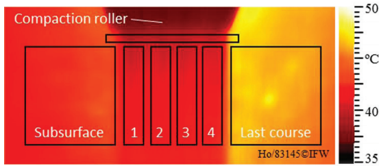
Fig. 1. Thermal process image within the ROI.
