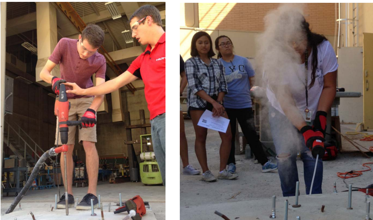
Figure 7: Activity was assisted by Hilti and tested the placement and pullout strength of concrete anchor bolts.
