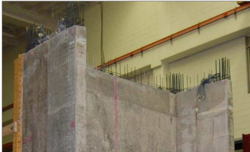
Figure 2.9: Wall 6 after formwork removal
