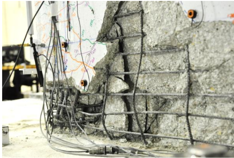
Figure 9.6: East flange damage attributed to out-of-plane movement in Wall 8
