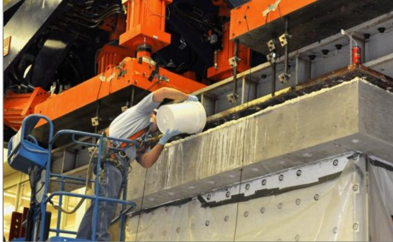
Figure 4.3: Pouring Hydrocal for connection of Wall 7
