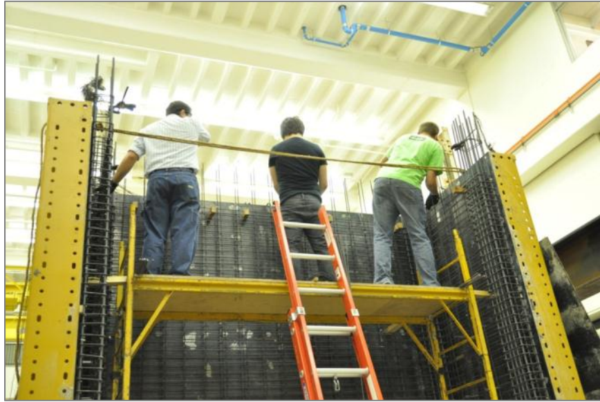
Figure 2.6: Near completion of Wall 8 rebar cage
