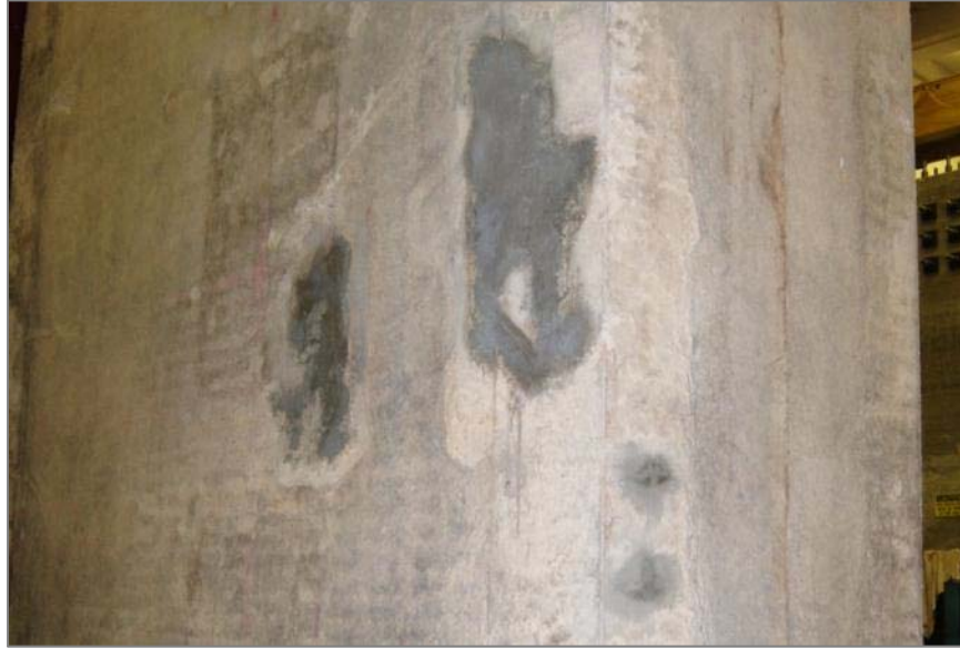
Figure 2.10: Wall 7 after patchwork near mid-height of web
