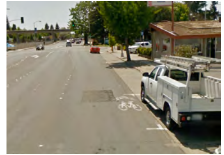
Figure 6.4 — Class III bike lane on A Street (Google Earth, 2011)
