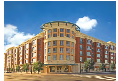
Figure 3.2 — Example of High Density Residential
