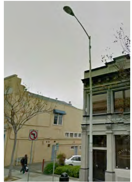
Figure 6.14 — Existing street light fixtures
