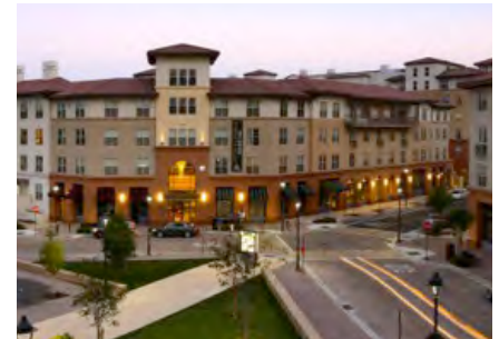
Figure 5.26 — Example of a BART Transit-Oriented Development, the Pleasant Hill BART development (MVE & Partners)
