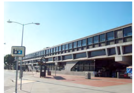
Figure 6.5 — AC Transit bus stop outside of the Hayward BART station
