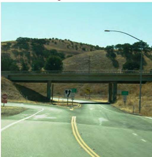
Figure 6-6: Existing interchange on 10th St.
