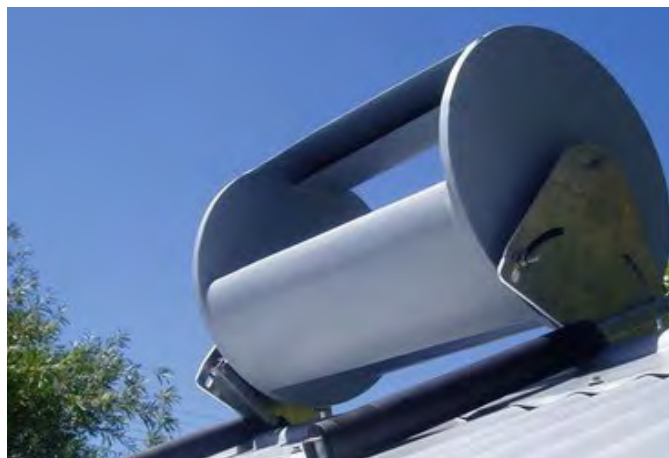
Figure 5-15: Roof top wind generator
