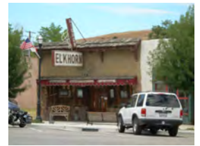
Figure 9-28: Elkhorn Bar on Mission Street
