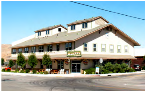
Figure 9-3: Mission Market and Deli, a main downtown business. An example of the newer commercial buildings in the Downtown Core.
