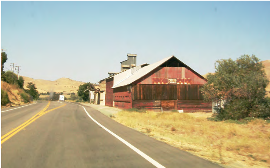
Figure 9-32: Existing commercial service building
