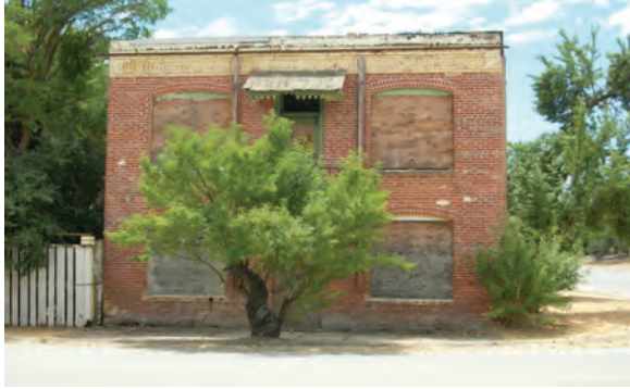
Figure 1-11: Historic Sims Hotel Source: Cal Poly Consulting Team
