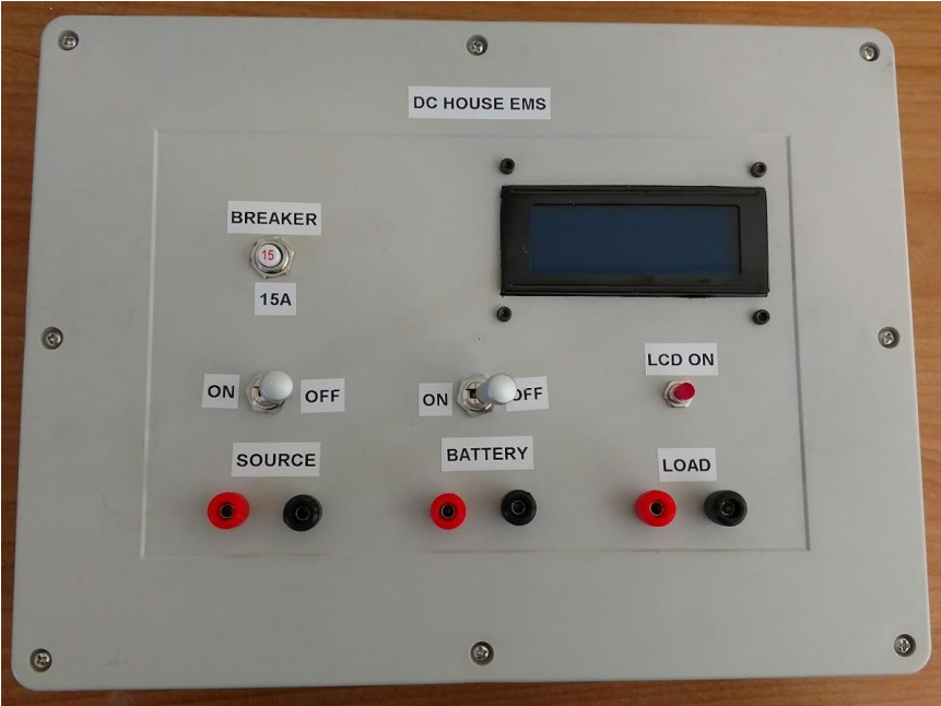
Figure 5-4: Fully Constructed Enclosure (Outside)
