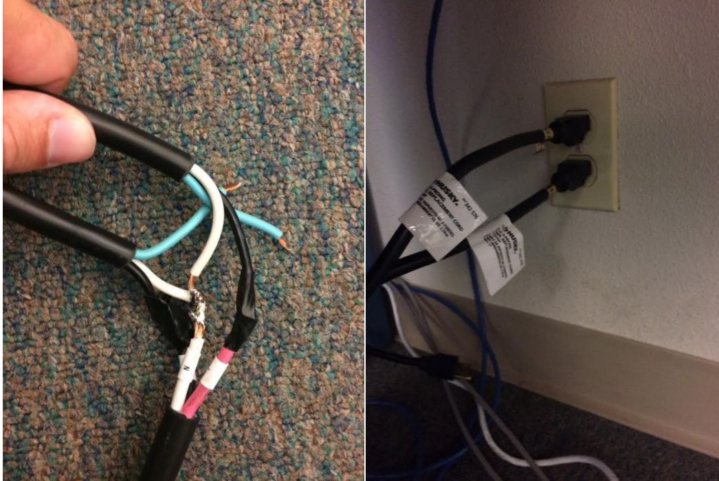
Figure 5 - 4: Microinverter to wall bare wires and plug connection
