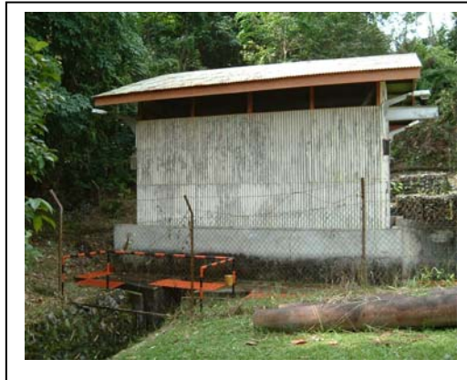
Figure 5 – SESCO turbine house
