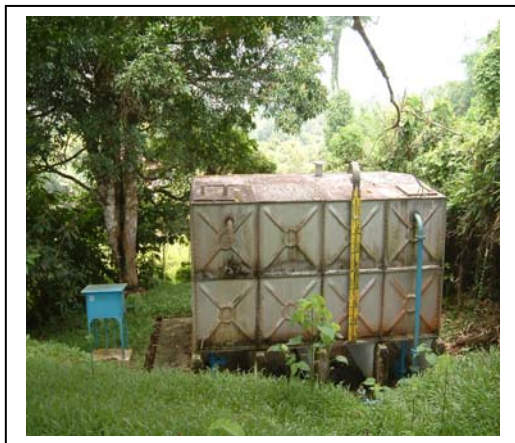
Figure 12(d) – The storage reservoir
