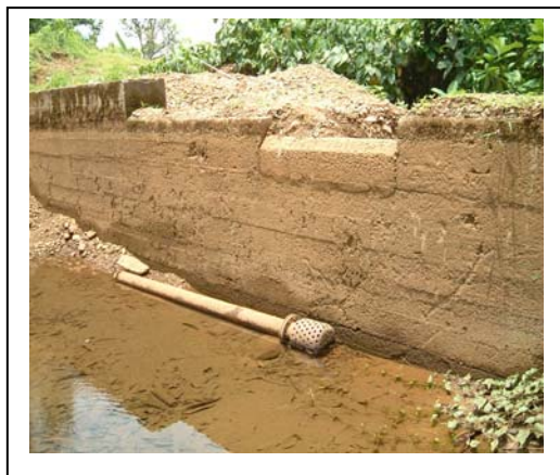
Figure 12(a) – The concrete weir and water intake
