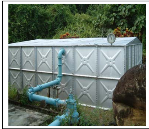
Figure 3 (f) – The high level storage reservoir next to the slow sand filter
