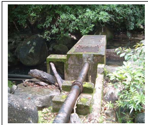
Figure 7 – Collecting chamber for inflow from SESCO to supplement shortage of raw water at the intake
