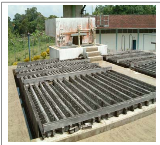
Figure 9(a) – The aerator and mixing channel for chemicals dosing and baffled flocculation tank
