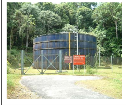
Figure 10(d) – The elevated high level storage reservoir
