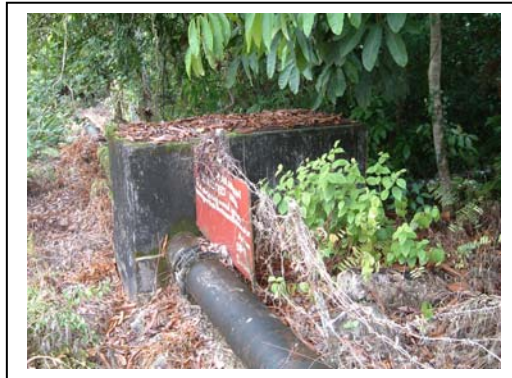
Figure 6 – The “tee-off” concrete chamber
