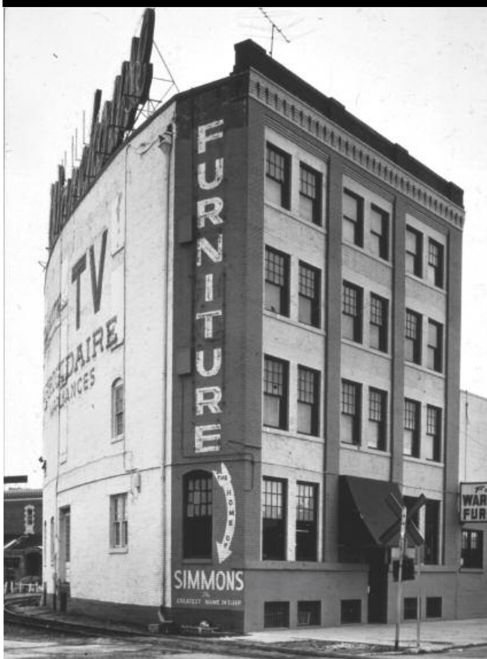
Foster's triangular "flat-iron" warehouse was rounded to accommodate the railroad's downtown right-of-way. The curved north face of the 1910 building has since been encapsulated by a parking garage.
