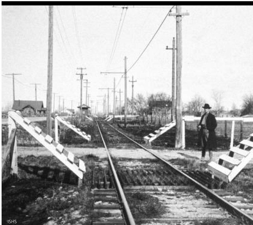
Cattle guards at a West Boise trolley crossing. Streetcars linked Boise to Ustick in 1907.
