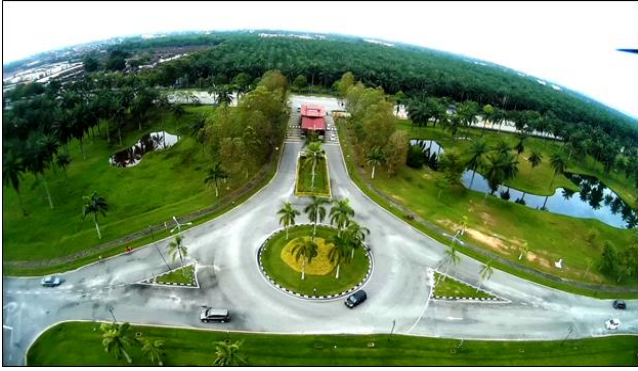
Figure 6 Traffic condition at entrance A
