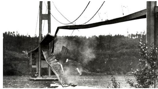
Figure 1 Collapse of Tacoma Narrows Bridge, 1940, USA [14]
