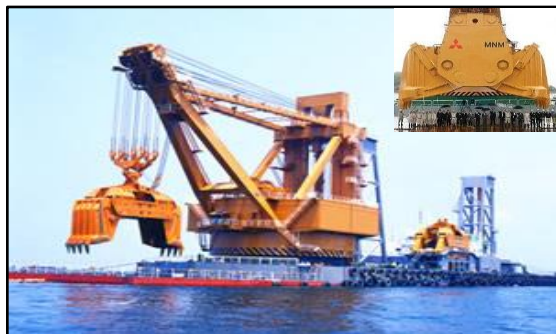
Figure 6 The world's largest & heaviest grab dredging system
