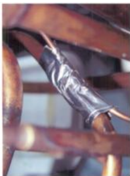
Figure 4: Capillary tube-discharge line heat exchanger
