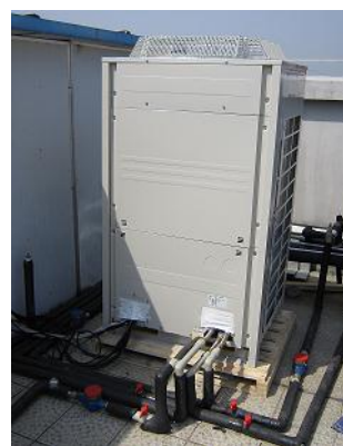
Figure 8: HVAC&DHW system: (a) layout of pipe system (Simplified version in cooling mode); (b) Hybrid HP unit
