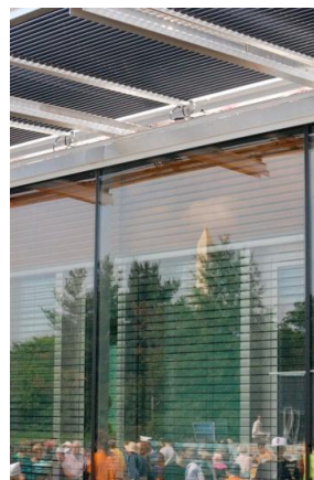
Figure 15. View of the south façade during the competition week at the Solar Decathlon 2011. The Washington Monument can be seen in the reflection.
