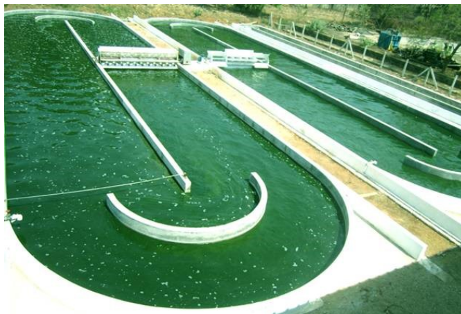
Figure 1.3 Open Pond reactor (Photo: Aban Infrastructure Ltd)
