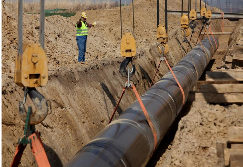
Figure 2-1. Pipeline construction: lowering the pipeline in a trench [17].
