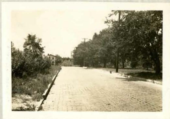
Looking south from Boulevard and Palm Ave.- Site north approach to proposed bridge. Street here 50 ft. wide, roadway 26 ft. Need widening to 60 and 40 ft. respectively at this point.
