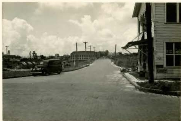
Looking south on Garcia Avenue from Palm Avenue toward bridge to be replaced.
