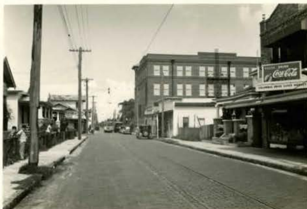
Looking west toward Regensburg factory. Note roadway clogged by street car and vehicles. Street here 40 ft. and roadway 28 ft.
