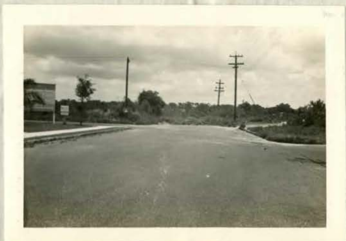
Looking north from corner Spruce St.- Site of south approach to proposed bridge. Street here 55 ft. wide, roadway 40 ft. Adequate roadway here.
