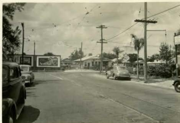
Tampa St. at its northern terminus at Buffalo Ave. Street has 60 ft. wide, roadway 42 ft. Street should be projected from here to Florida Avenue.
