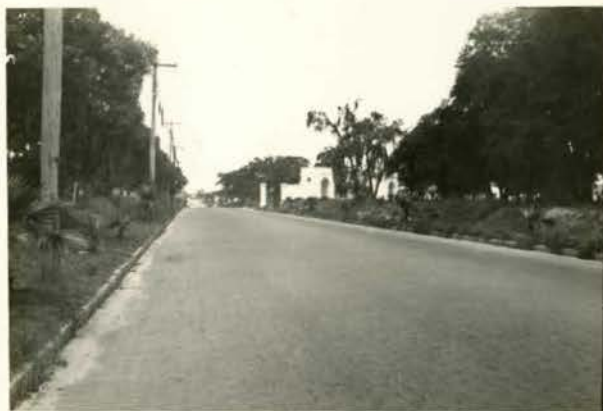
West of the river Columbus Drive has a street width of 60 ft. and roadway of 40 ft.
