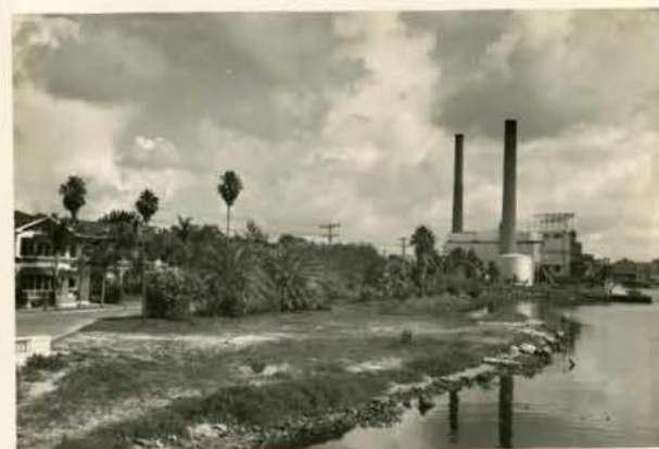
West side river from Platt St. Bridge.
