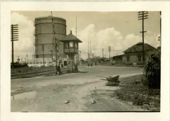
Grade crossing at 13th St. and 5th Ave.
