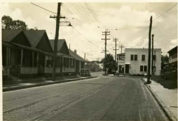
Severe jog in Jefferson St. north of Harrison Street.
