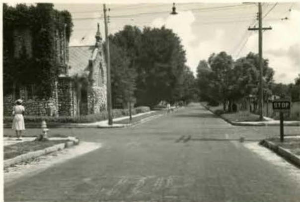
Looking north on Central Avenue from Columbus Drive. Street here 50 ft. wide, roadway 25 ft. Both need widening to 60 and 40 feet respectively.
