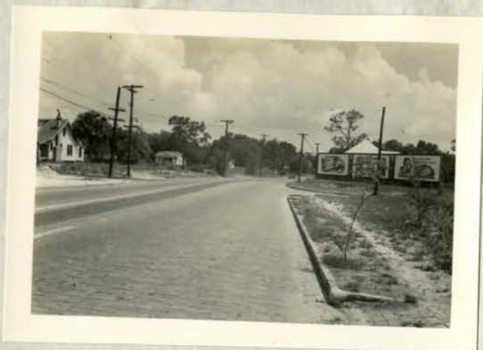
South on Tampa Street. Street here 60 ft. wide, roadway 30 ft. Curve on right side and sign board abstraction could be removed.
