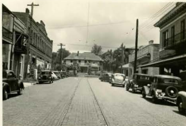
Dead end at Franklin and Oak Steets--site of proposed connection with Florida Ave. and Tampa St.
