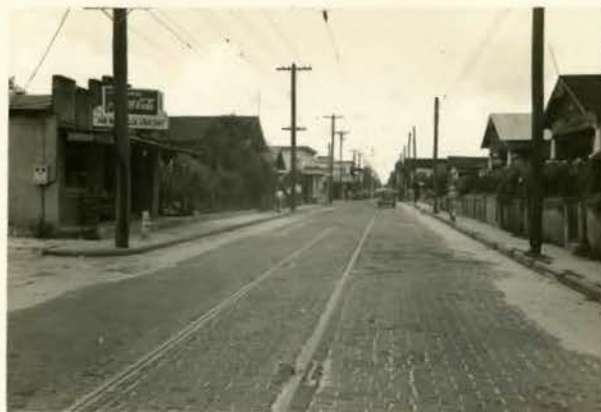
Columbus Drive looking west toward 22nd St. Note poor condition of street surface, also car track. Street here 40 ft. wide, roadway 30 ft. Need widening to 60 and 40 feet respectively.
