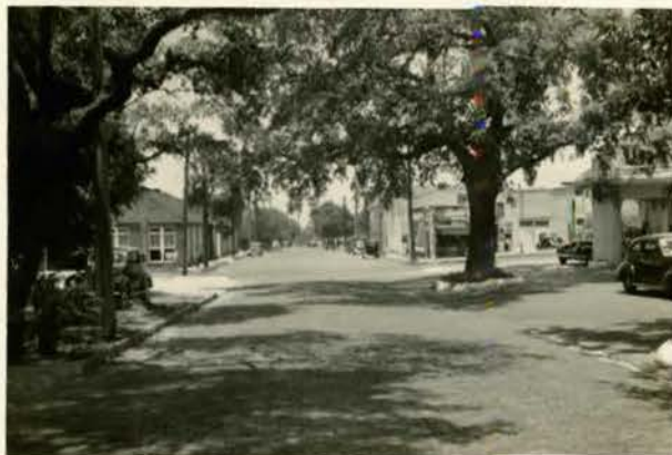
Showing roadway widening west of Florida Avenue.
