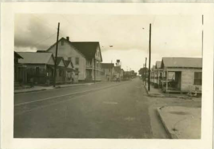
Nebraska Ave. north of about India St. Street width here 50 ft. wide. Roadway widening already carried to point where it has narrowed sidewalks and encroached upon fronts of houses.
