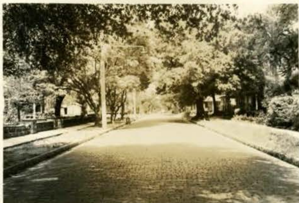
Looking west from near Tampa St. Note improved appearance of streets here. Street 40 ft. wide, roadway 28 ft.
