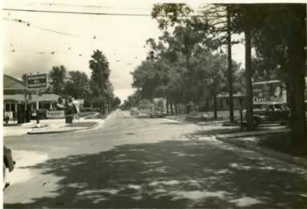
Central Avenue north of Buffalo Ave. Offset here on roadway. Street 60 ft. wide and roadway 30 ft. Roadway should be widened to 40 feet here.
