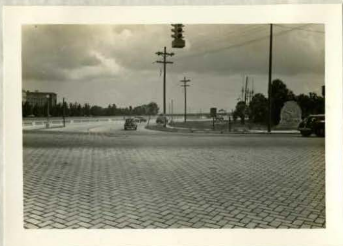
West approach to Platt St. bridge looking toward Bayshore Drive. Traffic circle enstalled here would insure steady flow of traffic and elimination of traffic light.
