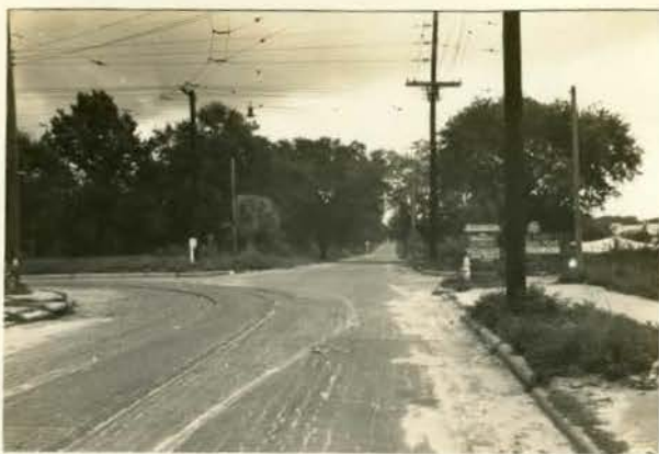
East of 29th St., Columbus Drive should be widened to 60 ft. and roadway to 40 ft.
