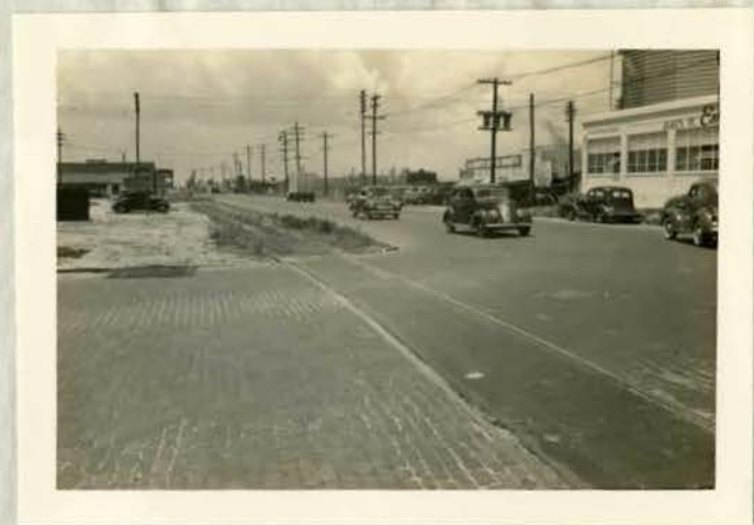
13th Street south from 4th Avenue. Sharp curb radius should be rounded.
