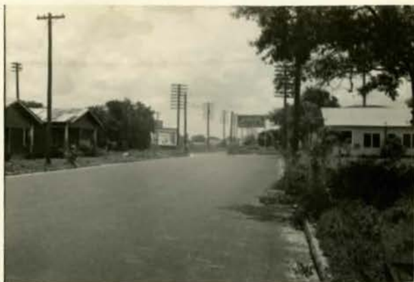
Jog in 4th Ave. that should be removed. Street at narrow part 30 ft. wide, roadway 29 ft.
