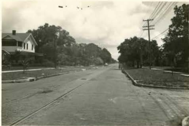
Central Avenue north of Mohawk Ave. Here street has width of 80 ft. and roadway of only 30 ft. Roadway could easily be widened.
