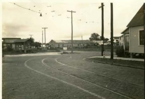
Severe jog at La Salle St. and Boulevard that should be removed.
