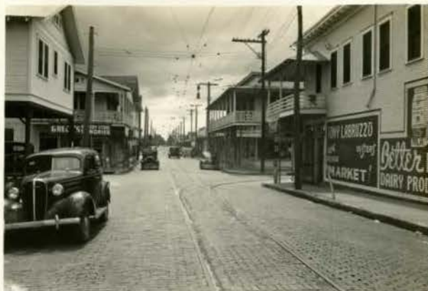
Looking east from 15th St. Street width 40 ft., roadway 28 ft. Widening here to 60 and 40 for street and roadway respectively.
