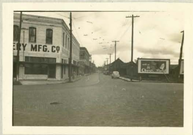
Looking north on Central Ave. from Cass St. Street only 40 feet wide here and roadway 30 ft. Both need widening to 60 and 40 ft. respectively.
