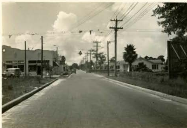
Boulevard looking south from Columbus Drive. Street 50 feet wide, roadway 26 feet need widening to 60 and 40 feet respectively.
