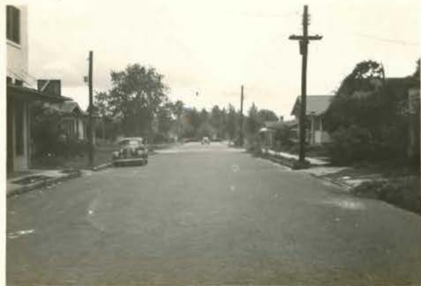
Looking north on Central Avenue toward Robles Park from Floribraska Avenue. Note here street is 50 ft. wide and roadway 34 ft.
