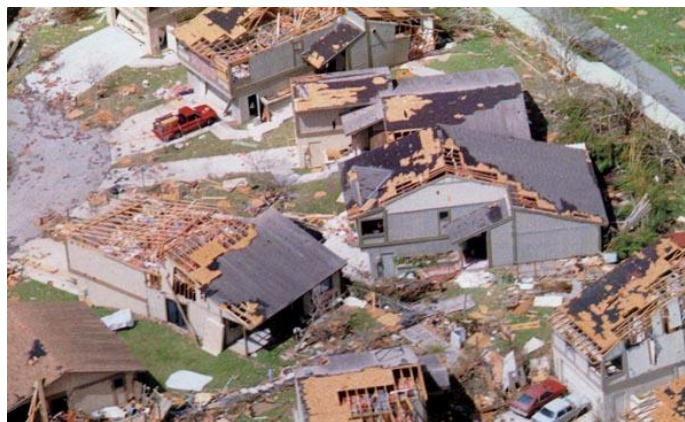
Figure 1.1 Roof damage from Hurricane Andrew, www.floridadisaster.org
