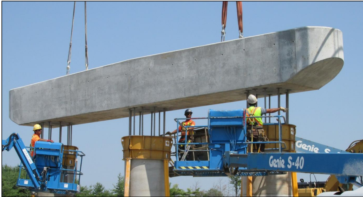
Figure 6: Pier Cap Installation
