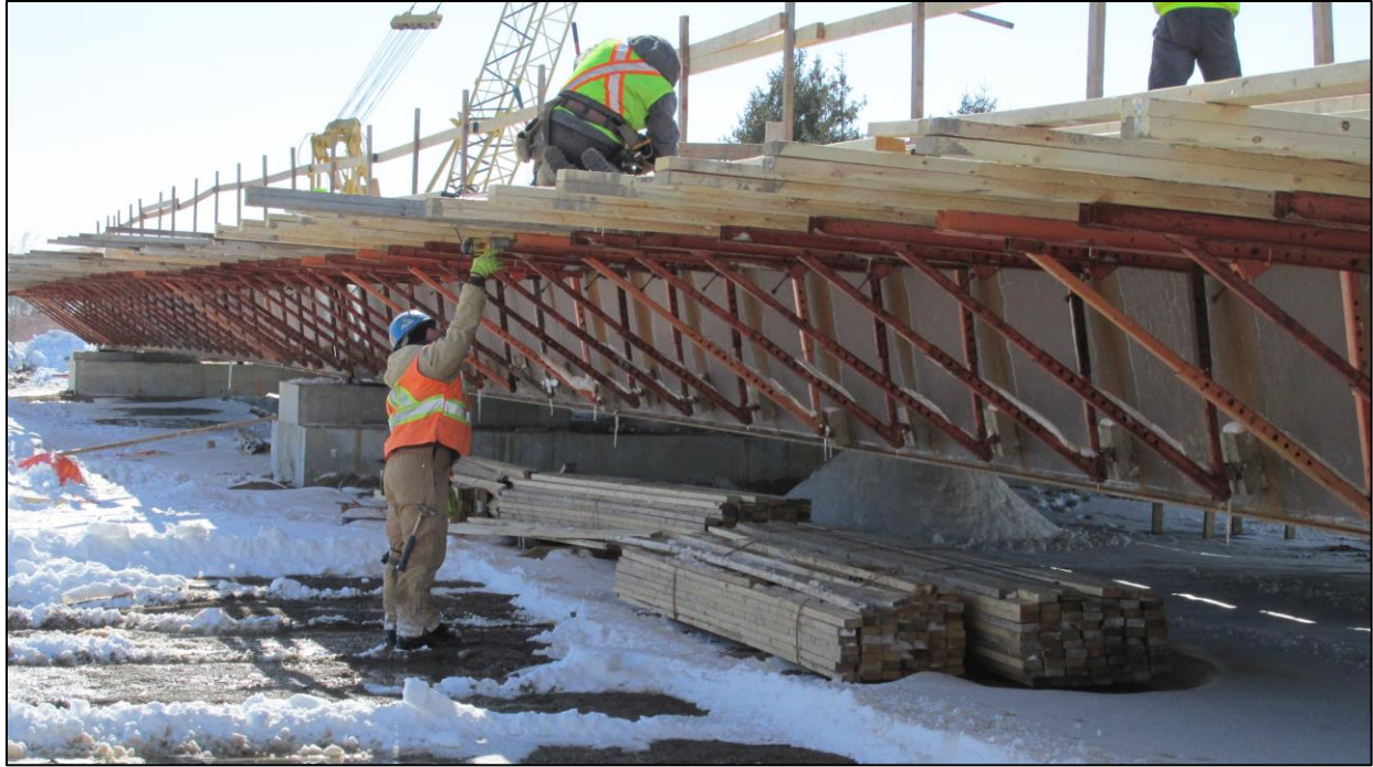
Figure 8: Supermodule Construction in Temporary Yard
