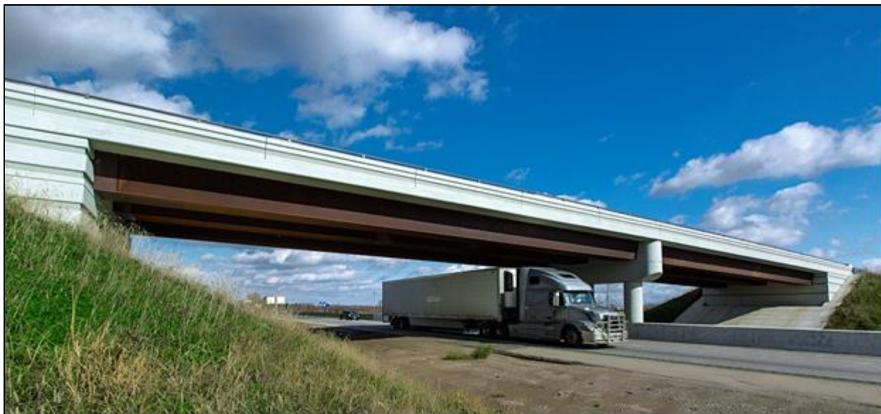
Figure 10: Westminster Drive Underpass
