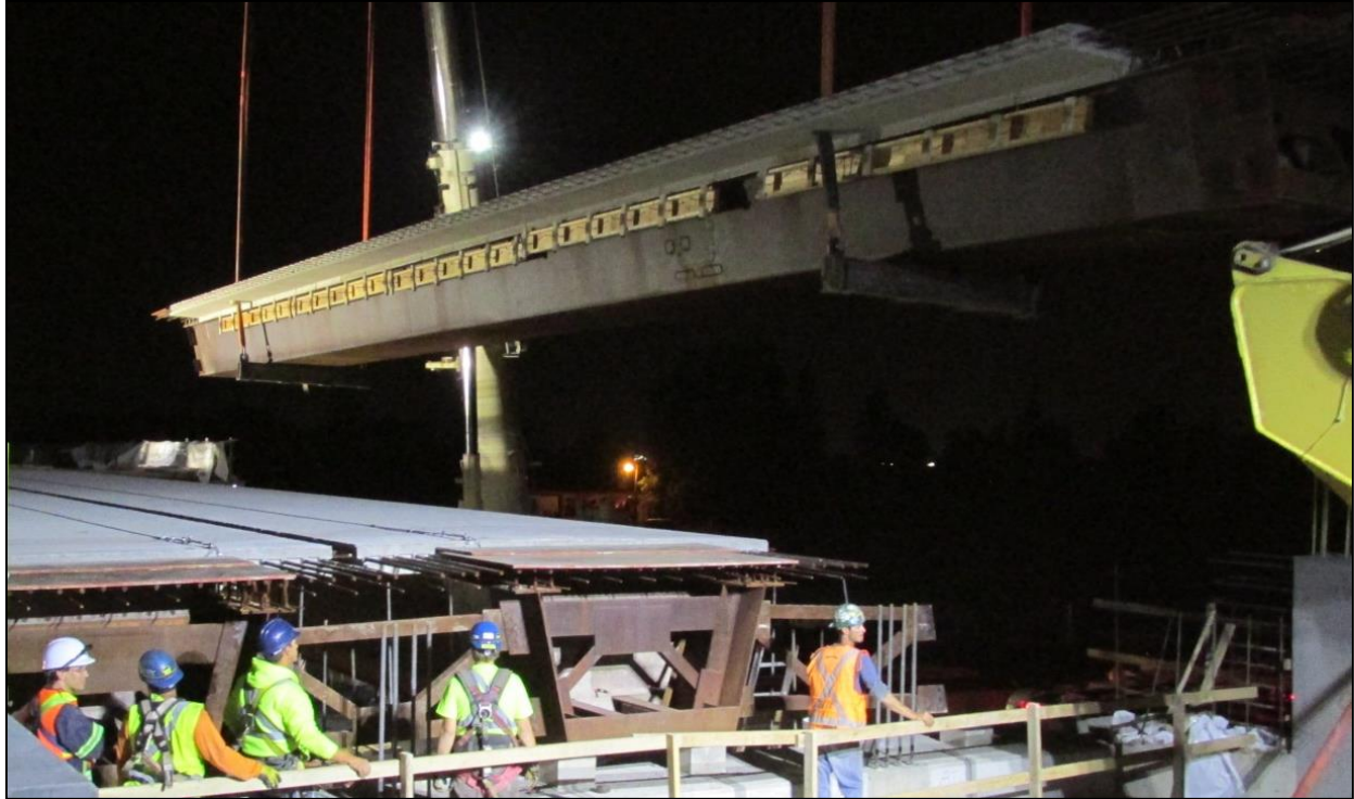
Figure 9: Supermodule Installation
