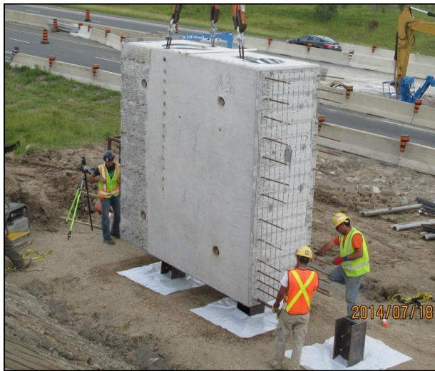
Figure 4: Prefabricated Abutment Stem Segment
