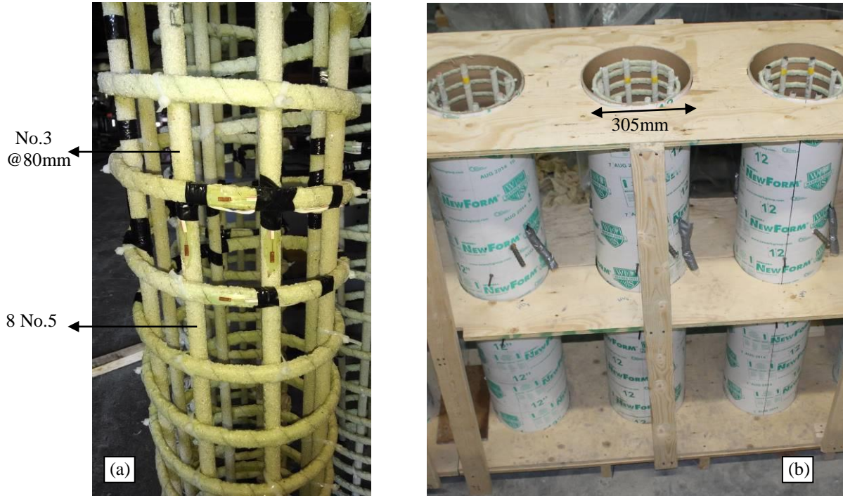
Figure 1: GFRP cages, (a) internal instrumentations; (b) cages inside wooden formwork
