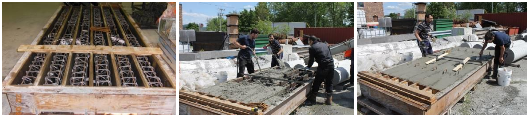
Figure 3: Fabrication of the beam specimens
