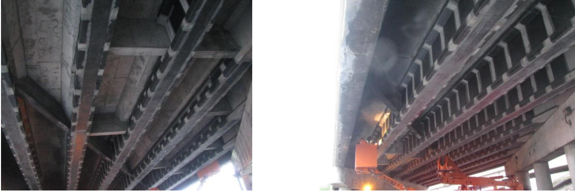
Figure 2: Girders with CFRP Wraps
