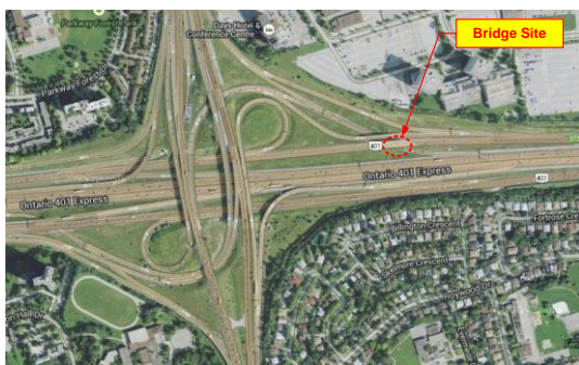
Figure 1(a): Bridge Site at Highway 401 and Highway 404
