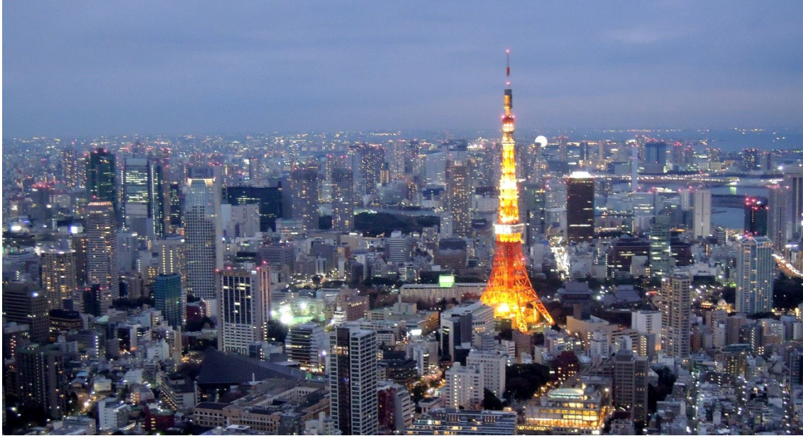
Fig. 92. Picture of the Minato Ward Skyline as 2016. (Photo by Author).
