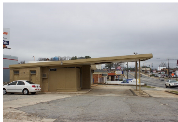
1950's Construction, 4124 Lawrenceville Highway
