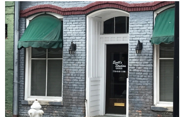
Inappropriate exterior balloon awnings detract from the historic character of the façade.
