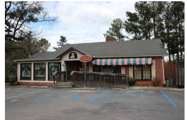
Inappropriate residential-to-commercial conversion illustrating improper parking and use of architectural elements.
