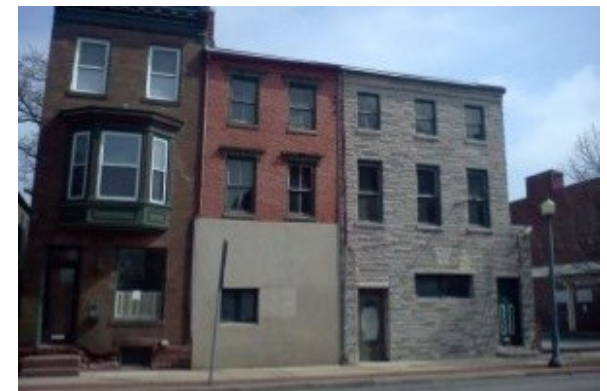
Inappropriate new construction with closed in storefronts. This type of infill breaks the historic language of the district.
