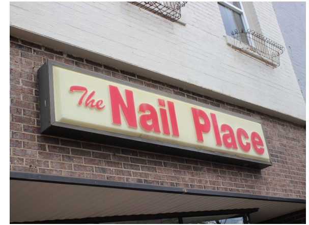
Inappropriate plastic light box wall sign material
