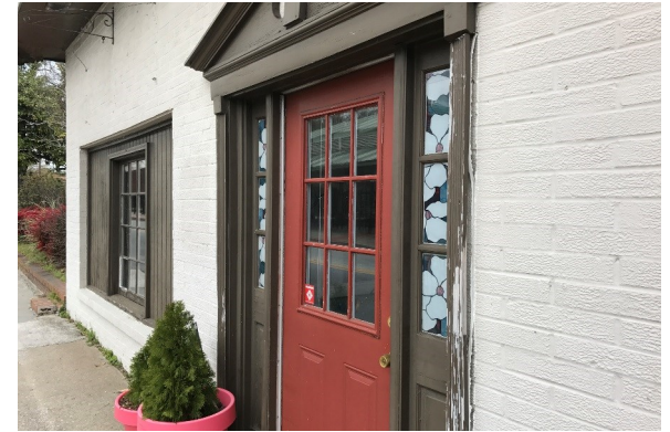
Wood panel infill and residential doors added to entrance
