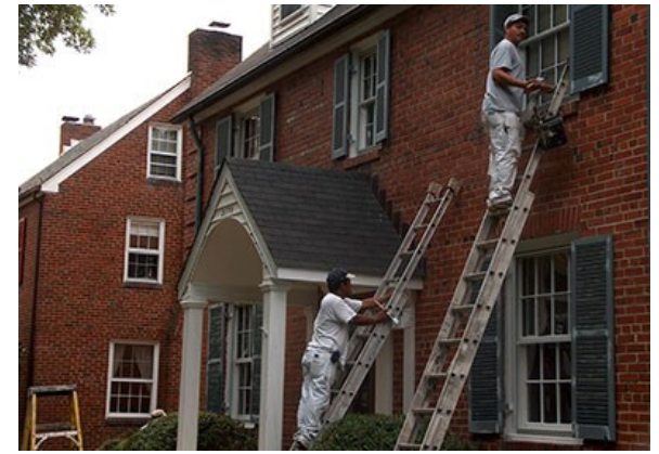
Subcontractors performing façade maintenance.
