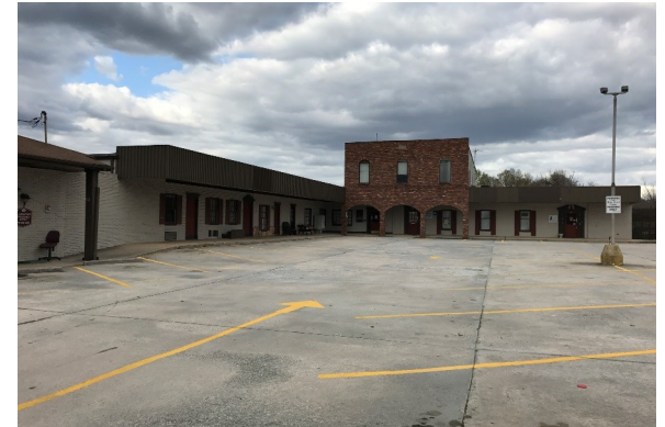
Improper landscaping and hardscape that detracts from public interaction and community gathering.
