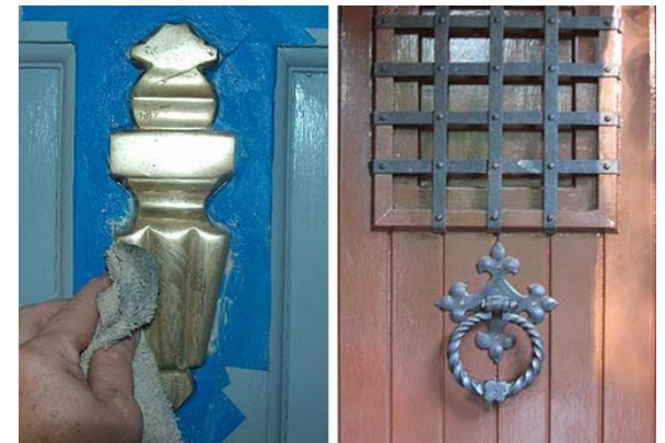
Door maintenance and conservation.
