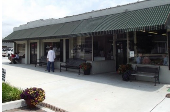
2293 Main Street in Tucker illustrates successful site development that incorporates a variety of activities and interactions into the community.
