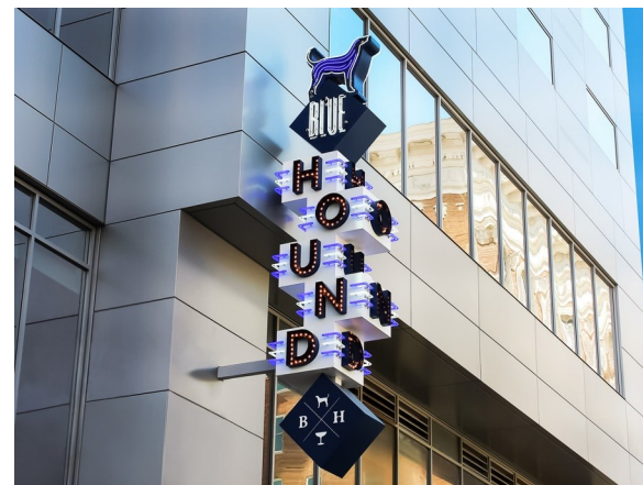
Inappropriate projecting neon sign that is not original to the building or context.
