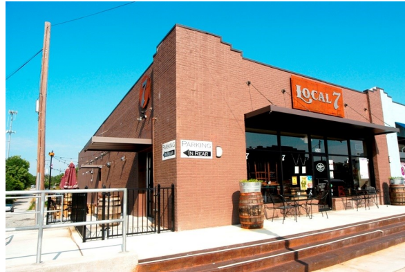
4236 Main Street, successful new construction illustrating proper use of patio elements for a seating and dining.
