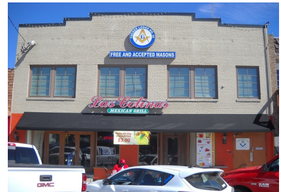
Two-Part Commercial Block, 2327 Main Street
