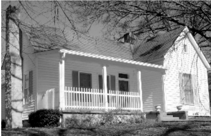
Figure D11 – This is an example of a gabled-ell cottage found on East Mountain Street.
