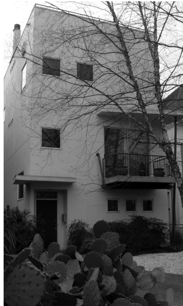
Figure G24 – While flat roofs may be appropriate in the Stone Mountain commercial character area, they are not in the residential character areas, where the Compatibility Principle would necessitate that gabled or hipped roofs traditional to Stone Mountain’s historic houses are most appropriate.
