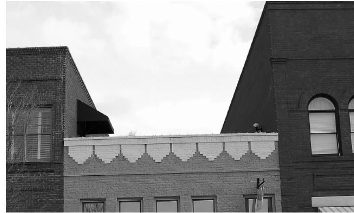
Figure G13 – The roofs of these new commercial buildings are recommended because they are flat, which is compatible with the historic commercial buildings found in Stone Mountain.
