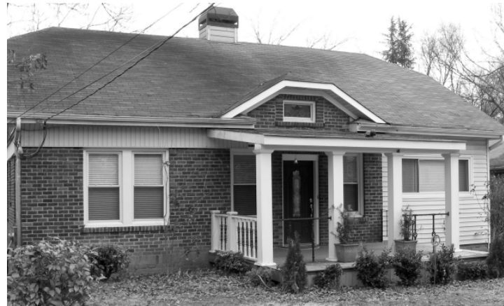
Figure F24 -The porch that has been added to the front of this historic house is not recommended because the materials are not compatible with the house. The railing is also not recommended because it is not complementary to the design of the house.
