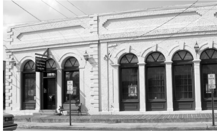
Figure E7 - The original materials, door location and general design of this commercial storefront have been maintained, which is recommended for historic storefronts in Stone Mountain.
