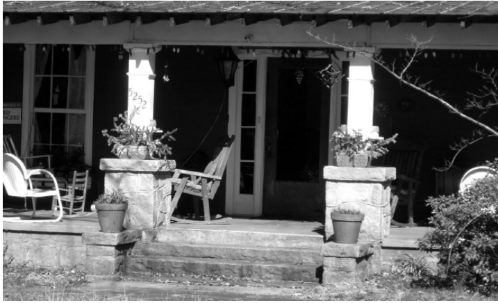
Figure E15 - The original configuration of this porch has been well maintained; no enclosures or additions have been made, allowing it to maintain its integrity.
