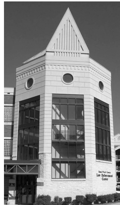
Figure G2 - This new commercial building does not have a recommended massing or scale and would not be compatible for new construction in Stone Mountain. Historic commercial buildings in Stone Mountain are of two stories or less, so new construction that is three stories or more would not be recommended.
