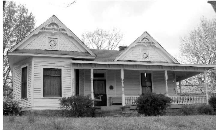
Figure D41 – This is an example of a Queen Anne style house located on Sheppard Road. Note the asymmetry of the façade, the shingles in the gables and the detail in the wood trim.
