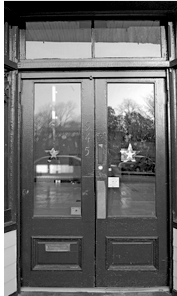
Figure E2 – Historic doors in the commercial character area of Stone Mountain are made of wood and most are at least half glass. Historic doors should be maintained.
