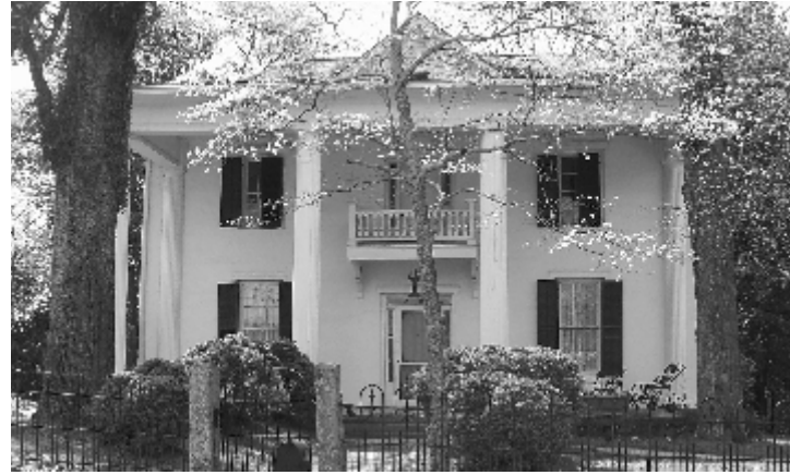
Figure D39 – This is an example of a Greek Revival style house found on Ridge Avenue. The two-story columns, small porch over the door, side lights, and transom light over the door are all elements of the style.
