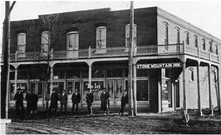
Figure B1 - This photograph shows the Stone Mountain Inn, at the corner of Main Street and Manor Drive, when it still had its balcony. This would be a good resource for reconstructing the balcony on the current building.
