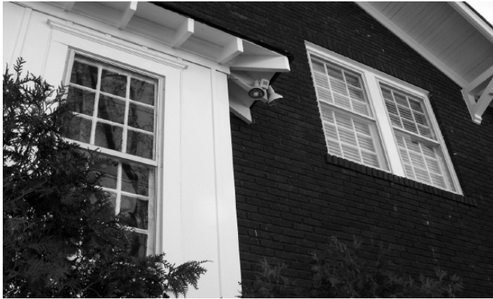
Figure E13 - This house's historic windows exhibit storm windows that do not interrupt or conceal the historic glazing pattern.
