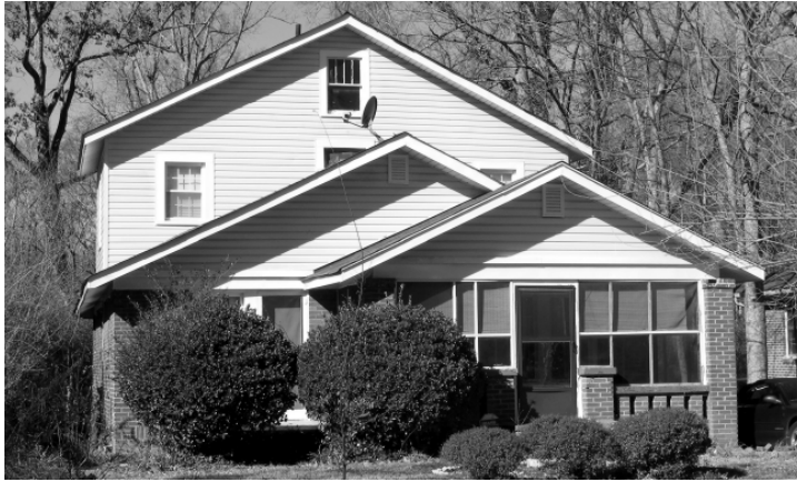
Figure F26 -The rear addition is out of scale with the original house in front. Its roof line is higher than that of the original building, which significantly alters the house's integrity.
