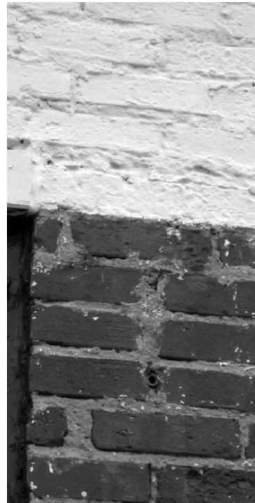
Figure E11 – Painting brick that was historically unpainted diminishes the historic integrity of the material and associated building and is not recommended.
