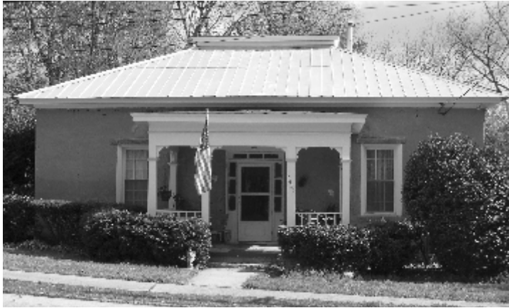
Figure D38 – This house on East Mountain streets has elements of the Georgian style such as a transom light above the door and double-hung windows with multiple, small panes of glass.
