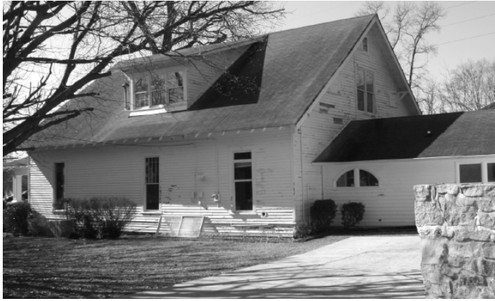
Figure F13 -If added to the rear of the house, this roof dormer would be a recommended addition.
