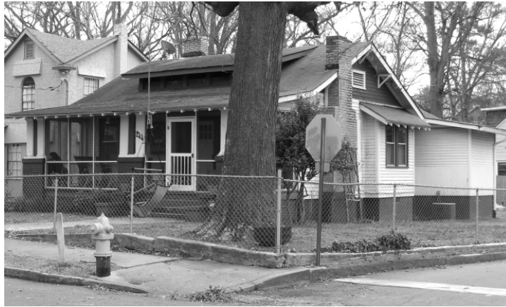
Figure F19 - This addition has been constructed using recommended materials. The materials, primarily wood, are complementary to the historic house.
