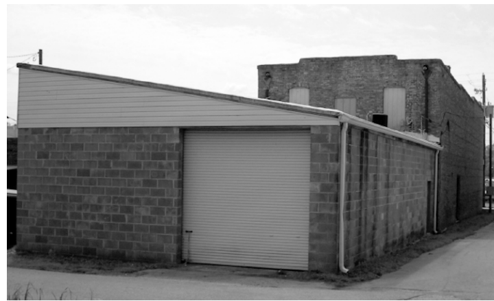
Figure F5 - The general design of this addition is not recommended because it does not complement the historic building. The materials also are not recommended because they are not compatible with materials used in the historic building.
