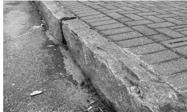
Figure J3 - The granite curbing used on sidewalks is a historic element that should be maintained. Brick pavers are also recommended materials for use on sidewalks.
