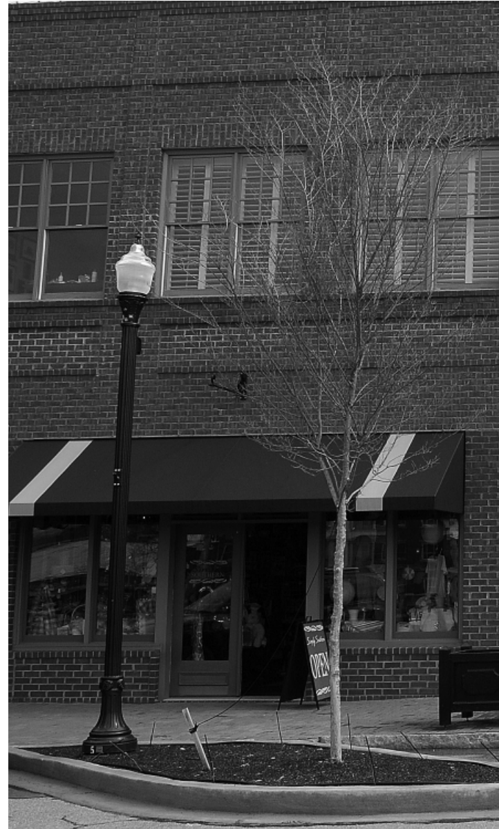
Figure G6 - The storefront design of these new commercial buildings is recommended because it has large display windows and doors with wooden frames and large panes of glass, similar to historic storefronts.
