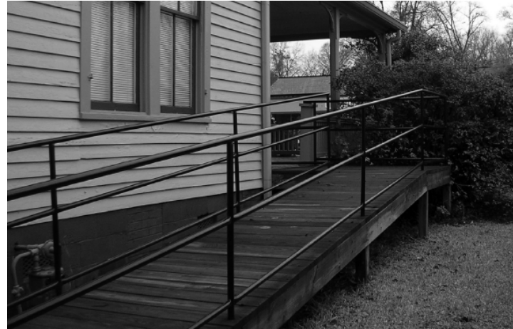
Figure G25 – Accessibility ramps should be located on the side or rear of the building and screened from view of the public right-of way
