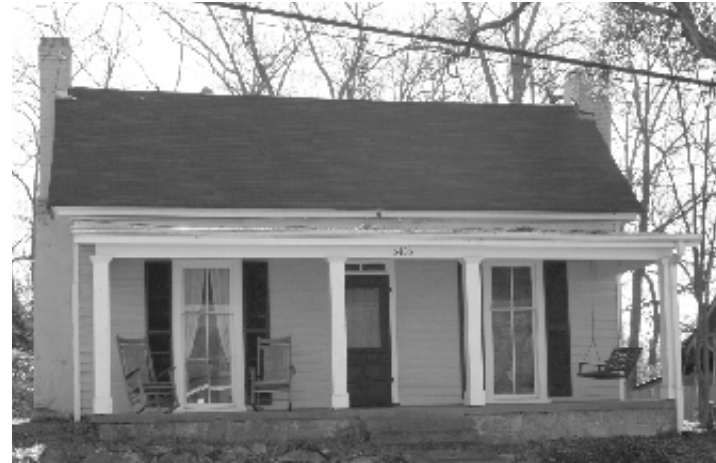
Figure D5 – This central hallway house is located on East Mountain Street. The two end chimneys and the central doorway are characteristic of the house type.
