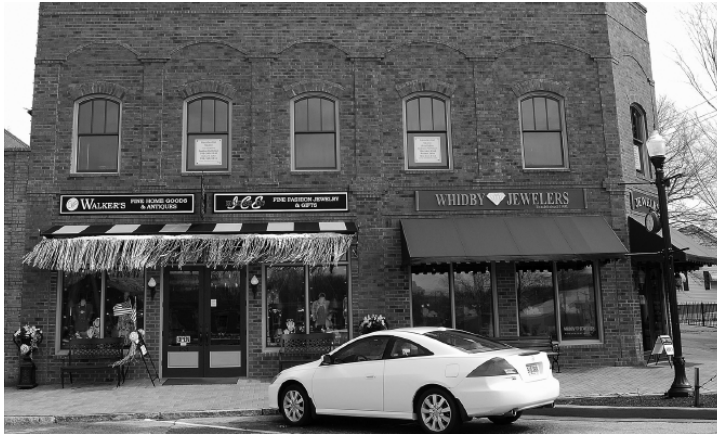
Figure G4 - This new commercial building has a recommended design that is compatible with historic buildings on the surrounding block face. The building can be differentiated from historic commercial buildings by its use of slightly more contemporary materials and less ornate details than those of a historic commercial building, but the materials and design used do not detract from the historic character area in which it was built.
