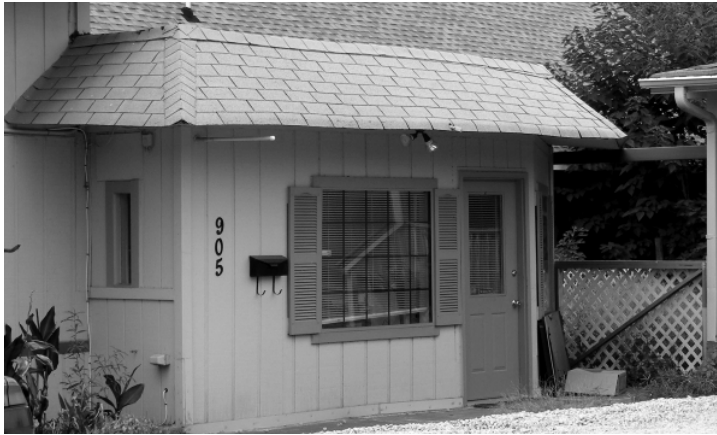
Figure F4 - The general design of this addition is recommended because it can be differentiated from the original building and the design mimics enough of the design elements of the original building to be complementary.
