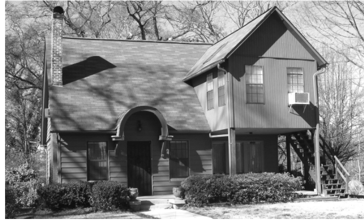
Figure F14 - This type of addition is not recommended because it is located on the front façade of the building, which obstructs the view of the historic house.
