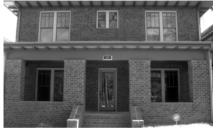
Figure G21 – This new house in Midtown Atlanta exhibits a 6-over-1 window pattern consistent with the other homes on the block. It's a good example of a recommended approach for windows on new construction in a historic neighborhood.
