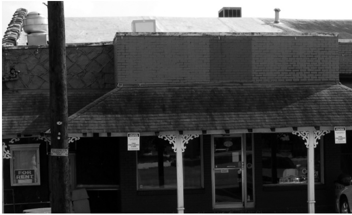
Figure E6– This air conditioning unit has been installed on the rear of the building, where it is not visible and does not obstruct the façade of the historic commercial building.
