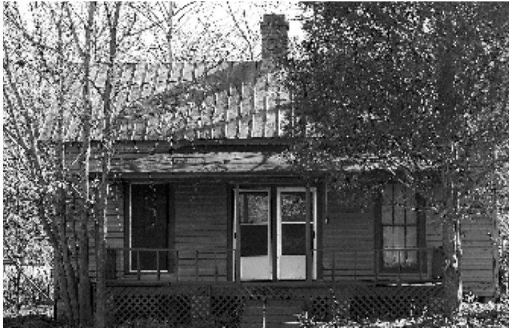
Figure D3 - This is an example of a saddlebag found on Main Street.
