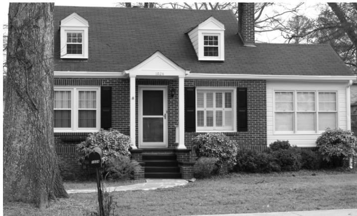
Figure F20 - The addition of this extra room enclosing a porch is not only not permitted in Stone Mountain, but it also uses materials that are not recommended for use on historic houses in Stone Mountain. The use of vinyl siding is not recommended.
