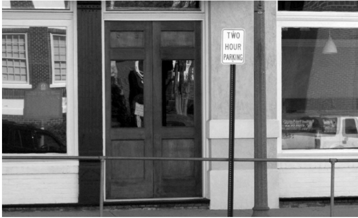
Figure F8 -This door is recommended because it uses materials that are complimentary to the historic doors in Stone Mountain and it does not detract from the historic nature of the building.
