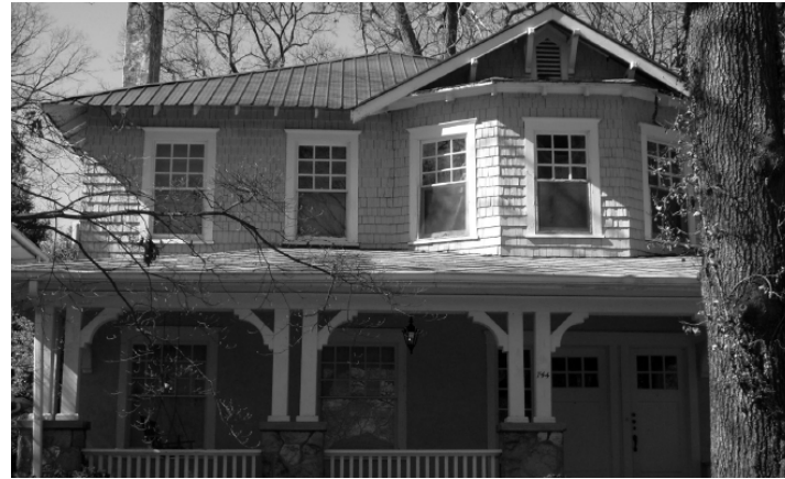
Figure E16 – This house’s historic roof has been replaced with a standing-seam metal roof that is inappropriate in material for the house.
