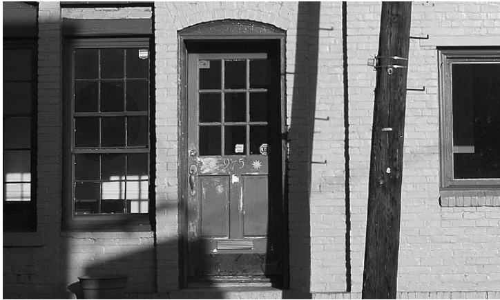
Figure F10 - The window on the left, although it is not original to the building, is complimentary and does not detract from the historic nature of the building.
