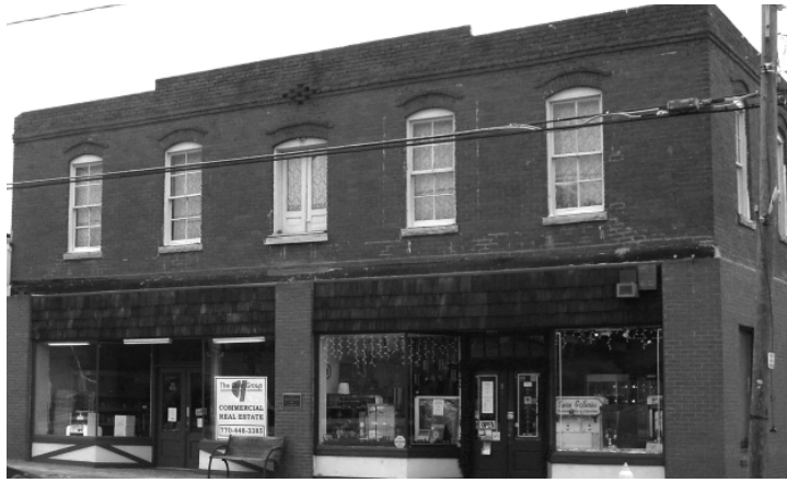
Figure E3 - There are multiple types of non-display windows within the Stone Mountain commercial character area. Multi-light, double hung types are most common, as can be seen on the two-story brick building in this photo.
