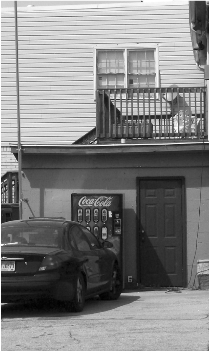
Figure F11 – The roof of this addition is flat, like that of the historic building it is associated with, which is recommended.
