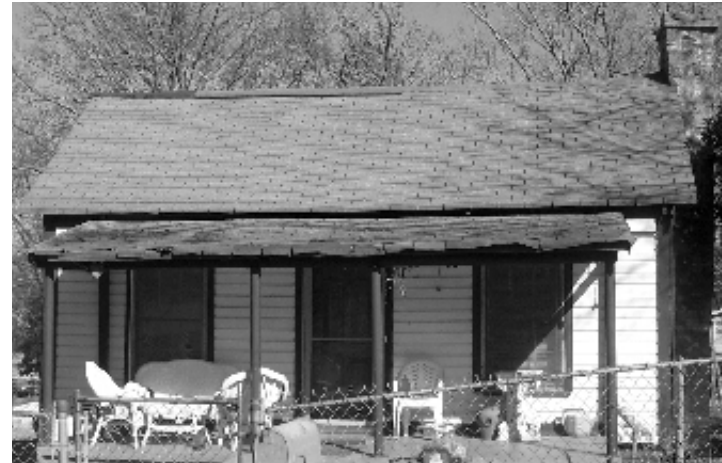
Figure D1 - This is an example of a hall-parlor type house found on Stillhouse Road. The door is at the center of the front façade, but the house has the small size of a Hall-Parlor type house.
