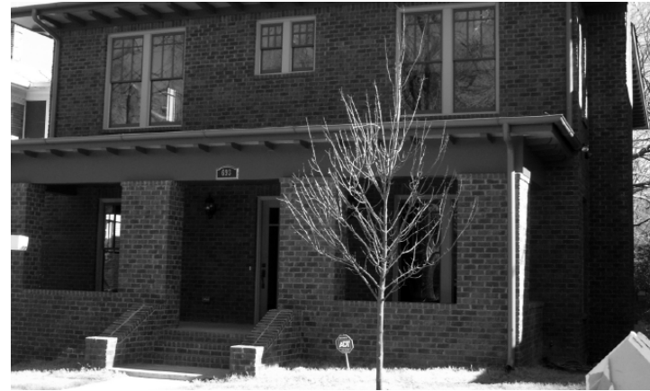
Figure G23 - This new house in Midtown Atlanta exhibits a full-length porch on the front façade. As the full-length porch is a character-defining feature of the houses in Midtown Atlanta, this is an appropriate new porch for the neighborhood and block face.
