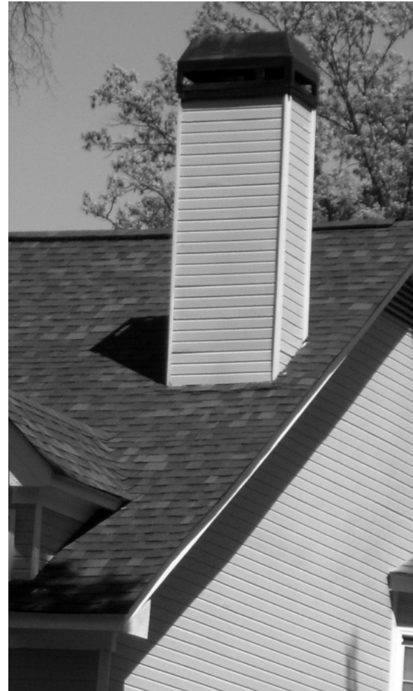
Figure G19 –The inappropriate use of siding veneer on chimneys is a common inappropriate use of materials in historic districts. While siding on the house itself may be appropriate, historic chimneys in Stone Mountain are constructed of masonry.
