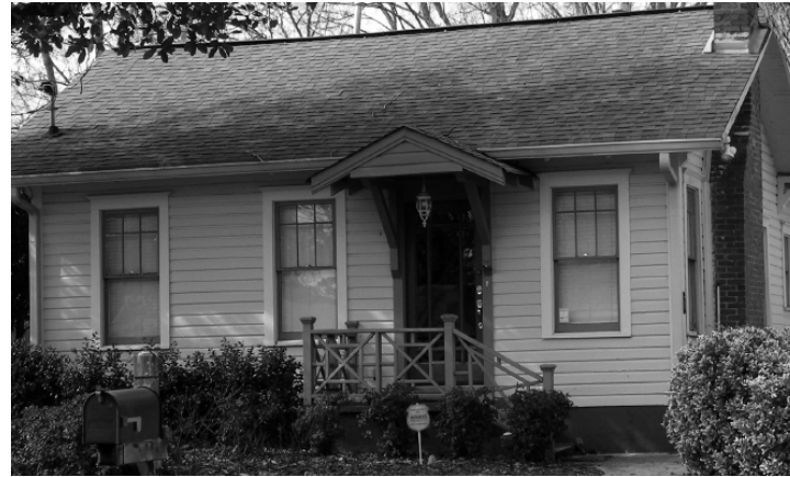
Figure E12 - The door on this historic house has been replaced with a more modern door that has multiple panes of glass. This is not compatible with the historic nature of the house and is not recommended
