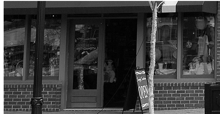
Figure G9 – The doors used in this new commercial building are compatible with doors that would be found on historic commercial buildings in Stone Mountain and are recommended.
