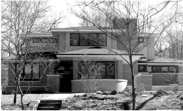
Figure G22 - The windows used in this new house are not compatible with the windows of historic houses that surround it. The windows are made with a reflective glass, they are set in metal frames and the windows are made of single panes of large glass. None of these elements is compatible with windows found on historic houses in Stone Mountain, therefore this style of window is not recommended for use on new homes.
