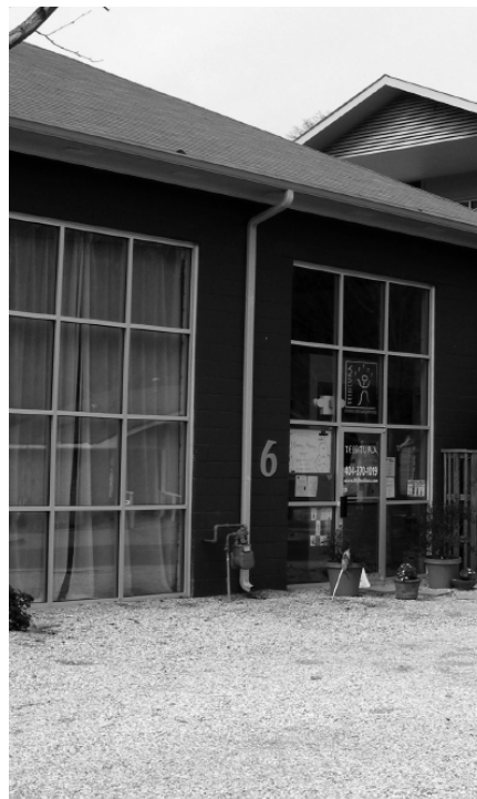
Figure G12 – The windows of this new commercial building have metal frames and numerous panes of glass that span almost the entire height of the building. This is not compatible with windows found on historic buildings in Stone Mountain and is not recommended.
