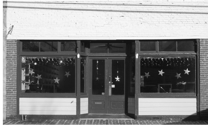
Figure E1 - The general design of the historic storefronts in Stone Mountain includes a recessed front door with large display windows and transom lights above the windows and door.
