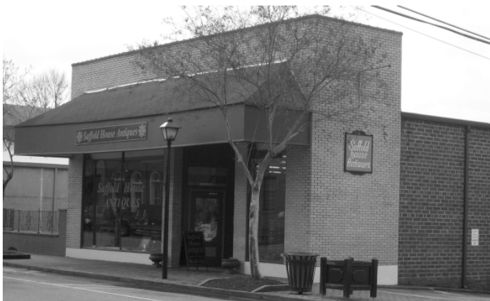
Figure F2 - The location of this addition is not recommended, because it has been added to the primary/ front façade of the historic storefront.
