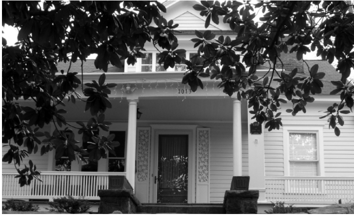
Figure G20 – This historic house exhibits a historic wood door with a single fixed light. When constructing new houses in Stone Mountain, one should follow the Compatibility Principle for character-defining architectural detail such as doors by observing what historic details are common on the block face.
