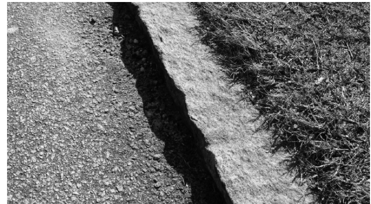
Figure J7 - The curbing in residential areas is of various materials, including granite. When these historic curb materials exist, they should be maintained.
