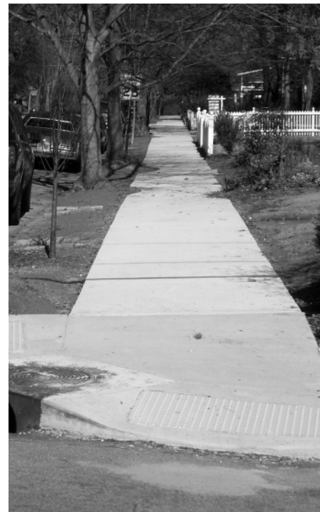
Figure J4 - This design is not recommended because historic materials have not been used and new curb cuts have been made.
