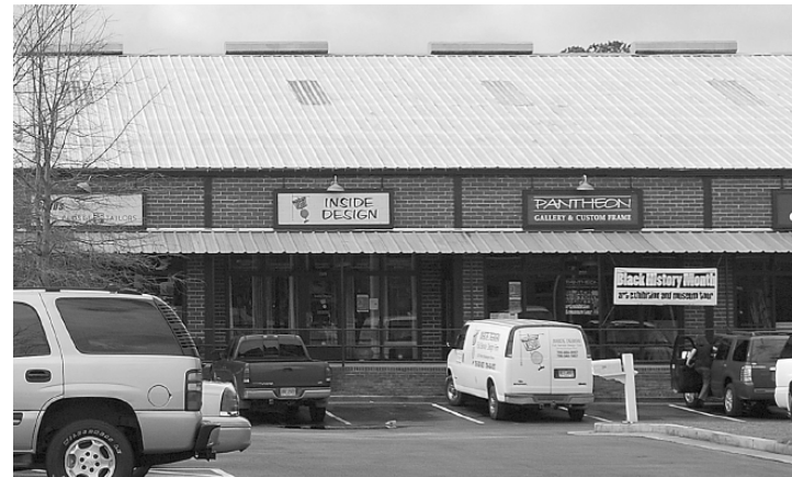
Figure G14 – The roof of this new commercial building is not of a recommended design because it has a pitch that is not compatible with historic buildings that would be found in Stone Mountain.
