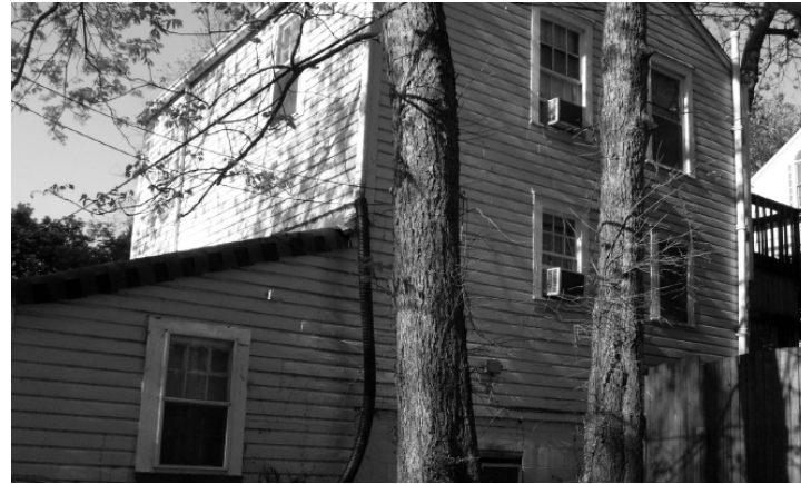
Figure F22-The shed-roofed rear addition to this historic residential building exhibits the same 6-over-6 windows as are found on the historic building. The matching of window light patterns is just one of the elements that make this addition compatible with the historic building
