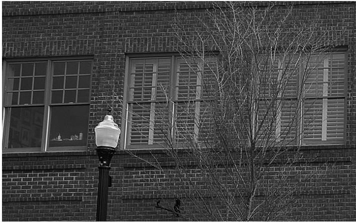
Figure G11 – These windows are compatible with windows that are found on historic commercial buildings and are therefore of a recommended design.
