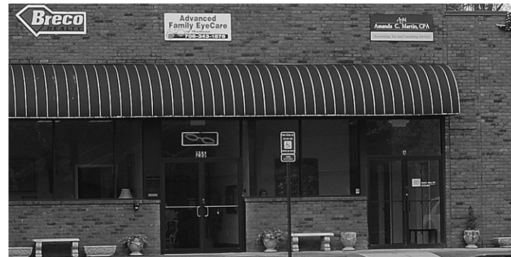
Figure G10 – The doors used in this new commercial building are not compatible with the doors that might be found on historic commercial buildings.
