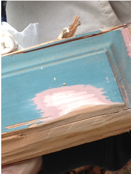
Paint layers on back of front door
