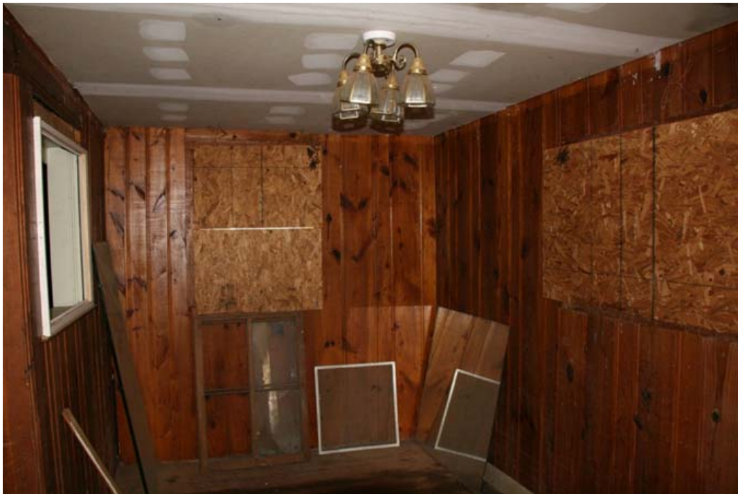
CA Figure 28: Room 111-Boarded windows, wood-paneled walls
