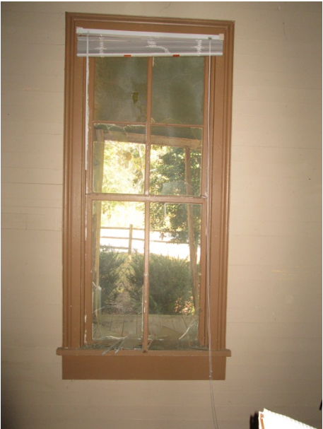
AD Figure 16: Window on north wall of Room 101
