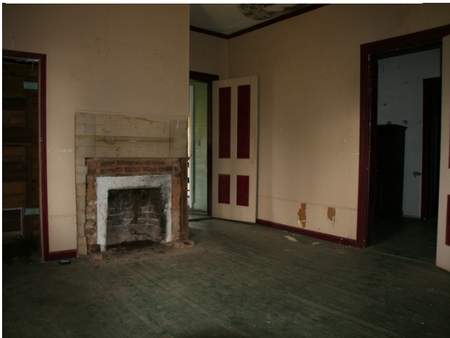
AD Figure 27: Northeast view of Room 105 with Door D7 and D9
