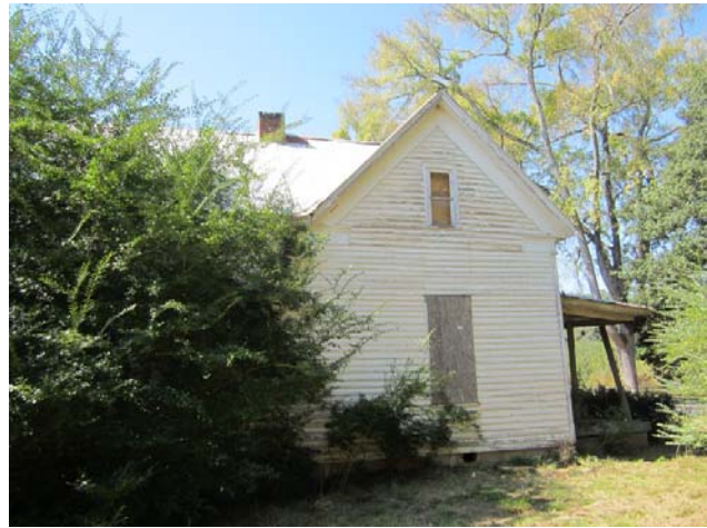
AD Figure 8: East facade of the Sherrill House with a one-over-one window on second story
