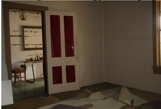
BC Figure 1: Four-panel wood Victorian door in Room 101
