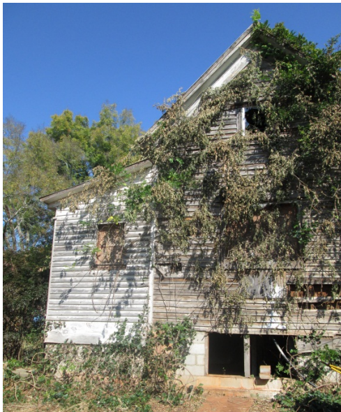
AD Figure 5: Access to the crawlspace under the house
