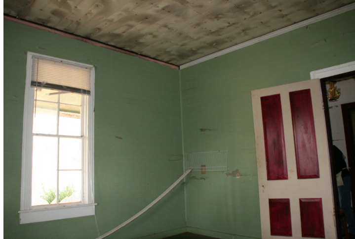
Room 103 wall and window
