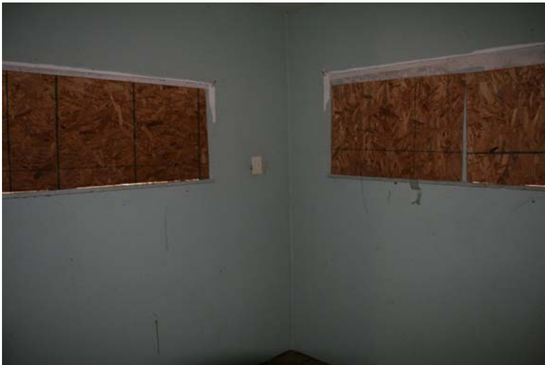
CA Figure 26: Room 109-Gypsum board walls; boarded windows
