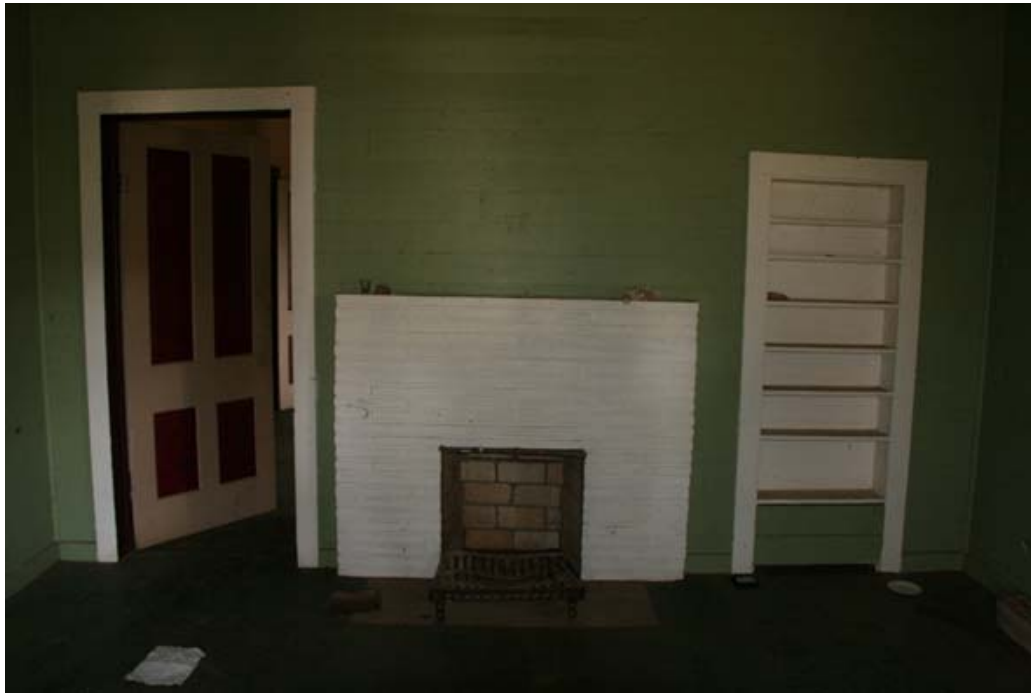
CA Figure 21: Room 103- Built-in bookshelf, coal burning fireplace
