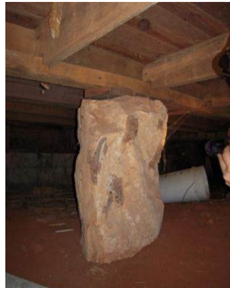
AD Figure 4: Marble pier from foundation of house
