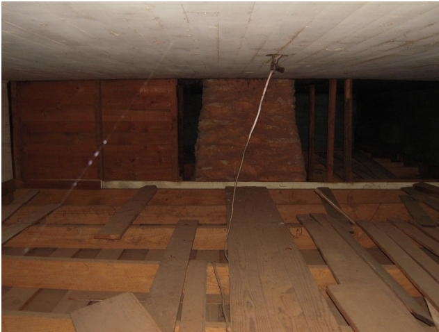
AD Figure 37: Lowered ceiling over Room 108
