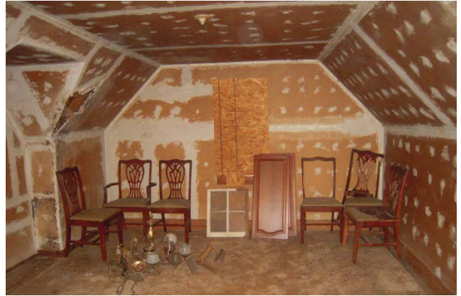
AD Figure 44: East view of Room 201 and unfinished walls
