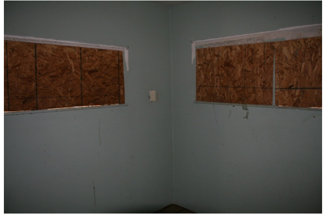
AD Figure 38: Southeast corner of Room 109
