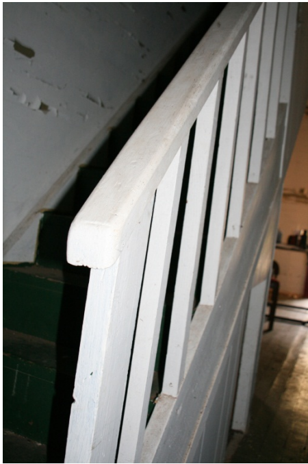
AD Figure 19: Stairs in Room 102
