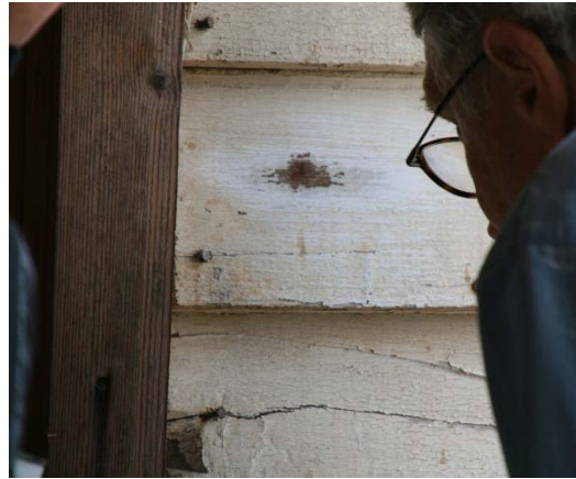
Exterior Siding outside of Room 111 on the west façade
