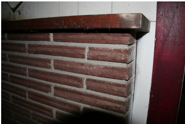
AD Figure 35: Faux Roman brick veneer and fireplace mantel in Room 108
