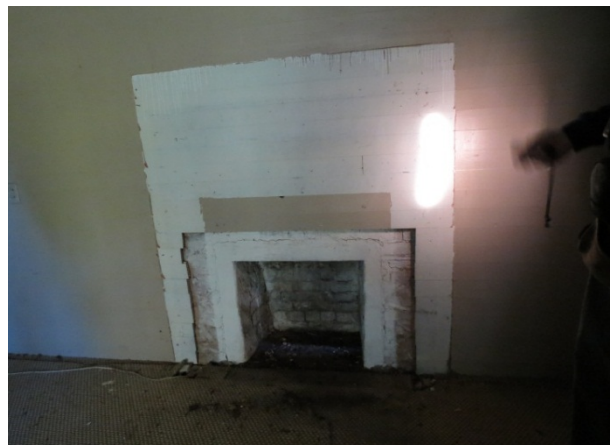
Mantel and surrounding wall
