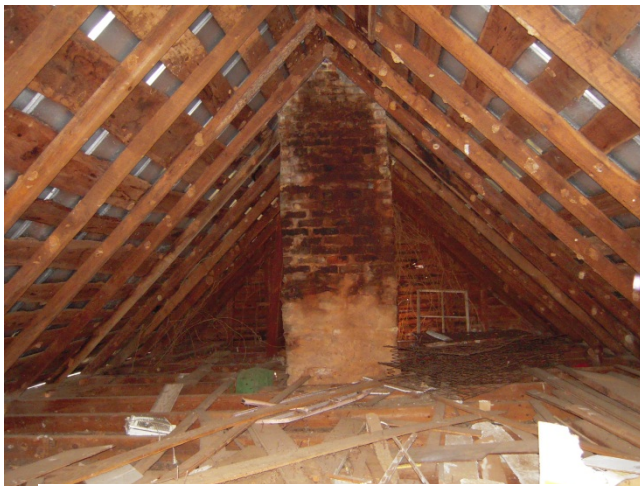
AD Figure 51: Attic space in Room 208
