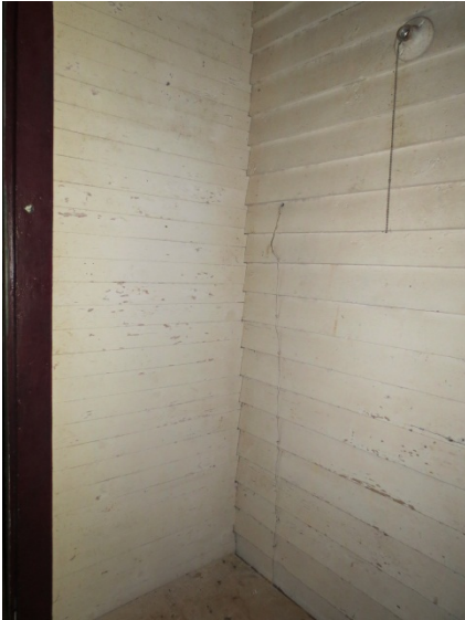
AD Figure 33: Exterior paneling outside of Rooms 108 and 109
