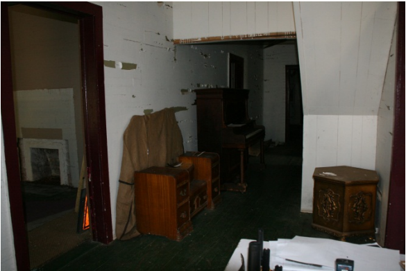
AD Figure 18: Room 102 looking southeast
