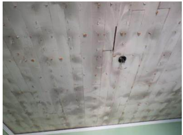
AD Figure 22: Acoustical Tile on ceiling in Room 103
