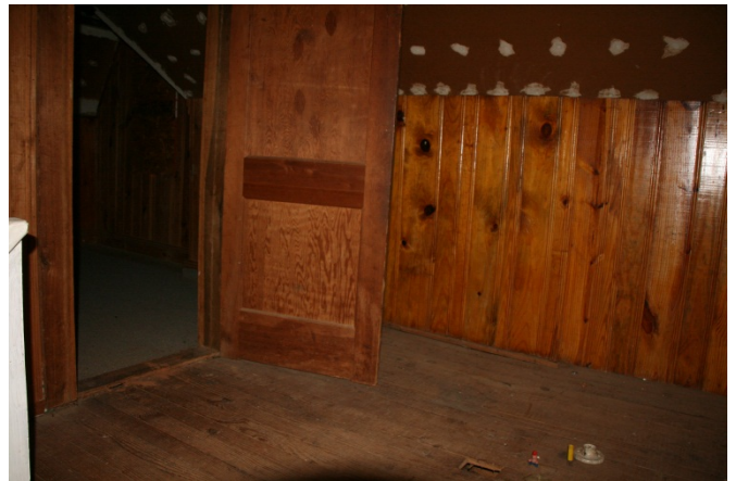
AD Figure 46: Room 202 looking west to Room 203, and half paneled walls
