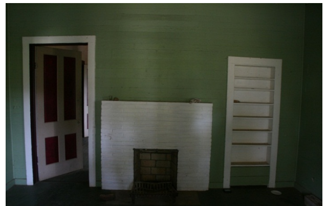
BC Figure 4: Room 103 and the faux Roman Brick veneer fireplace
