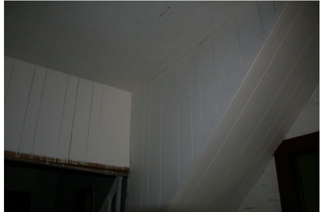
BC Figure 2: Paneled Partition in Room 102
