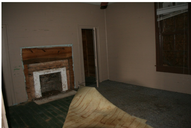
AD Figure 23: Northeast view of room 104 with fireplace and closet door
