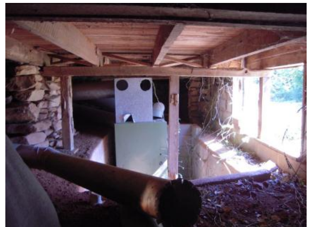
BC Figure 6: Furnace and cinder block pit were later additions ca. 1970-1980
