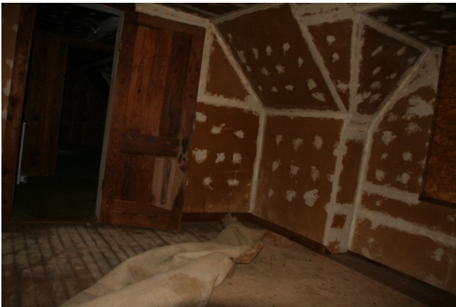
AD Figure 45: West view of Room 201 and Door leading to Room 202
