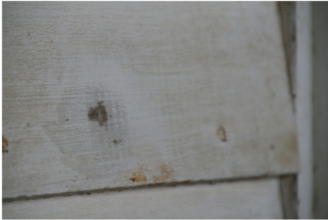
Exterior Siding outside of Room 108
