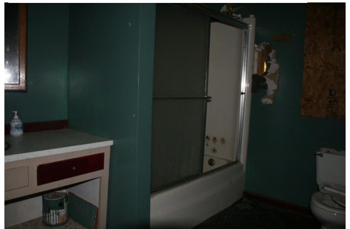
AD Figure 30: Room 106 looking northeast shower and toilet and sink
