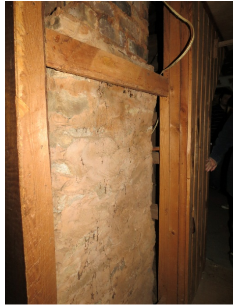
AD Figure 50: Exposed stuccoed chimney at the northwest of the house
