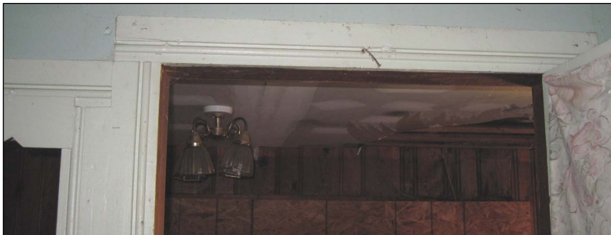
Window W-14 (left) and door D-16 (right) have similar casing profiles.
