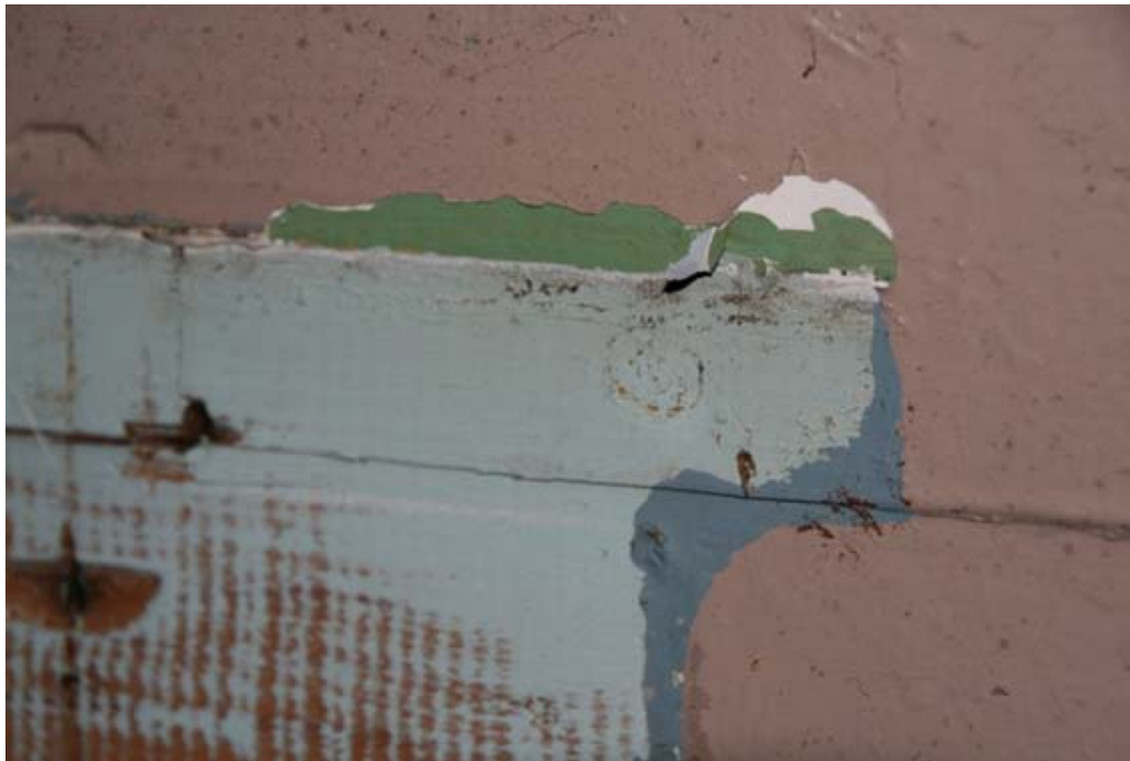
CA Figure 22: Room 104- Paint Analysis
