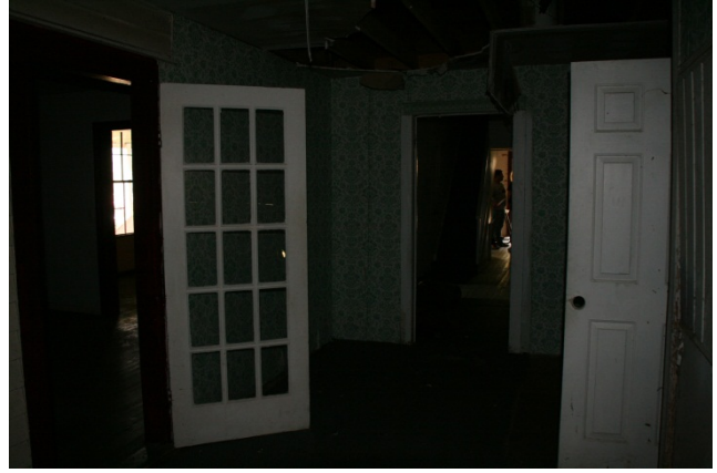
AD Figure 32: Room 107 looking north, Room 108 to the west
