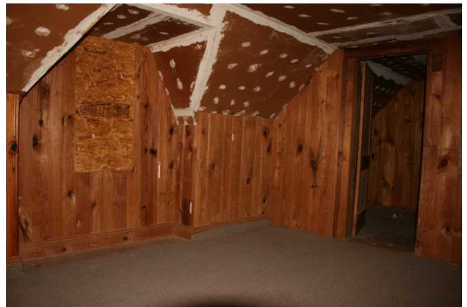
AD Figure 48: Southeast view of Room 203 and door leading to Room 202
