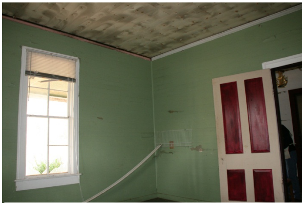
AD Figure 21: Northeast corner of Room 103
