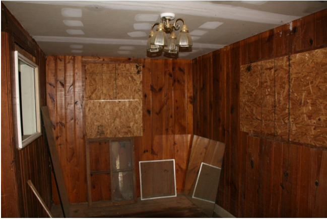
AD Figure 43: South view of Room 111
