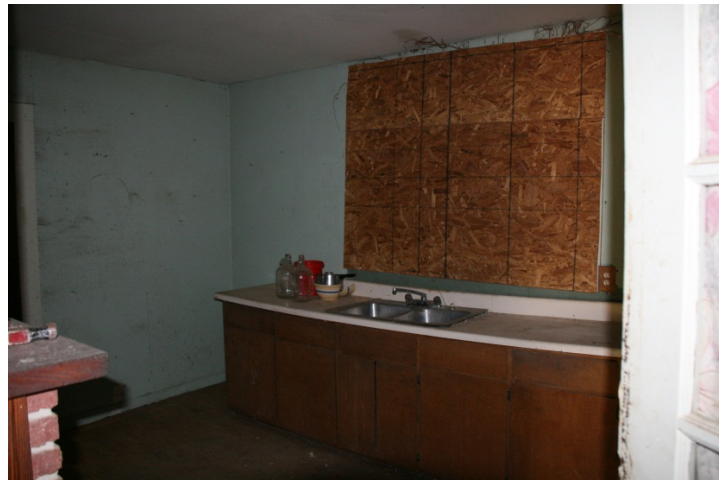
AD Figure 40: Southeast view of Room 110 and the kitchen sink
