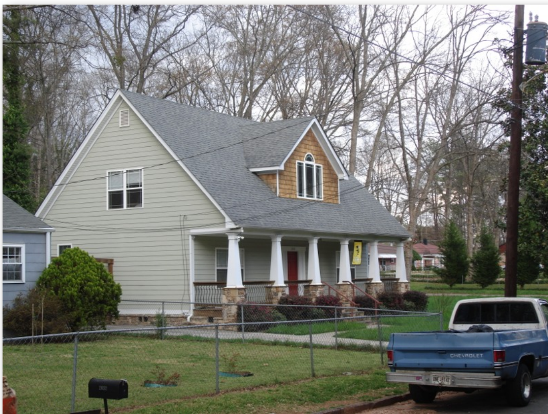
Image 153 Infill construction, Greystone Park subdivision
