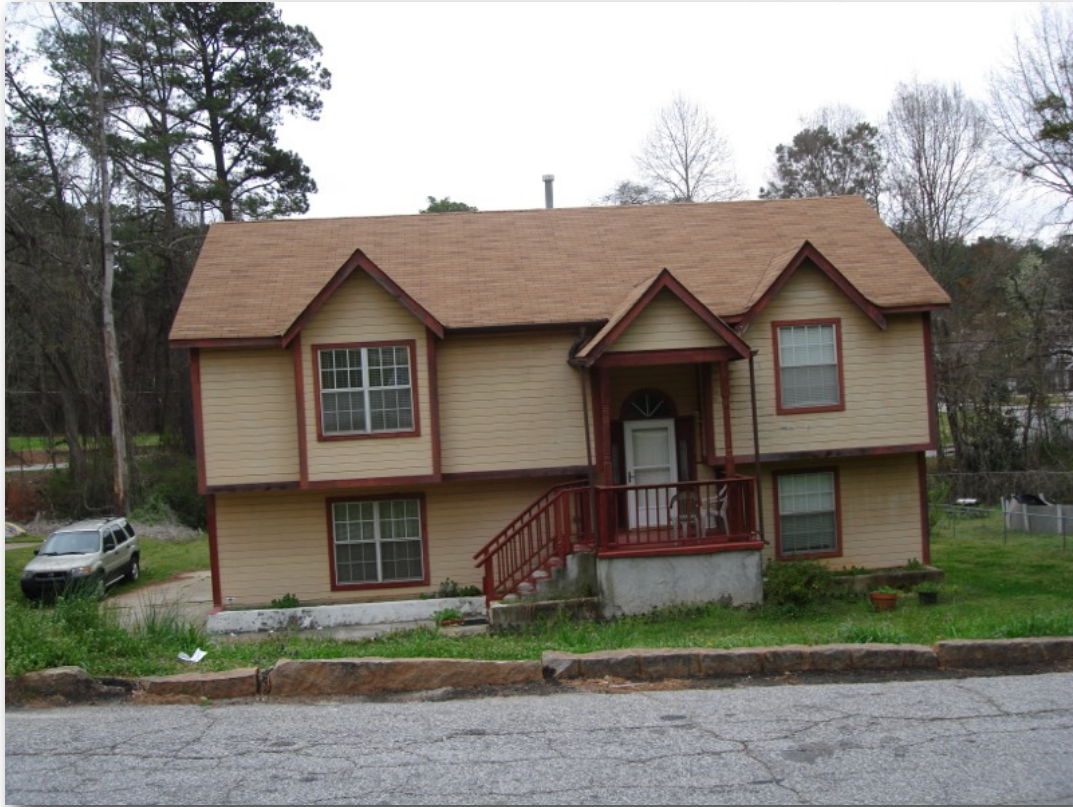
Image 144 Infill construction, Gresham Park subdivision
