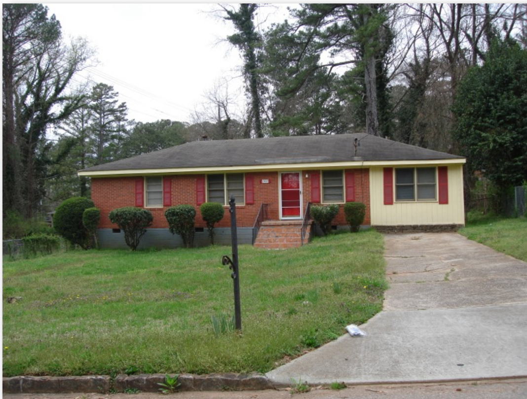
Image 142 Enclosed carport, Gresham Park subdivision
