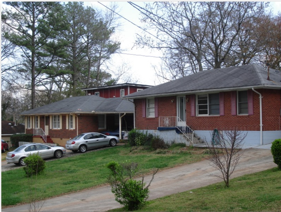
Image 152 Second floor addition, Greystone Park subdivision
