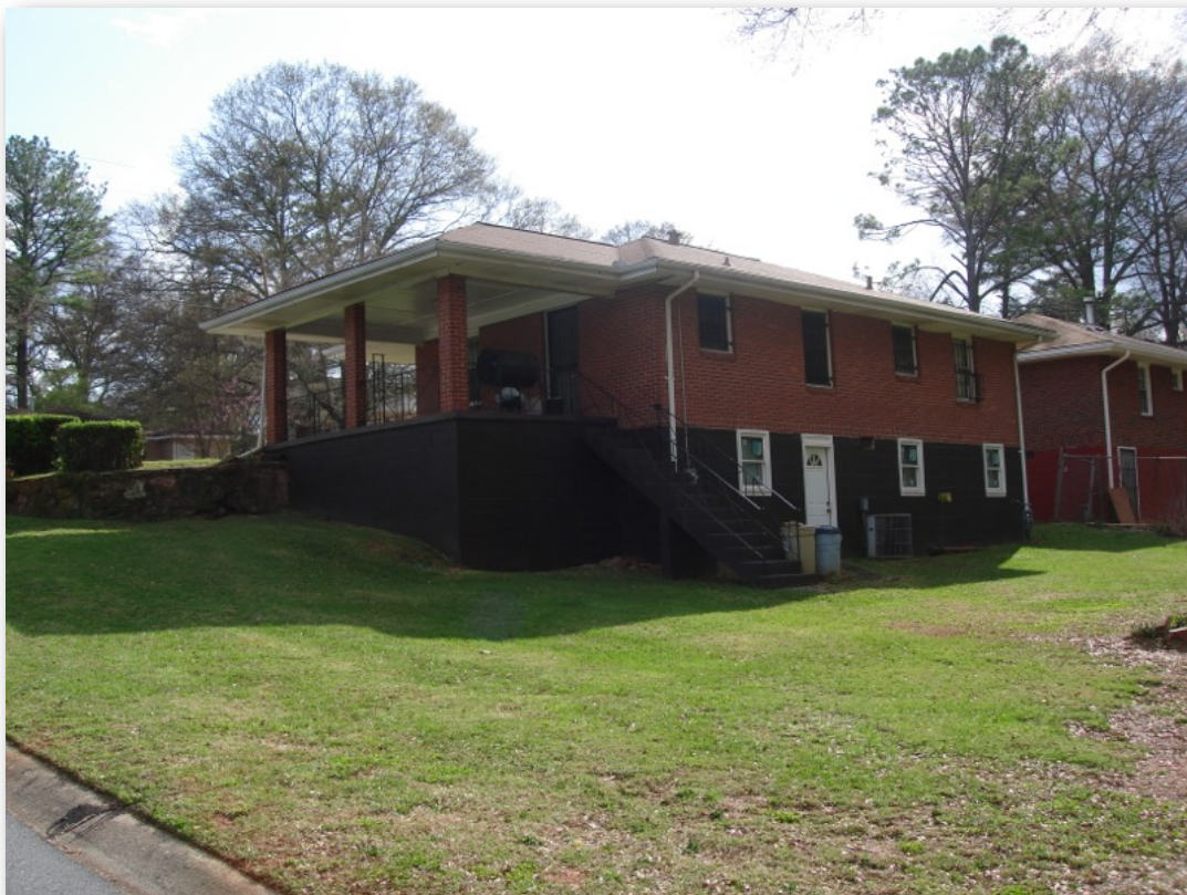
Image 149 Half basement, Greystone Park subdivision
