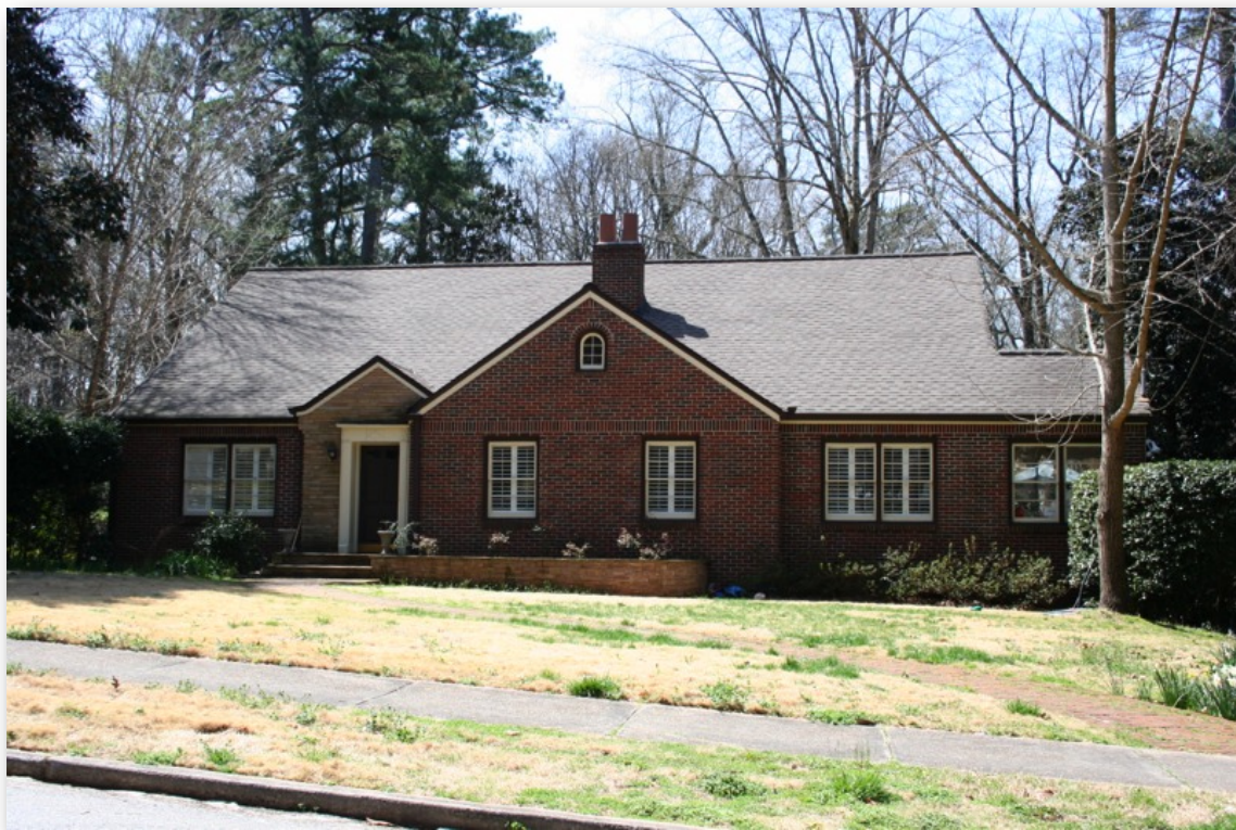
Image 97 "Red Brick Ranch," Parkwood subdivision
