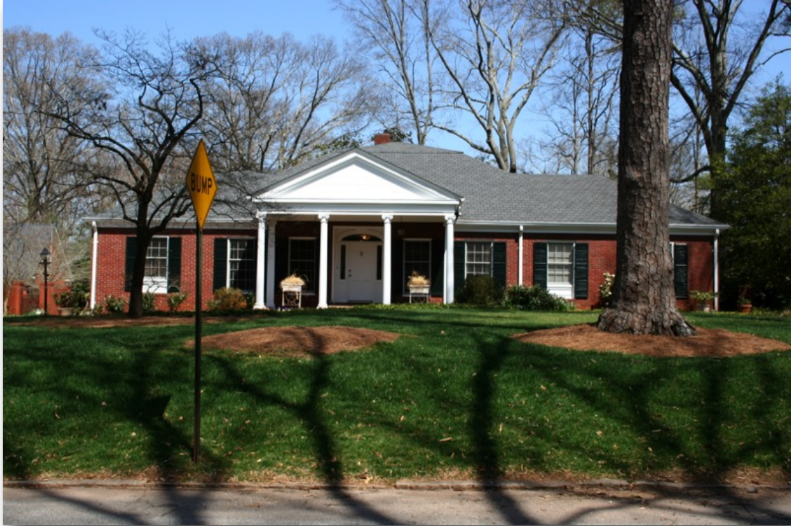
Image 176 Greek-revival style Ranch house, Parkwood subdivision
