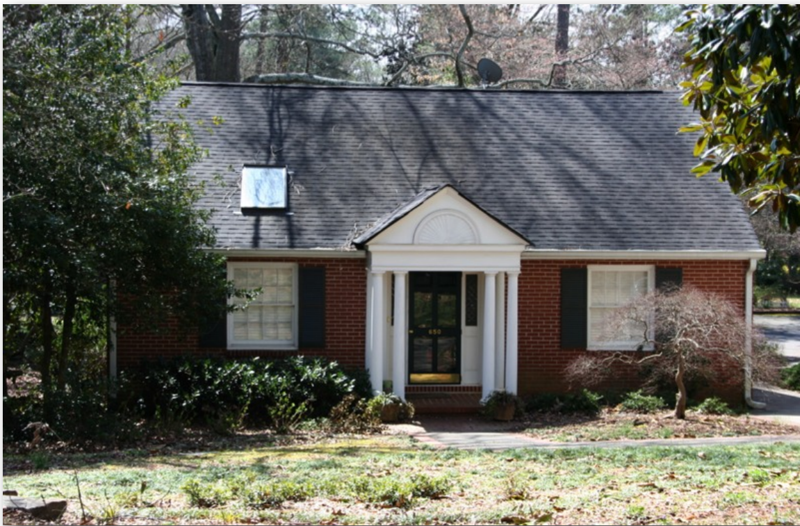
Image 171 American small house, Parkwood subdivision
