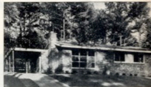
Front of house shows how well trees shade glass. Brick walls are insulated.
