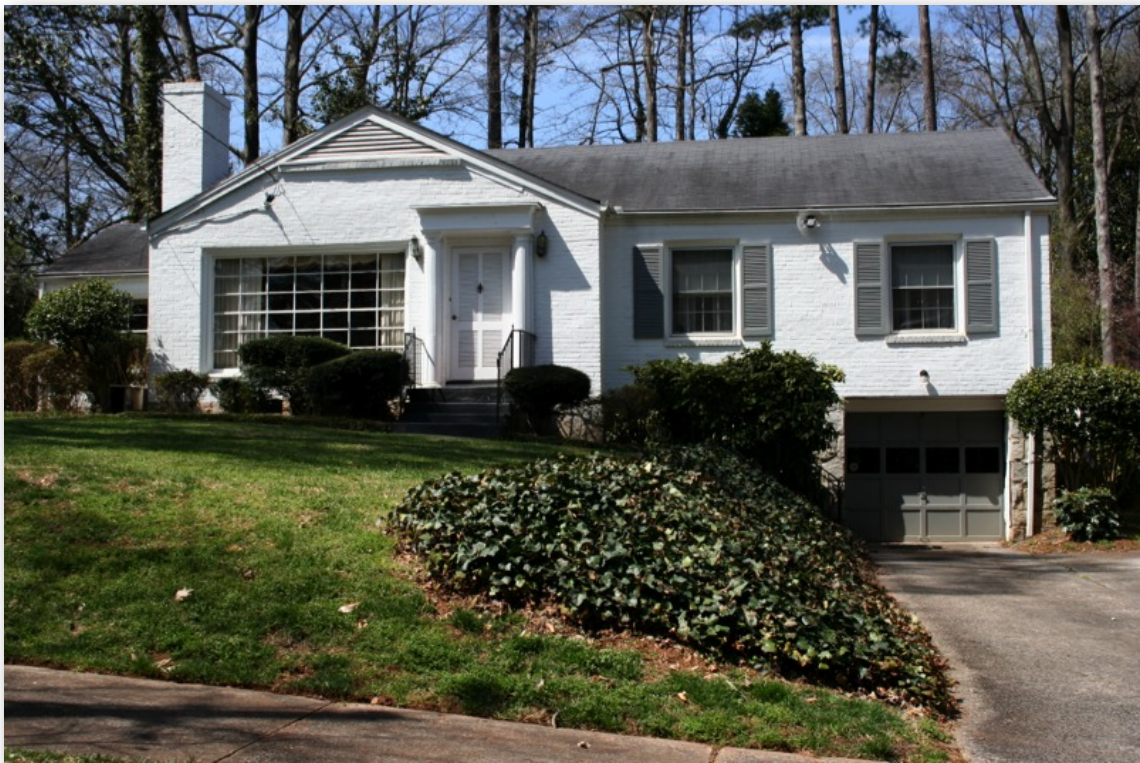
Image 181 Partial basement Ranch house, Parkwood subdivision
