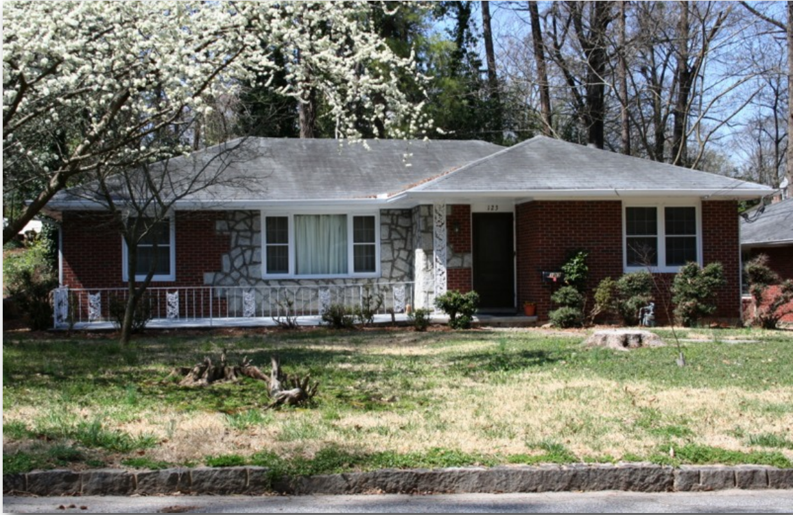
Image 98 Cast-iron columns and granite accent at entry
