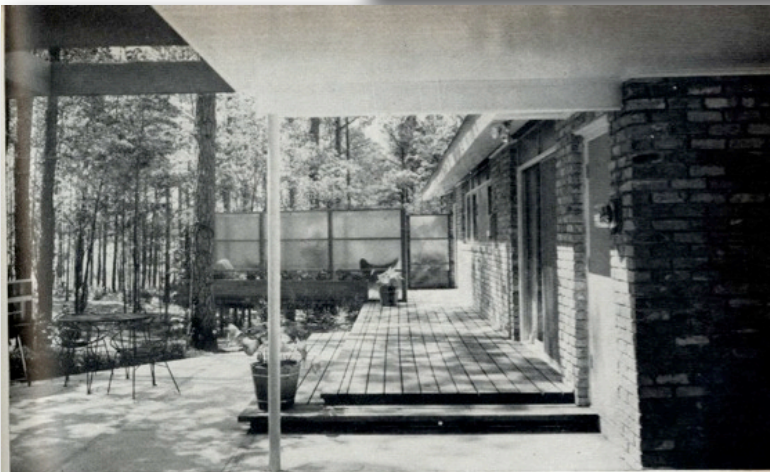
Rear of house has redwood deck, concrete terrace, and a plastic screen to give bedroom privacy. All this costs $900 extra.
