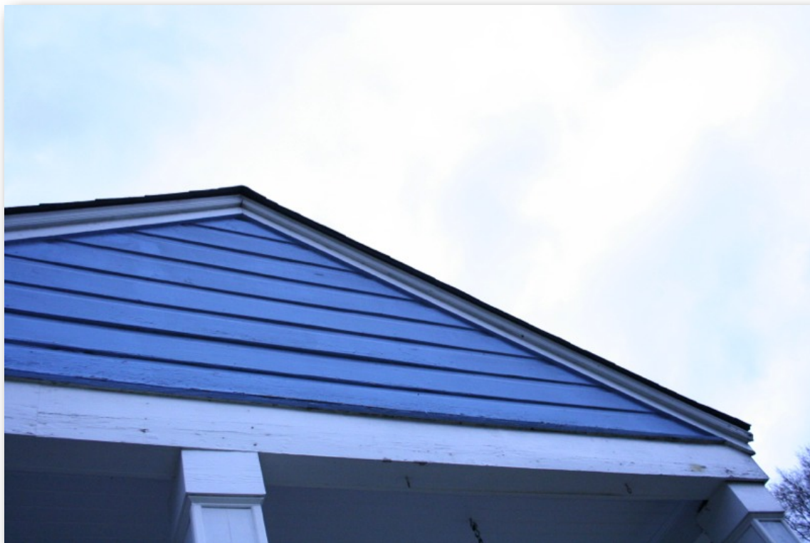
Image 73 Detail of eave on an American small house, Parkview subdivision
