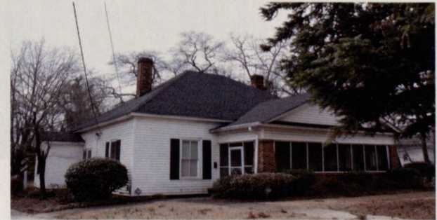
This house at 115 Bryan St. used transparent materials to create an appropriate porch enclosure that leaves the porch's historic materials clearly visible.
