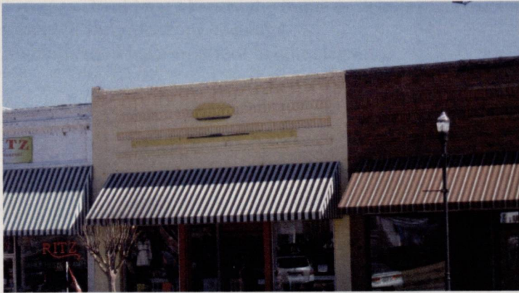
Characteristic flat roofs in McDonough
