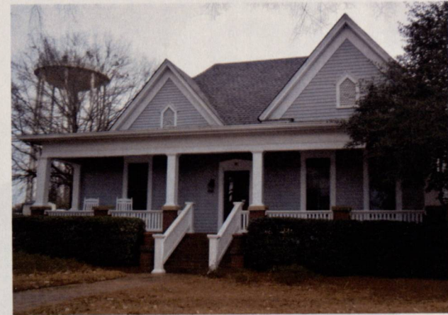
New South Cottage at 80 Macon St.
