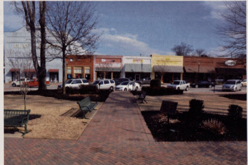
The herringbone brick pattern is used in the sidewalks of the square.
