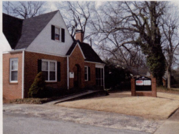
40 Jonesboro Rd., McDonough, Georgia Residential house now hosts office space
