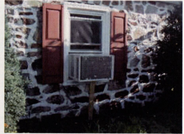
An air-conditioning unit like this one is inappropriate for a house's primary façade.
