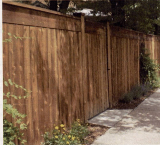
This fence is inappropriate because it is too tall and violates the 50:50 visibility ratio.
