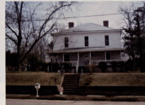
Georgian House at 212 Macon St.
