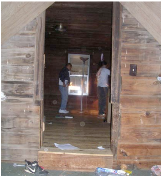
Fig. III-139. Unpainted exterior sheathing boards of the south wall, as shown from inside Room 206 looking north to Room 205.
