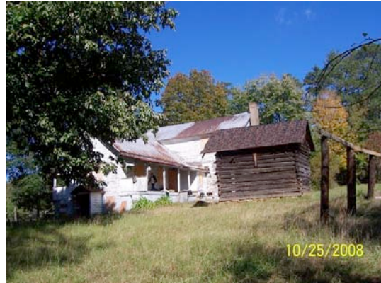
Fig. V-4. Lyon house and property. Outbuilding landscape site.
