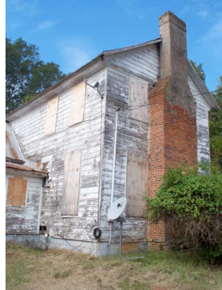
Fig. III-70. Intersection of the east and south façades of the main house.
