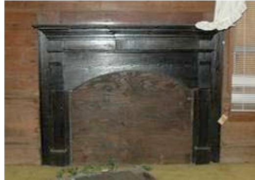
Fig. III-102. Fireplace on west wall, Room 105.
