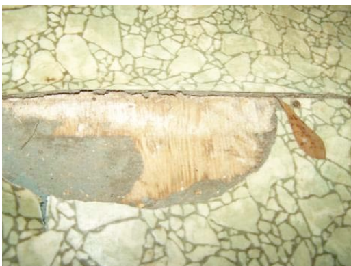
Fig. III-109. Room 106 plywood subfloor with rolled pebbled vinyl.
