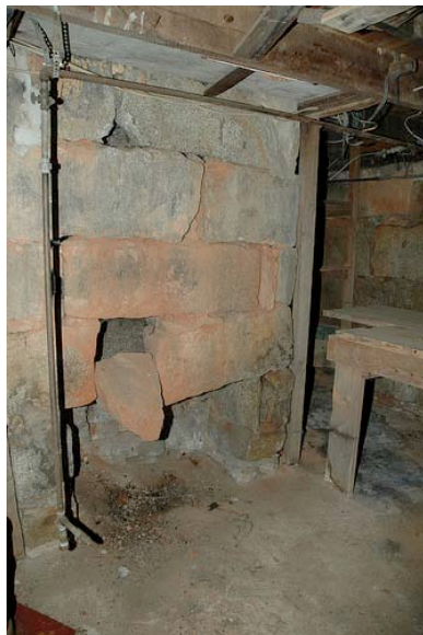
Fig. III-41. Looking north in Room 001 at the granite fireplace.
