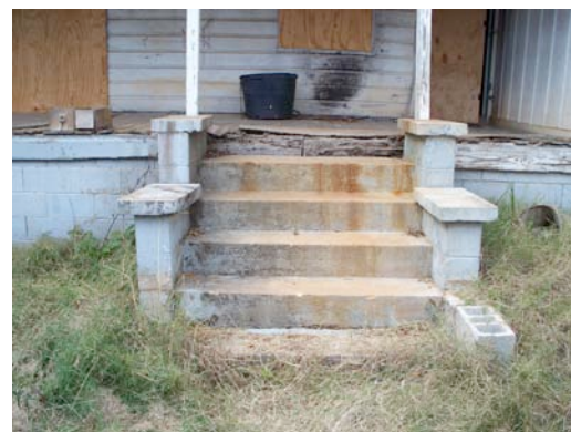
Fig. III-72. East porch steps.
