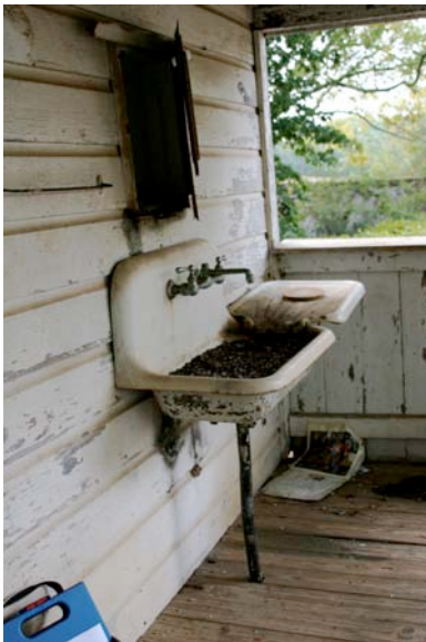
Fig. III-55. Sink on the west porch, south end of the porch.
