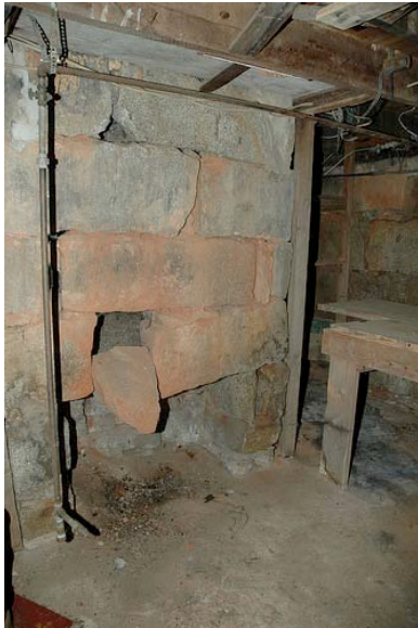
Fig. IV-26. Looking north in Room 001 at the granite fireplace.
