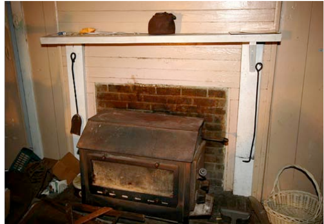
Fig. II-12. Room 106 south wall. Note: chimney also shared by Room 107.
