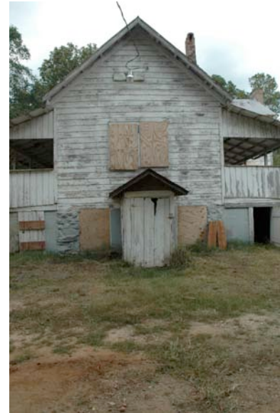
Fig. III-65. The south facade.
