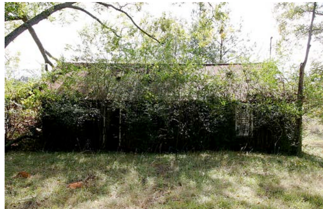
Fig. IV-10. North facade of the workshop. Notice the encroaching trees on the east façade.
