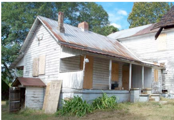
Fig. III-79. East and south facades. Rear ell has a rear-gabled roof with two interior chimneys. Shed roofs extend from just below the eaves to cover full-length porches on the east and west facades.
