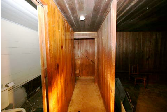
Fig. III-130 Room 201 (Hall) showing door frame at the far end of the hall.
