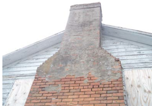
Fig. IV-54. Repair work at top of east façade chimney.
