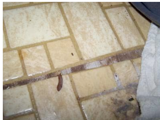
Fig. III-98. Room 104 (Laundry Room) Vinyl flooring.
