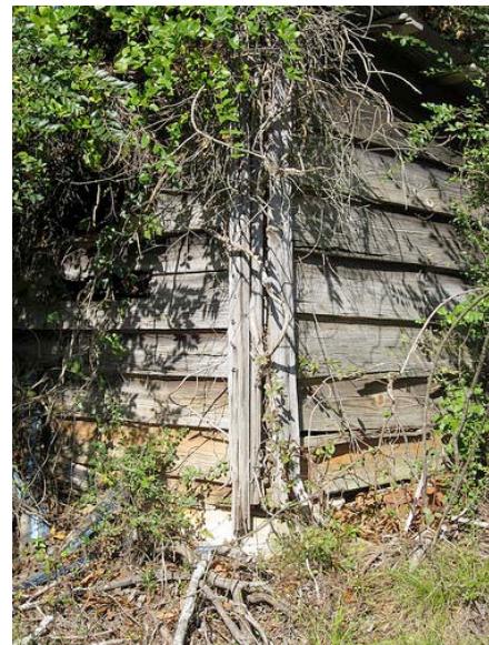
Fig. III-18. Northeast corner boards of the single pen.
