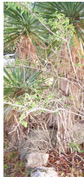
Fig. IV-4. Looking east. Overgrown vegetation in
