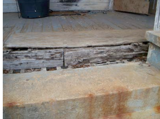
Fig. IV-56. Rust stains caused by runoff from metal roof.
