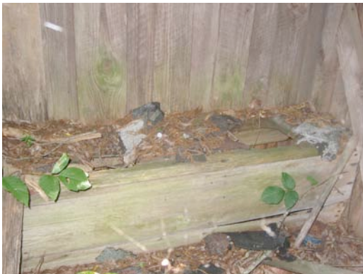
Fig. III-21. Interior of the privy, east wall.
