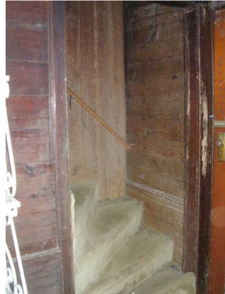
Fig. IV-73. Stairwell entrance to second floor.
