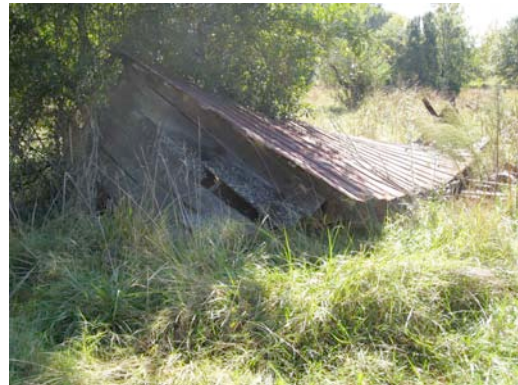
Fig. IV-14. Unknown structure located east of the Lyon House, which collapsed prior to the commencement of the HSR.
