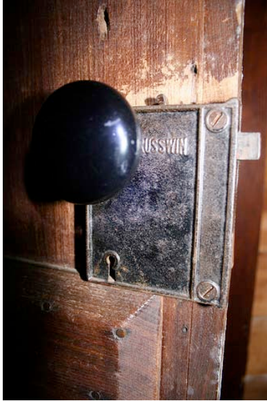
Fig. III-95. Hardware on door D6, note manufacturer name "Russwin".
