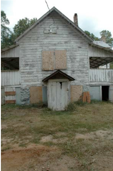
Fig. IV-46. The south façade of the rear ell.
