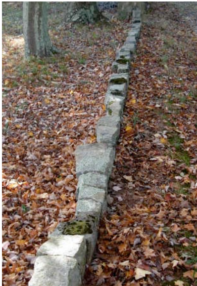
Fig. III-5. Retaining wall, looking west.
