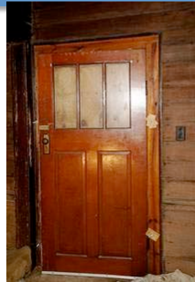
Fig III-88. Door D5, note varnished finish.
