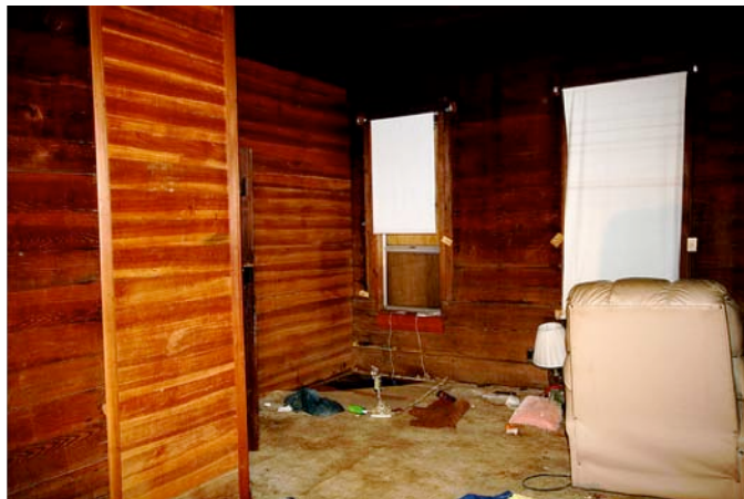
Fig. II-10. Room 102 (looking northwest). Note: closet wall added at a later date.
