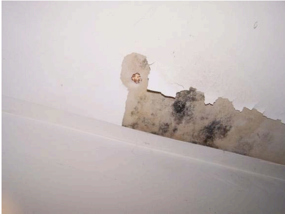
Fig. III-99. Room 104 (Laundry Room). Gypsum board walls.
