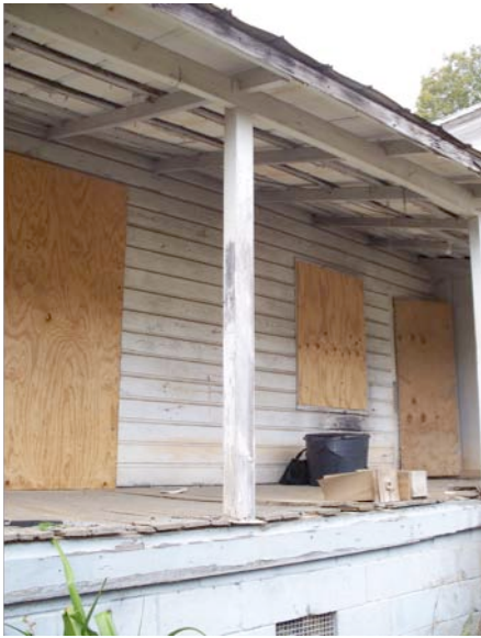
Fig. III-73. Detail of porch on east side of Lyon house.
