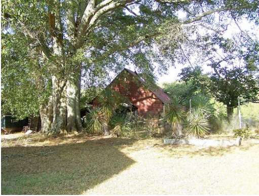
Fig. III-25. South façade of the barn—several pieces of clapboard siding are missing as well as elements from the roof.
