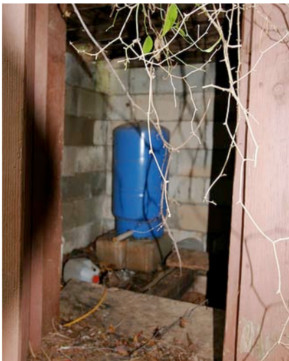
Fig. III-33: Interior of well house
