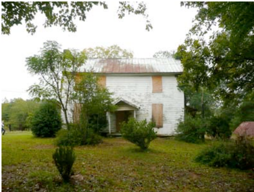
Fig. III-46. View of north façade, looking south.
