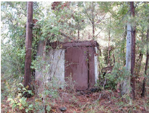
Fig. IV-19. Well structure surrounded by overgrown vegetation.
