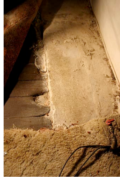
Fig. III-93. Granite hearth at fireplace, Room 102.
