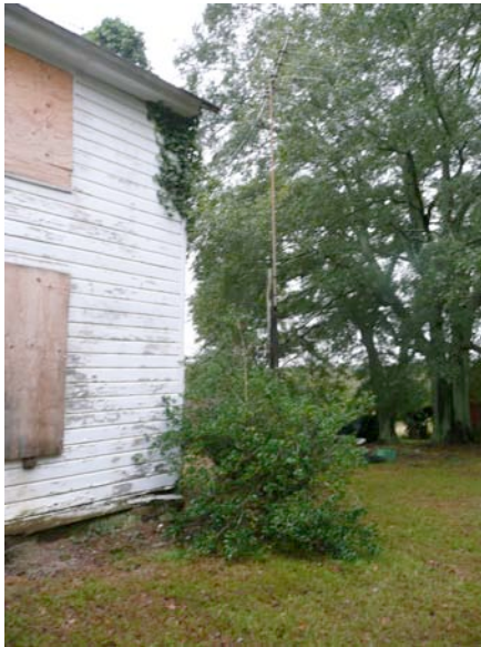
Figure IV-31 Northwest corner. Notice damage to boards above foundation, vines growing on wall, and overgrown shrub adjacent to house.
