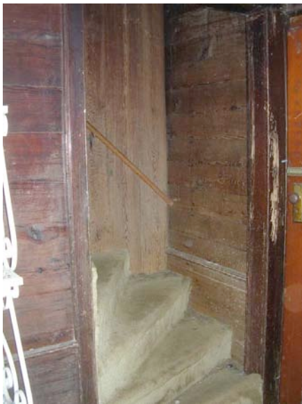
Fig. III-123 Stairwell entrance to second floor.
