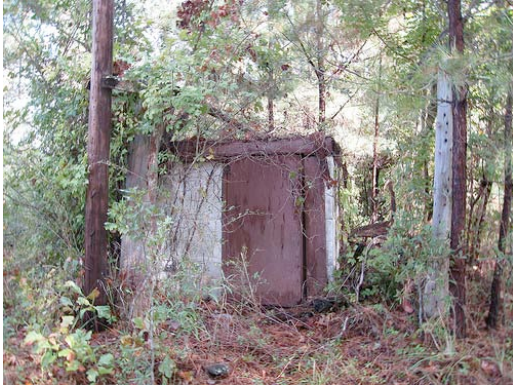
Fig. III-31. South facade of well house. Notice the wood post to the right—a post of the former structure covering the well hole.
