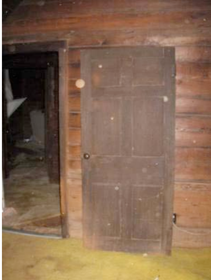
Fig. III-107. Mortise-and-tenon door, originally located between Rooms 105 and 101.
