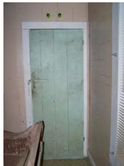
Fig. III-117. Door in attic was removed and placed in doorway between Room 106 and Room 107. Door hinges and hook match ghost marks and latch on doorframe.
