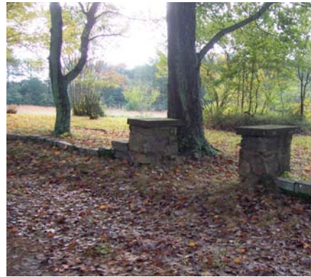
Fig. III-6. Cut granite columns with concrete copings. North side of property, viewed looking east.
