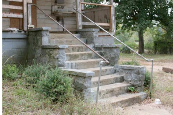
Fig. IV-37. Main stairs to the west porch.
