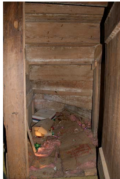
Fig. III-101. View of closet below stairs in Room 105 (door open).
