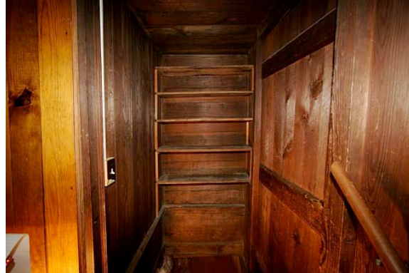
Fig. III-125 Built in case on south wall of second floor landing.
