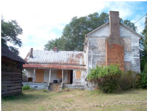
Fig. III-68. East facade of the Lyon house.
