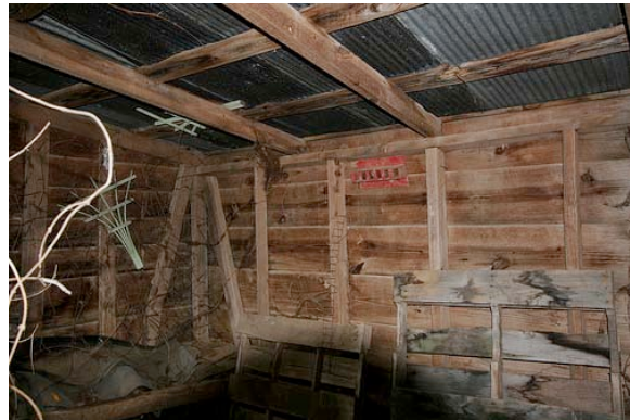
Fig. III-17. Interior of the single pen; notice the brace frame construction.
