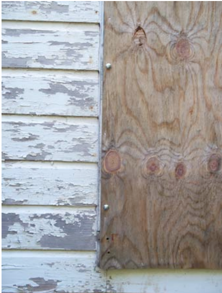
Fig. IV-51. Protective plywood panels that were mounted to window frames for security.
