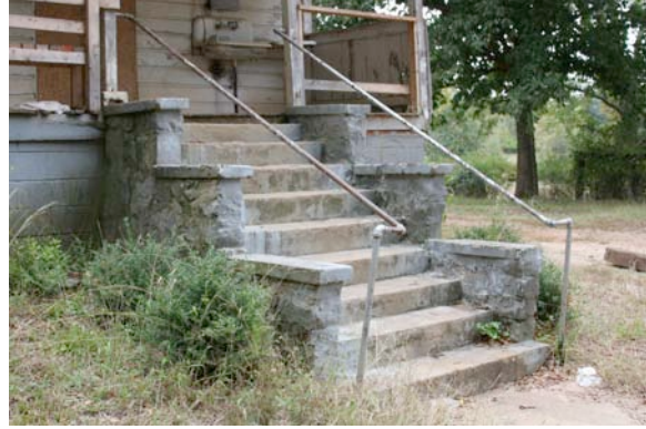
Fig. III-59. Main steps up to the west porch.
