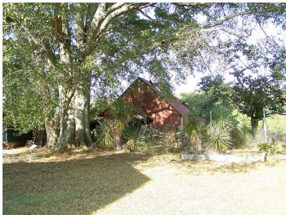
Fig. IV-15. Looking west from the Lyon House, the east façade of the barn is visible.
