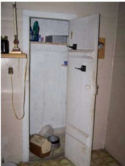
Fig. III-120. Room 107. Board-and-batten door (D15)
