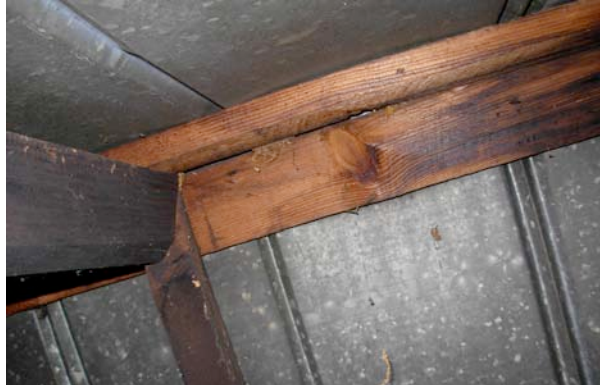
Fig. III-81. Attic (Room 207). Ridge purlins where rafters connect at ridgeline.
