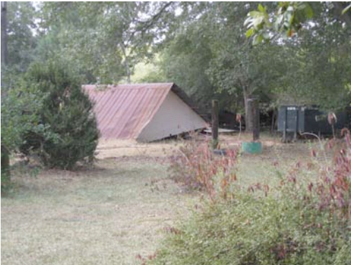
Fig. III-26. Looking southwest from the Lyon house. The collapsed garage is visible (center).
