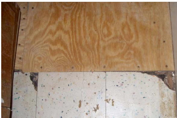
Fig. III-97. Vinyl tile and plywood subfloor, Room 103.
