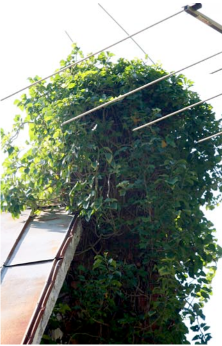
Fig. IV-33. Top of the west chimney, note the television antenna.
