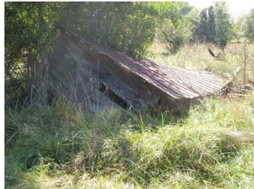
Fig. III-23. Unknown structure, to the east of the Lyon House that has collapsed.
