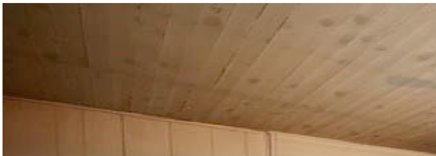
Fig. III-111 Room 106 ceiling boards running north to south.
