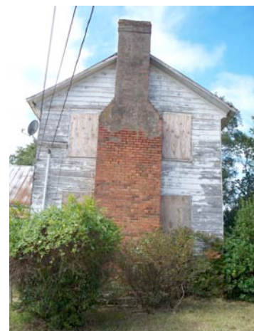
Fig. III-69. The east façade of the two-story portion of the Lyon house.
