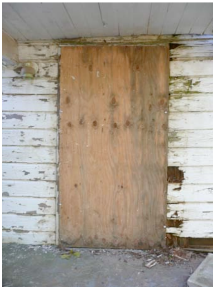
Figure IV-28 Door (D5) covered with plywood.
