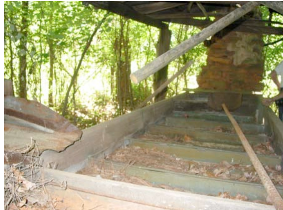
Fig. IV-21 Copper evaporator prior to it being stolen. Notice the portland cement patches visible on the chimney.
