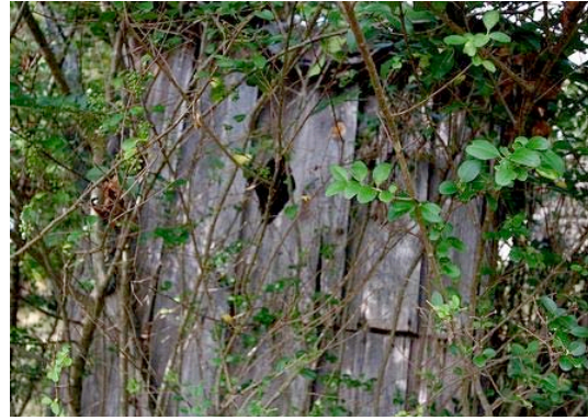
Fig. III-22. Close up of diamond cut window on north façade of privy.
