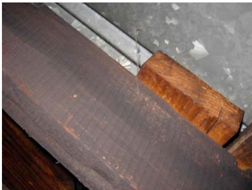
Fig. III-80. Attic (Room 207). Circular saw marks on rafters in rear ell roof.
