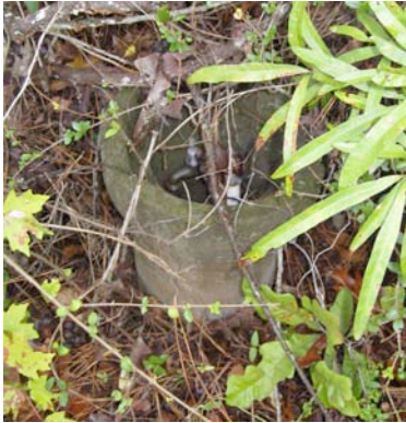
Fig. III-32. Faucet surrounded by cement located west of the well structure.
