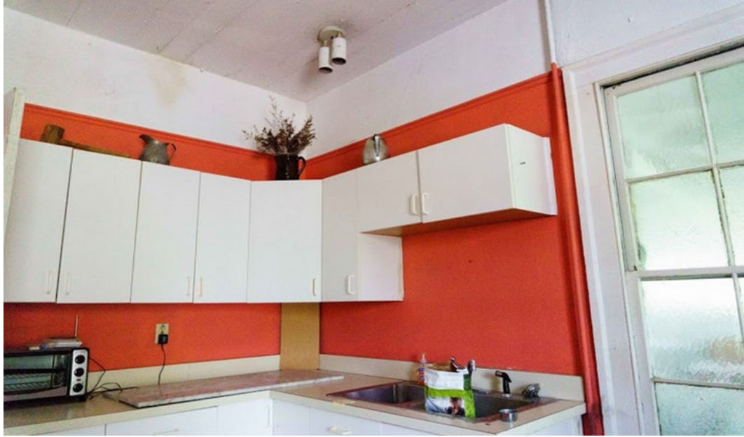
Figure 47. Room 203 facing southwest.
