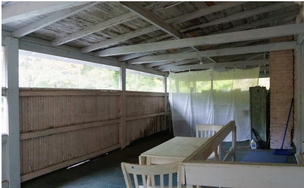
Figure 57. Room 207 facing northwest.
