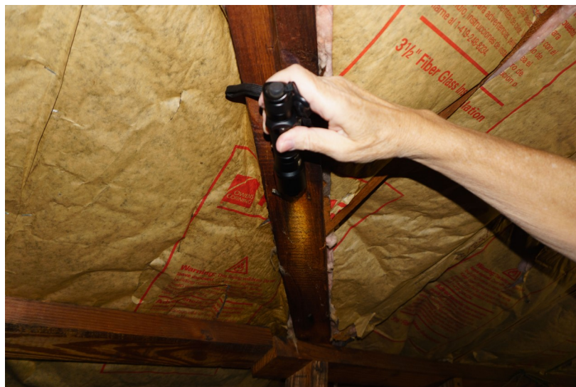
Fig 66 Attic: Historic wood beams with dense graining.
