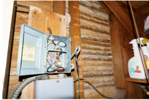
Figure 29. Closet underneath stairs in Room 105.
