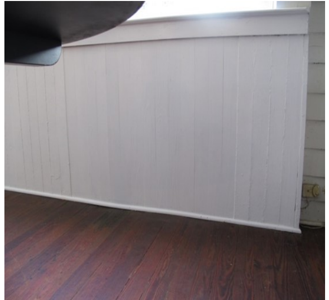
Figure 87. Repair made on the west wall.
