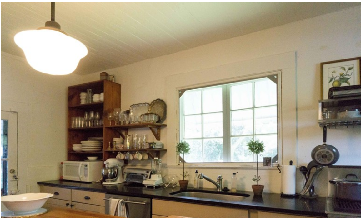
Figure 40. Room 107 facing west.
