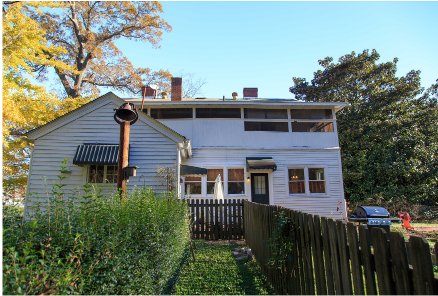
Figure 16. This view of the west side of the Avary-Fulton house shows the numerous features visible along the roof.
