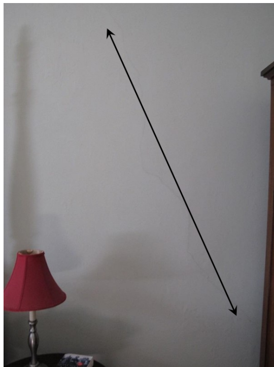
Figure 79. Room 102. North of the window on the west wall.
