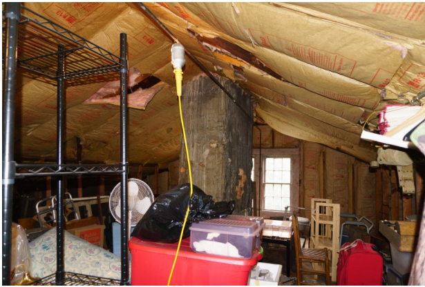
Figure 62 Attic: use as storage space
