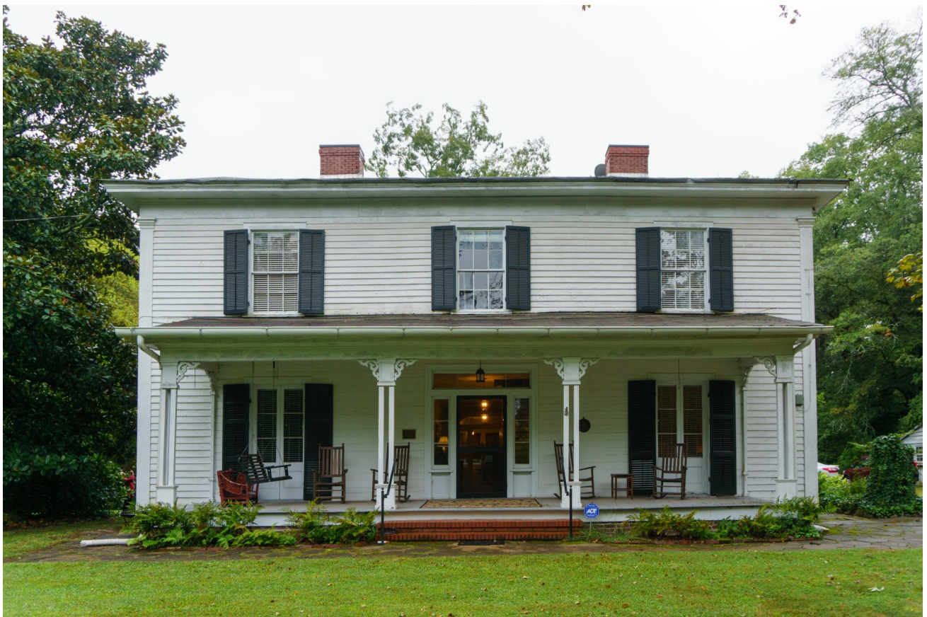
Figure 15. The side-gabled roof of the main house and shed roof above the front porch.
