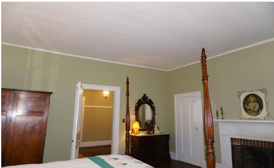
Figure 25. Room 102 facing north.
