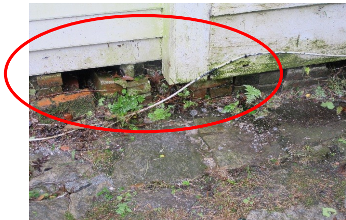
Figure 70. Open space in foundation.
