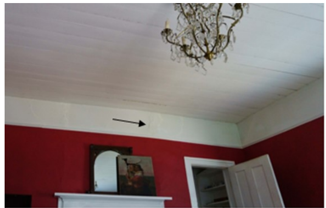
Figure 133 Room 204 facing west.
