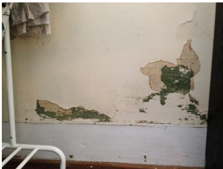
Figure 125: Room 201 facing south.
