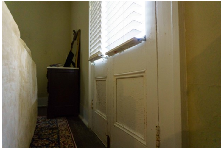
Figure 124: Room 104 facing northeast.
