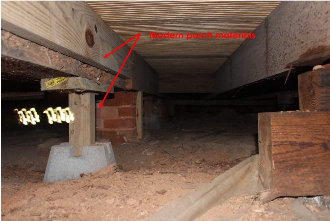
Figure 8. Modern foundational elements.
