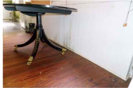
Figure 34 Room 106 wainscot west wall.
