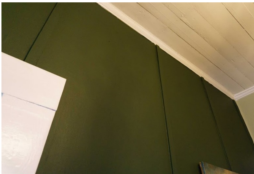
Figure 52 West wall of Room 205.
