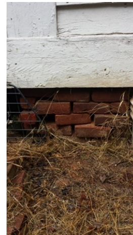
Figure 101: South façade foundational brick pier recommended repointing
