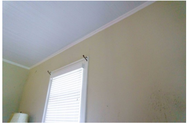
Figure 123: Room 104 facing north.
