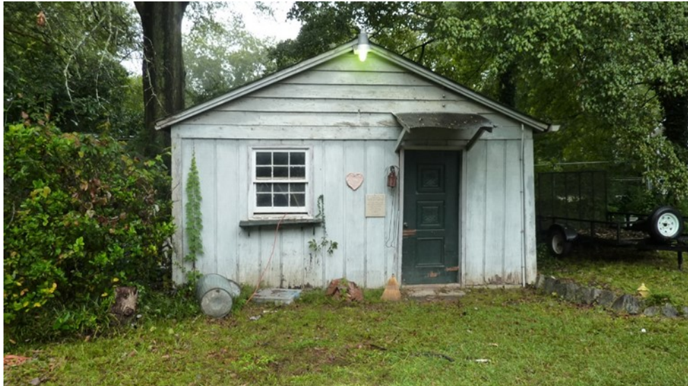
Figure 4. The Avary-Fulton House outbuilding
