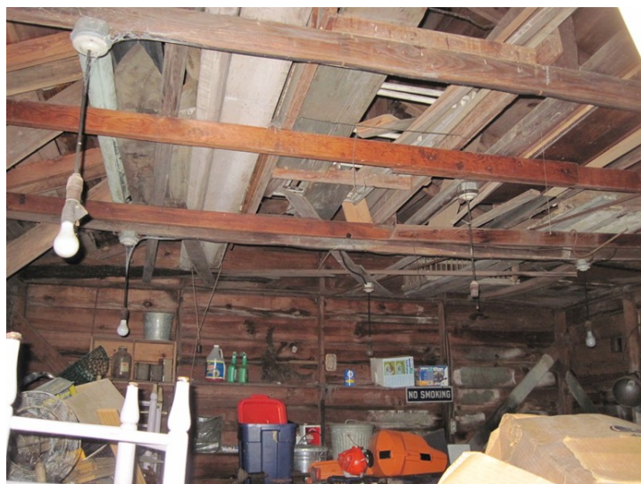
Figure 4a. The outbuilding's interior, now used for storage, reveals the wood platform frame construction. Photo by Laura Drummond
