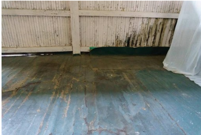
Figure 136 Room 206 facing west
