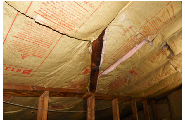
Figure 63 Attic: Remnant of hipped roof-
