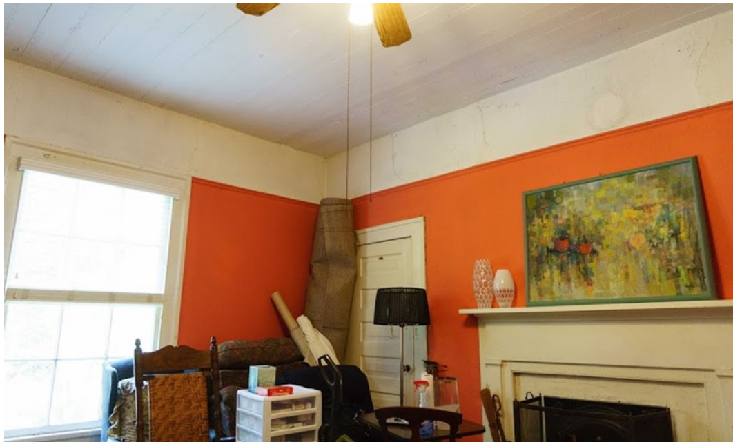
Figure 48. Room 203 facing northeast.
