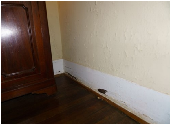
Fig120: Room 103 facing north.
