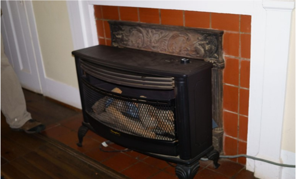
Figure 27. Fireplace in Room 103.
