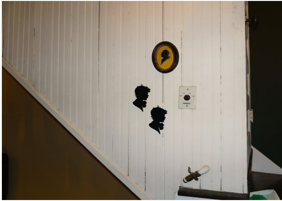
Figure 53. Room 205 enclosed attic stairs. Notice the beadboard siding, switch for the house fan and gas hook-up.
