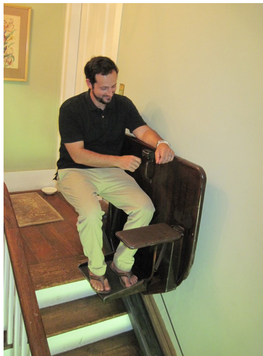
Figure 61. Resident Rob Sway demonstrates the Inclinator's operation. (Photo by L. Drummond)
