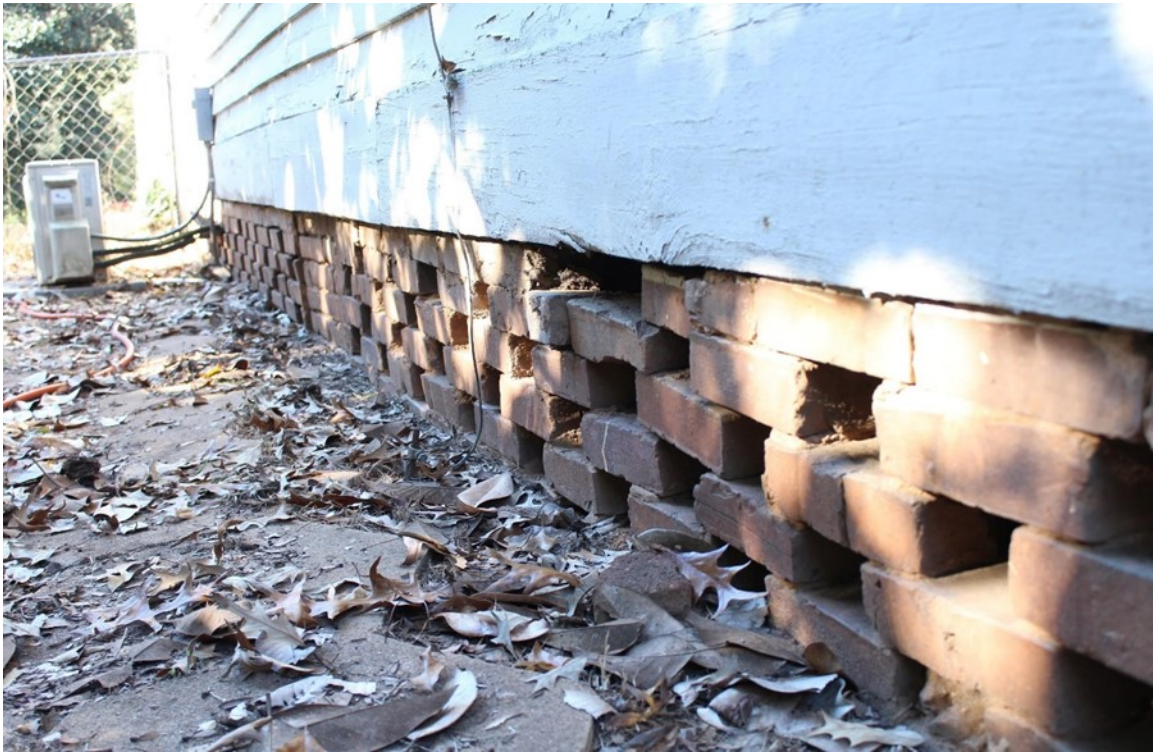
Figure 12. Foundation brick latticework.
