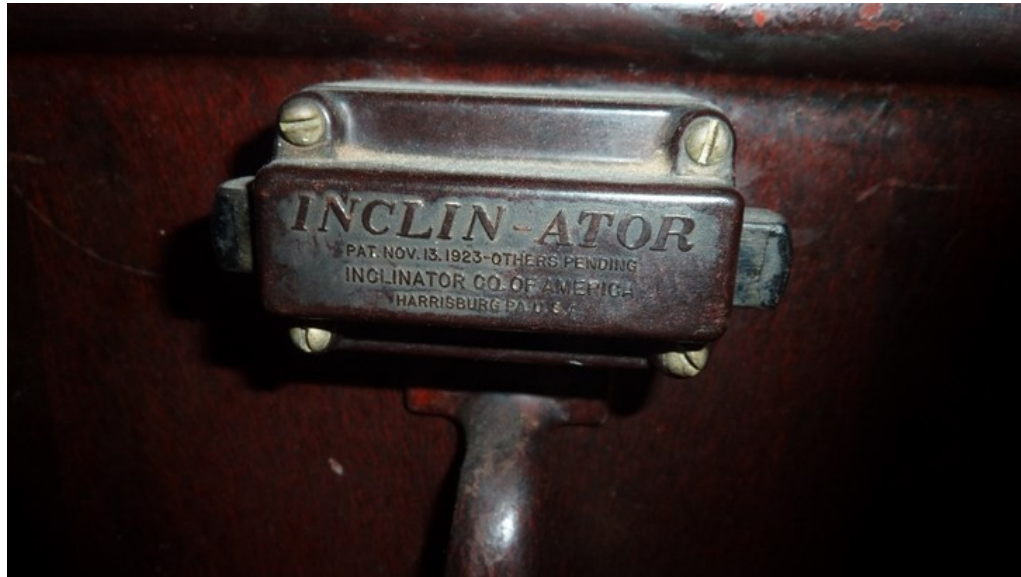
Figure 60. Inclinator fixture with patent date.
