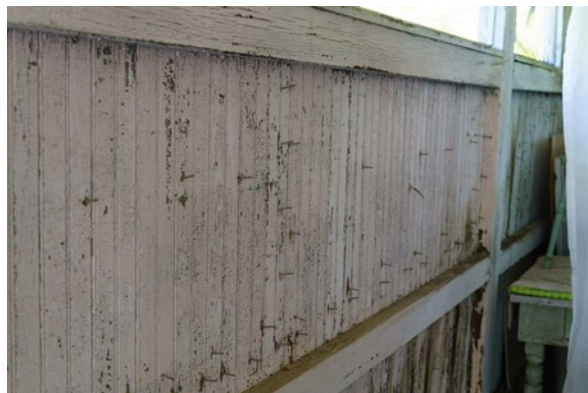
Fig 137: Room 206 facing northwest
