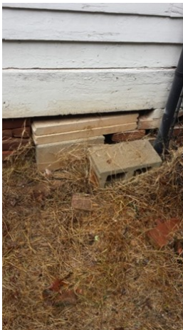
Figure 100: South façade with concrete supporting brick pier.
