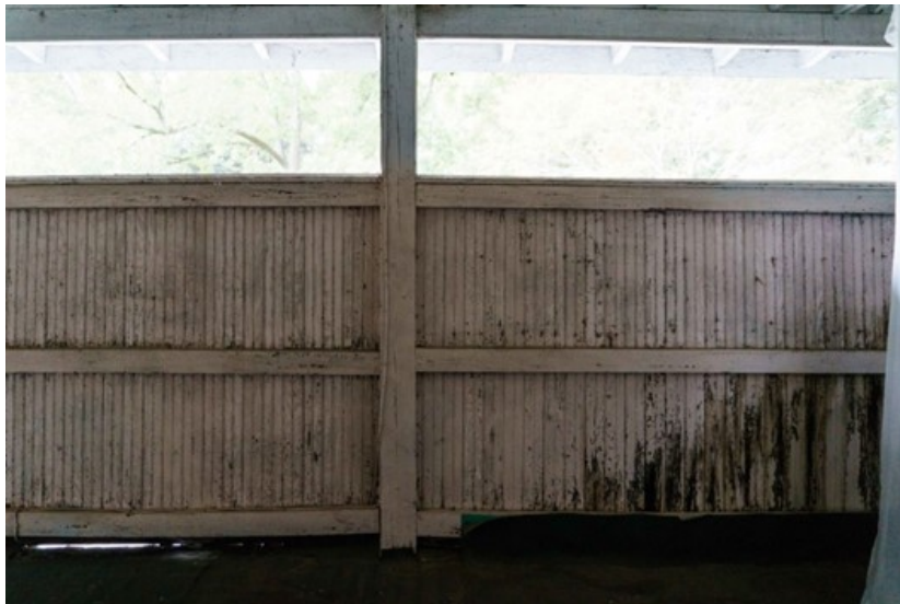
Figure 127: Room 206 facing west.
