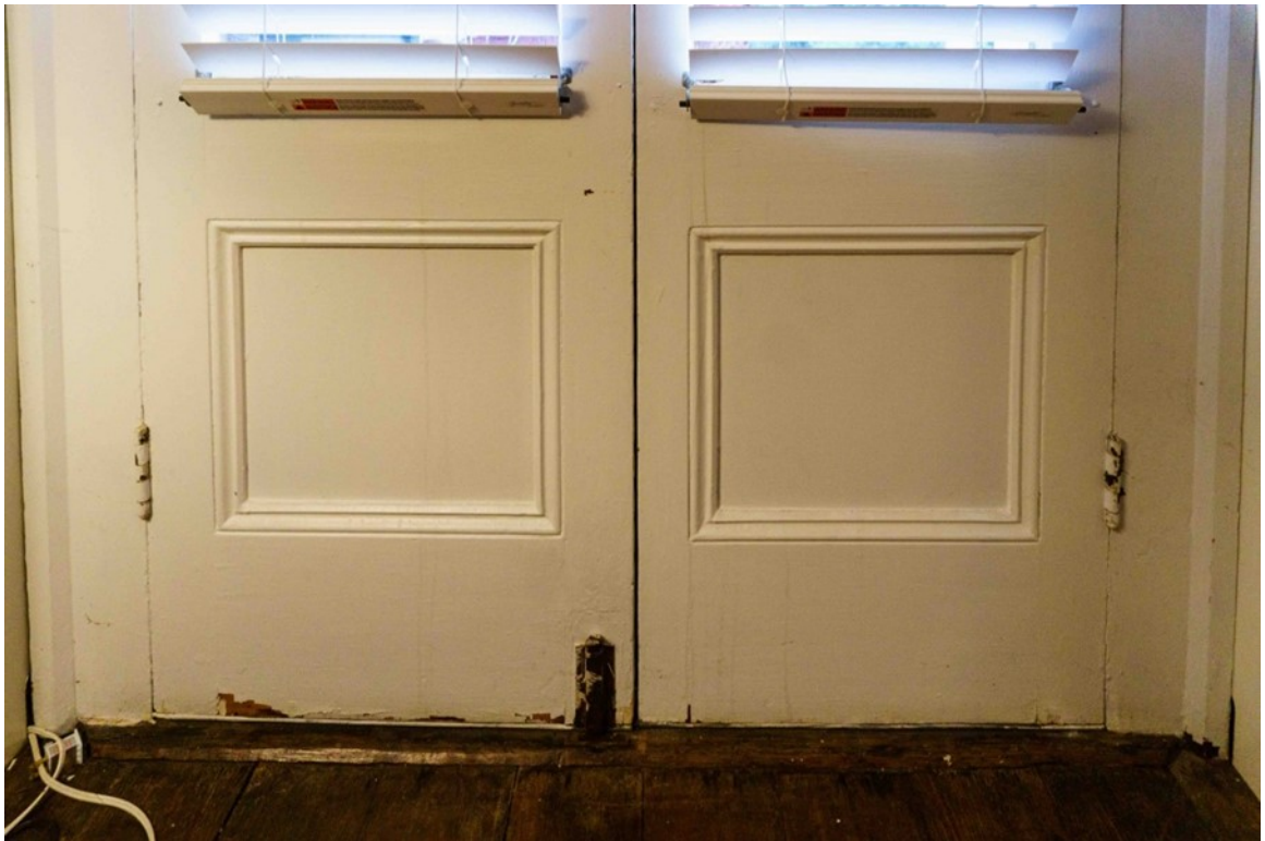
Figure 77 Room 101. Base of the double doors.
