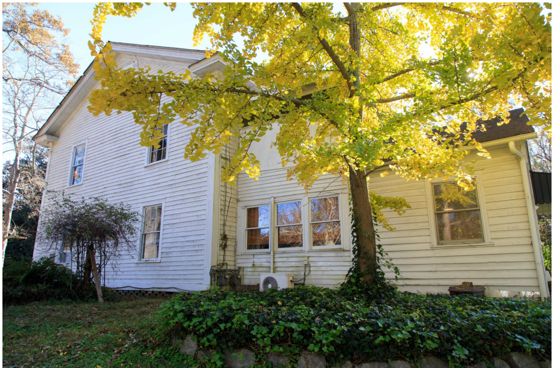
Figure 21. North Façade, main house view.
