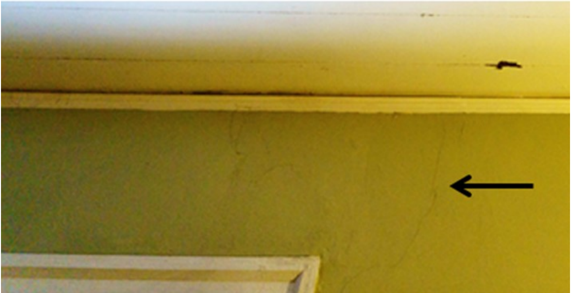
Figure 78. Room 102. Upper right corner of the south window.
