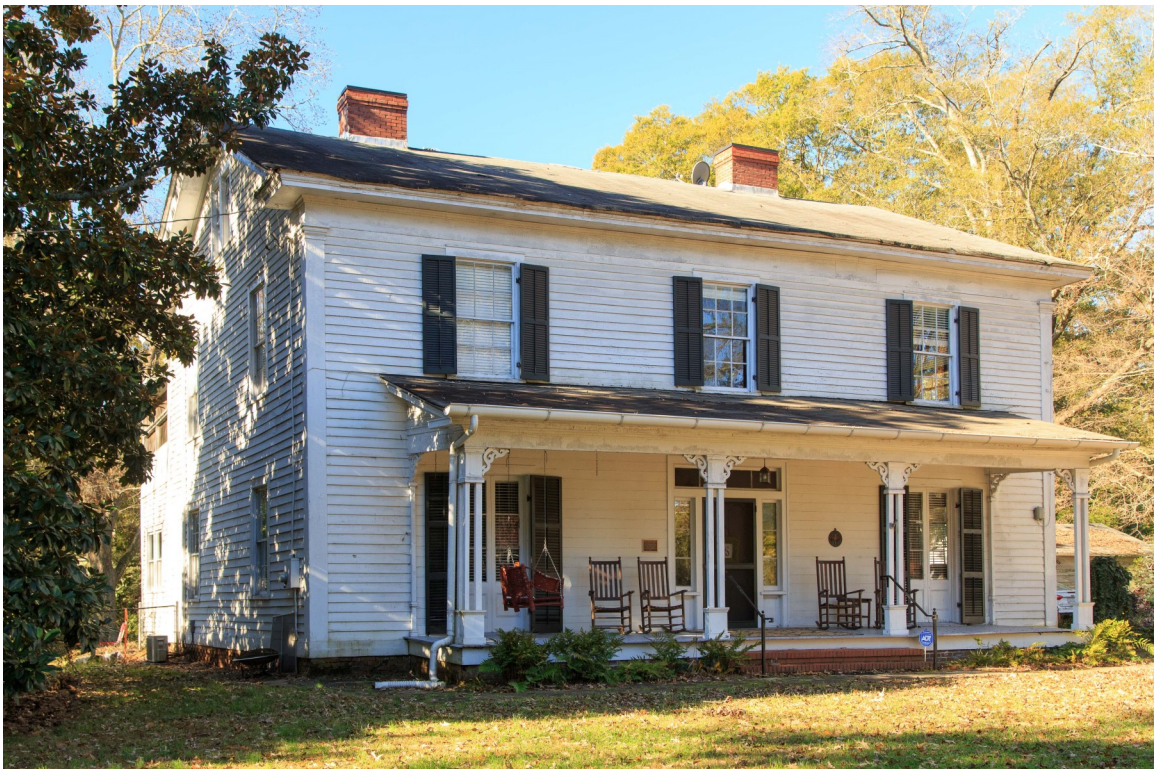
Figure 18. East Façade with view of south facade.
