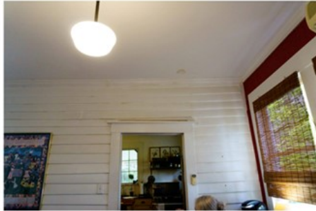
Figure 33. Room 106 facing west.
