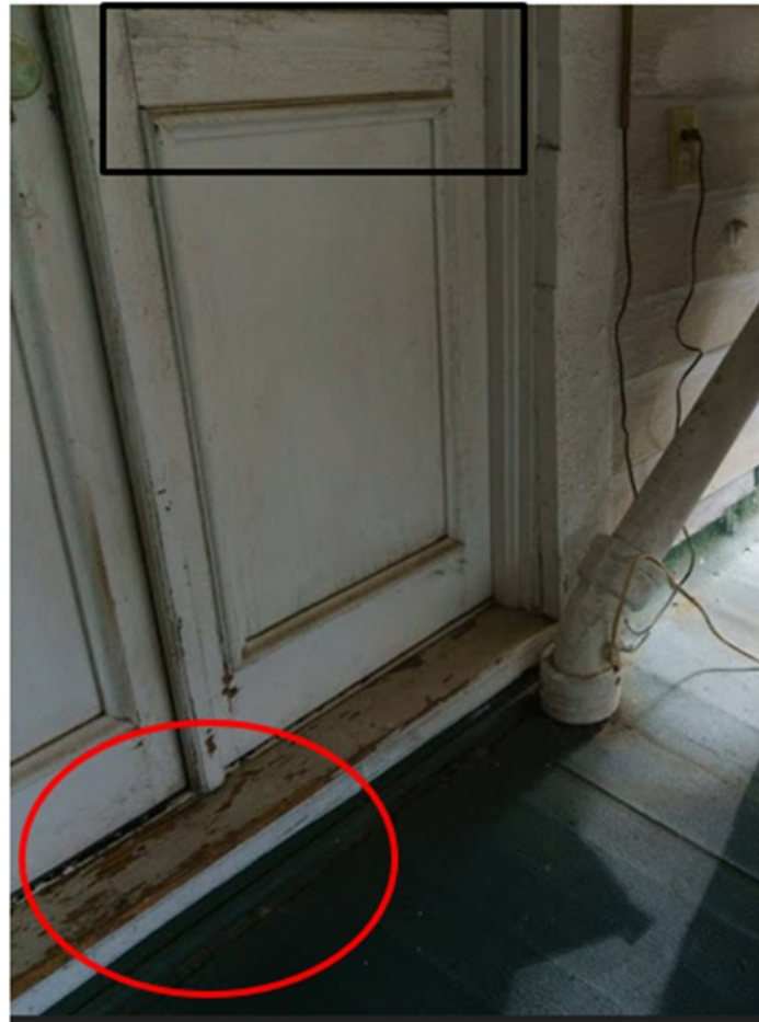
Figure 98. The double doors on the east wall of Room 206. The red circle highlights the paint alligating and the circle shows where the paint is wearing away.
