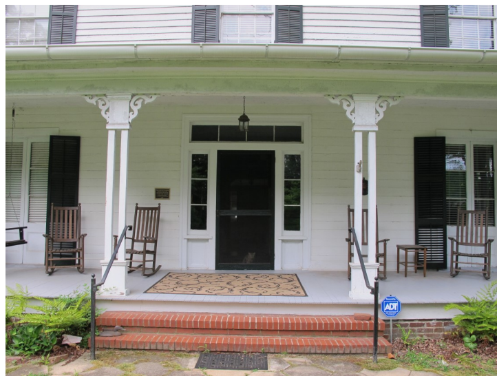
Figure 6 Greek Revival four-over-three lights surrounding front door & flush plank siding under porch roof; folk Victorian ornamental brackets topping porch columns
