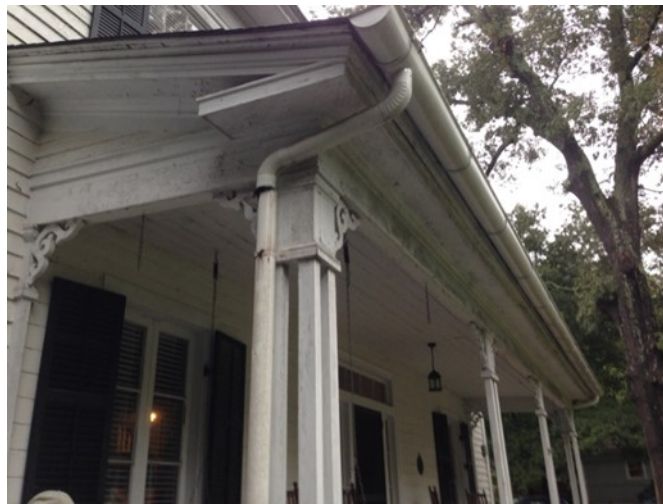
Figure 112. East Façade on the southeast corner downspout and gutter system
