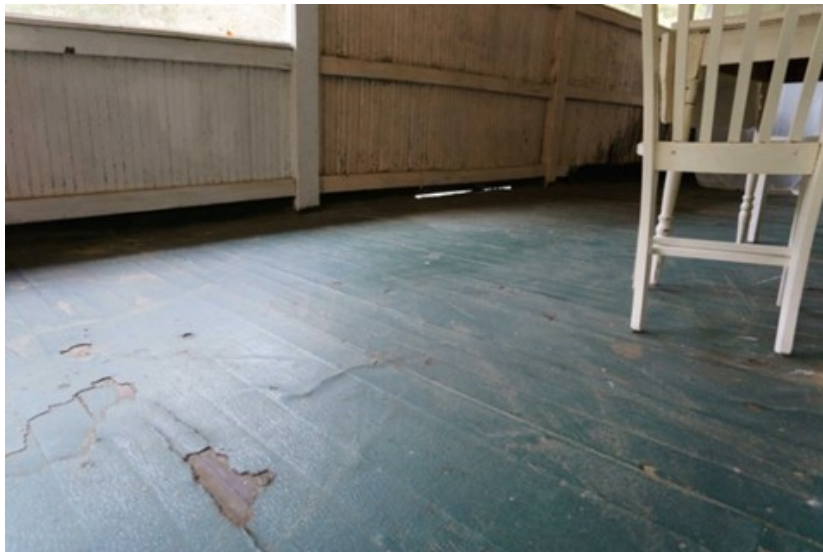
Figure 126: Room 206 facing west.
